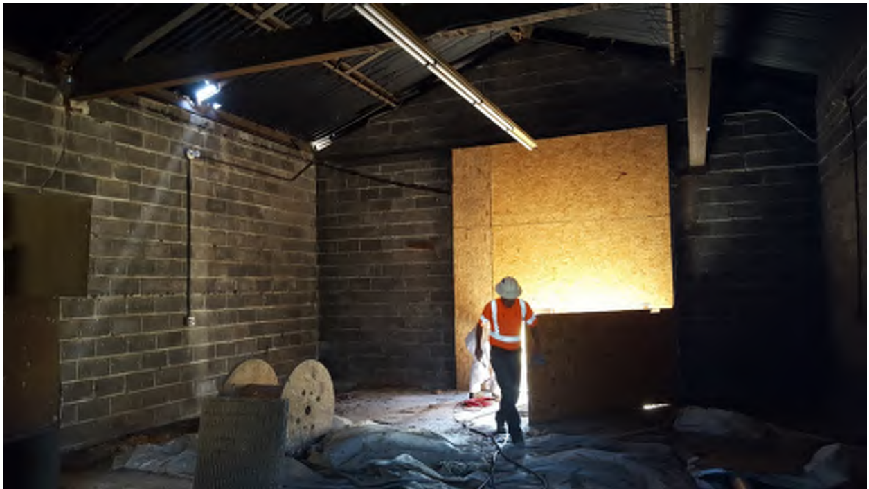
Building interior, looking south
