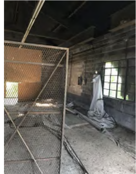
Photo 2 Building 8 interior, looking south
