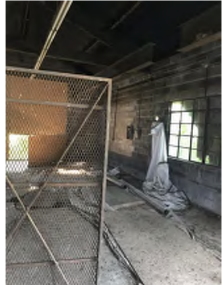
Photo 2 Building 8 interior, looking south
