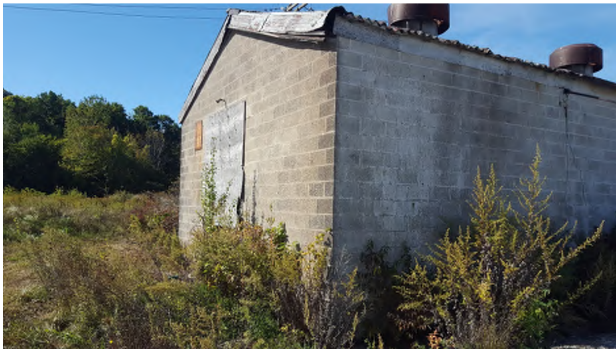
Southeast corner of Building #8, looking northwest.
