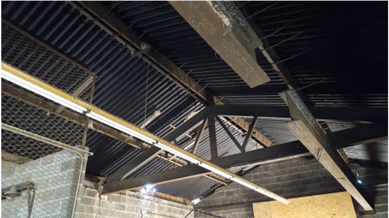
Building ceiling, looking southeast
