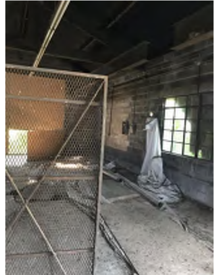
Photo 2 Building 8 interior, looking south
