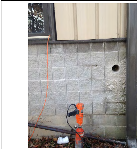
Photo No: 5 Description: Hole through exterior wall for system installation
