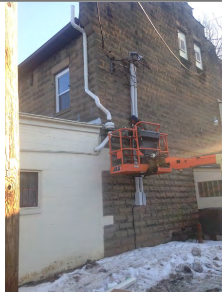
Photo No: 12 Description: System B installation in Building 3
