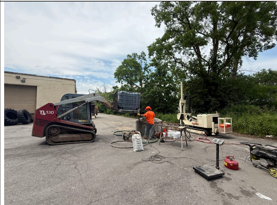
Photo 2: TREC Environmental mixing solution for IP-4 in the vicinity of MW-35M.
