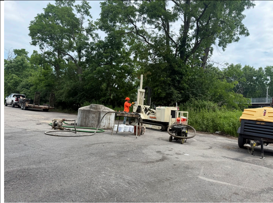
Photo 1: View of TREC Environmental setting up equipment to start injection point 3 (IP-3) in the vicinity of MW-35M.
