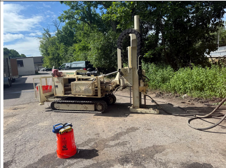
Photo 2: View of TREC Environmental injecting fluids at IP-2 in the vicinity of MW-35M.
