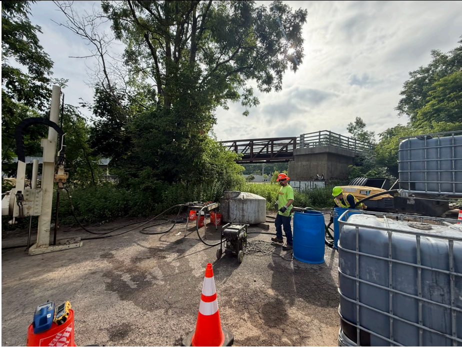
Photo 1: View of TREC Environmental injecting fluids at 35M-IP-2 in the vicinity of monitoring well MW-35M.
