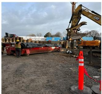
Excavating dry, clean soil from the eastern portion of the Study Area. All soil went into a dump truck and transported to the local approved landfill facility, Full roll-off dumpster, lined & covered with tarping in the process of being loaded onto a truck. All soil rolloffs staged pending PCB results.
