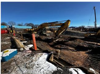
Excavating soil from the eastern portion of the Study Area. All soil went into a roll-off and was placed at the staging area pending composite sample PCB analytical results.
