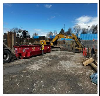
Excavating soil from then northern portion of the Study Area. All soil went into a lined roll-off and was placed at the staging area pending composite sample PCB analytical results.
