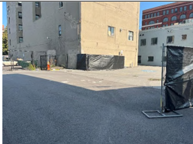
Fencing unlatched for garbage truck
