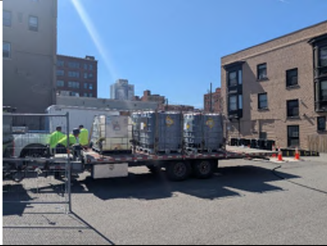
Delivery of four permanganate mixed totes.
