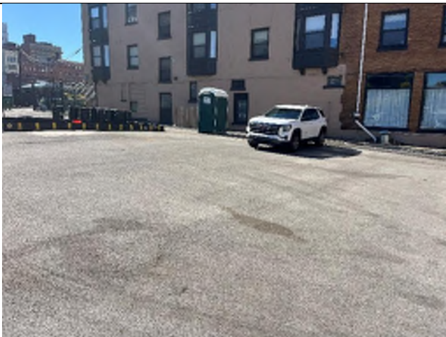
Area at the end of the day.
