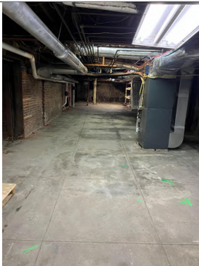
Basement area clear of injection material.
