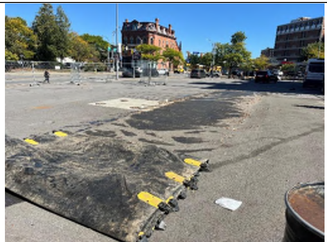
Area at the end of the day.
