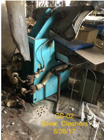
CS-02: Concrete Slab Sample Location
