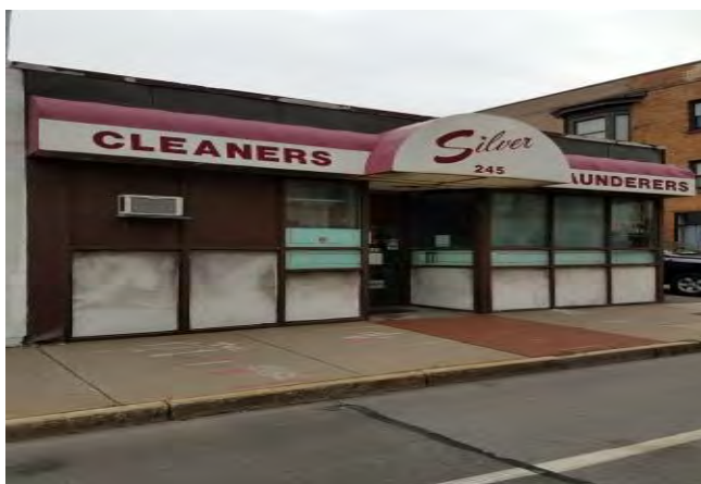
View of the Front of the Building
