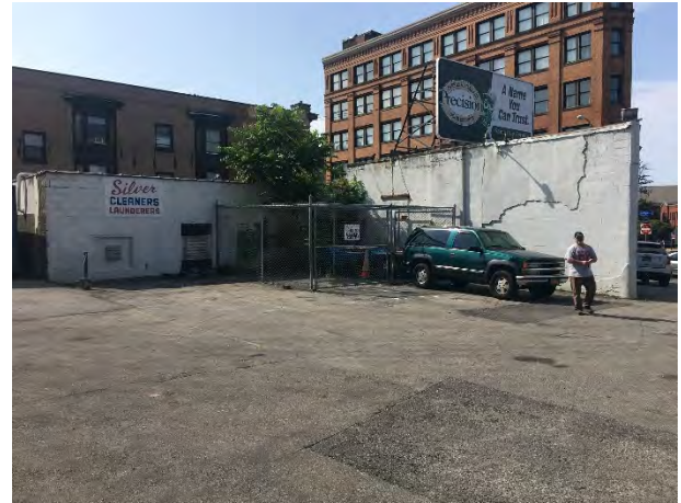
View of Rear Building Exterior- Facing Northwest
