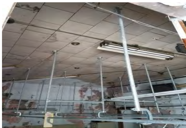
HA-9: 1' x 1' Mechanically Adhered Ceiling Tile
