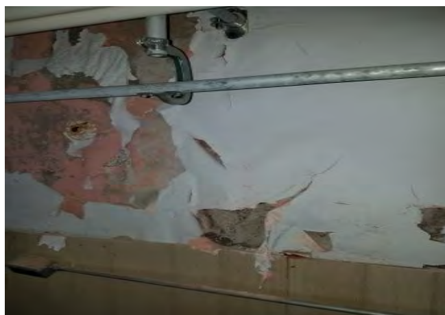
HA-11: Top Coat Plaster; HA-12: Base Coat Plaster
