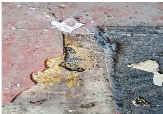
HA-1: 12" x 12" Orange Mottled Floor Tile; HA-2: Yellow Mastic from HA-1
