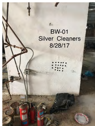
BW-01: Brick Wall Sample Location
