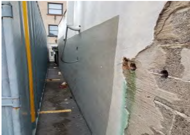
HA-33: Exterior Top-Coat Plaster; HA-34: Exterior Base-Coat Plaster
