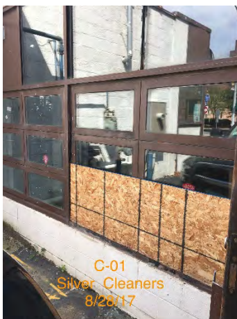
C-01: Caulk/Glazing Sample Location- Building Exterior Adjacent to Andrews St Parking Lot
