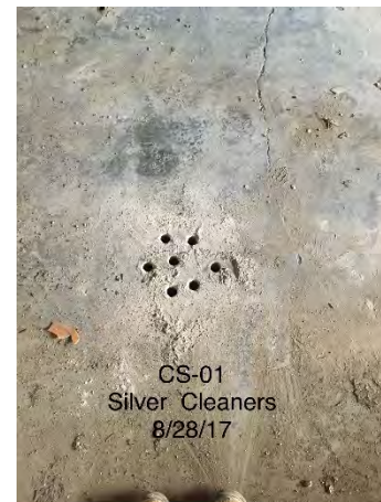
CS-01: Concrete Slab Sample Location
