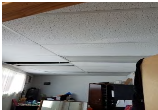
HA-10: 2' x 4' Suspended Fissured Ceiling Tile
