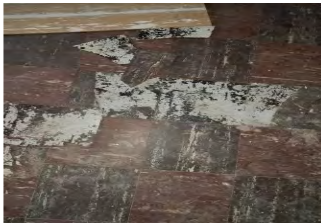
HA-5: 9" x 9" Black with White Streaks Floor Tile; HA-6: 9" x 9" Brown with White Streaks Floor Tile; HA-7: Black Mastic from HA-5 and HA-6
