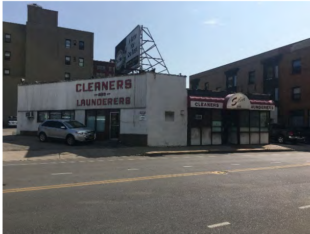
View of Building Exterior- Facing South
