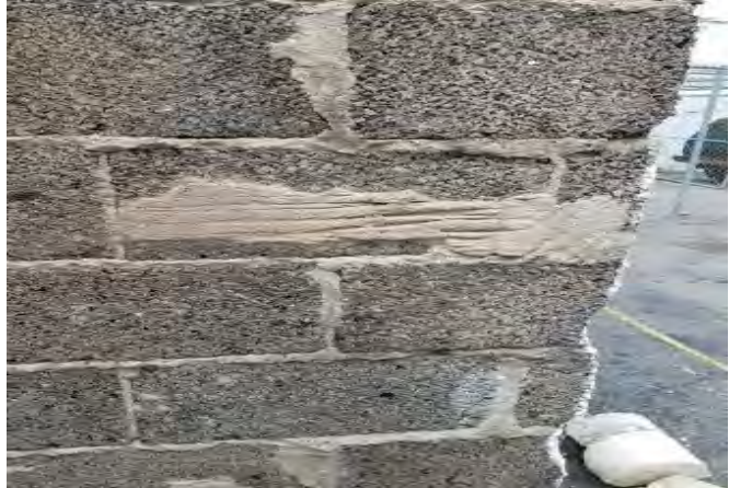
HA-35: Older Concrete Block Mortar
