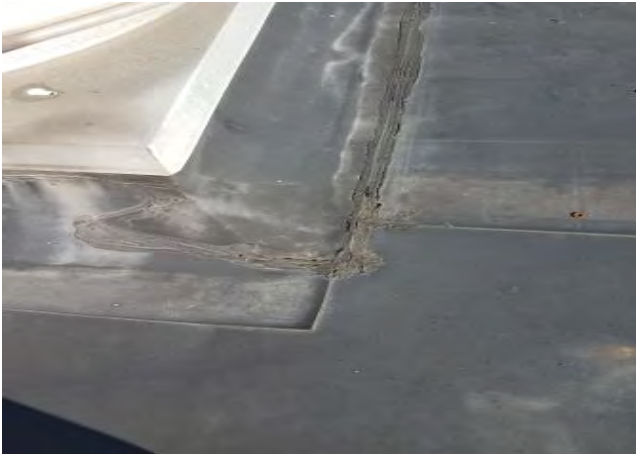
HA-48: Black Repair/Seam Caulk
