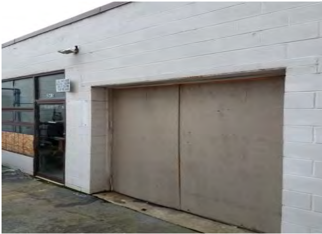
HA-31: Newer Concrete Block Mortar
