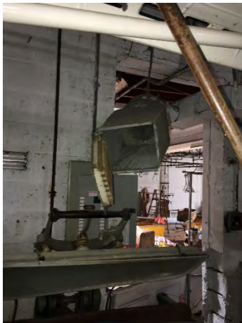
D-01: Dust Sample Location- Air Duct
