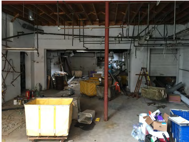
General Site Conditions- Western Portion Facing South
