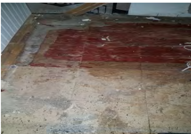
HA-17: 9" x 9" Red with White Streaks Floor Tile; HA-18: 9" x 9" White with Brown Specks Floor Tile; HA-19: Black Mastic from HA-17 and HA-18
