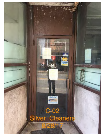
C-02: Caulk/Glazing Sample Location- Building Exterior at Andrews St Entrance
