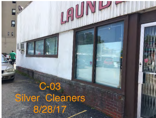
C-03: Caulk/Glazing Sample Location- Building Exterior
