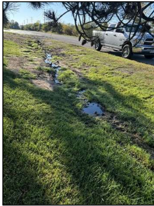
Photo 7: Example of Surfacing that occurred overnight after injection of product into eastern most PRB.
