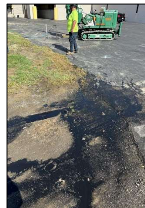
Photo 6: Surfacing occurring as a result of injection of eastern most PRB.
