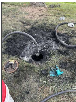
Photo 5: Active injection of monitoring well MW-3.
