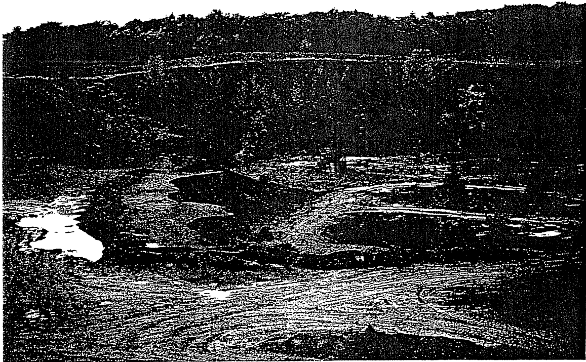
Photograph 2. View of active lower excavation bench looking north (foreground). The height of the face is approximately 20 feet. Material here consists of steeply dipping layers of sandy gravel and gravelly sand (foreset beds).
