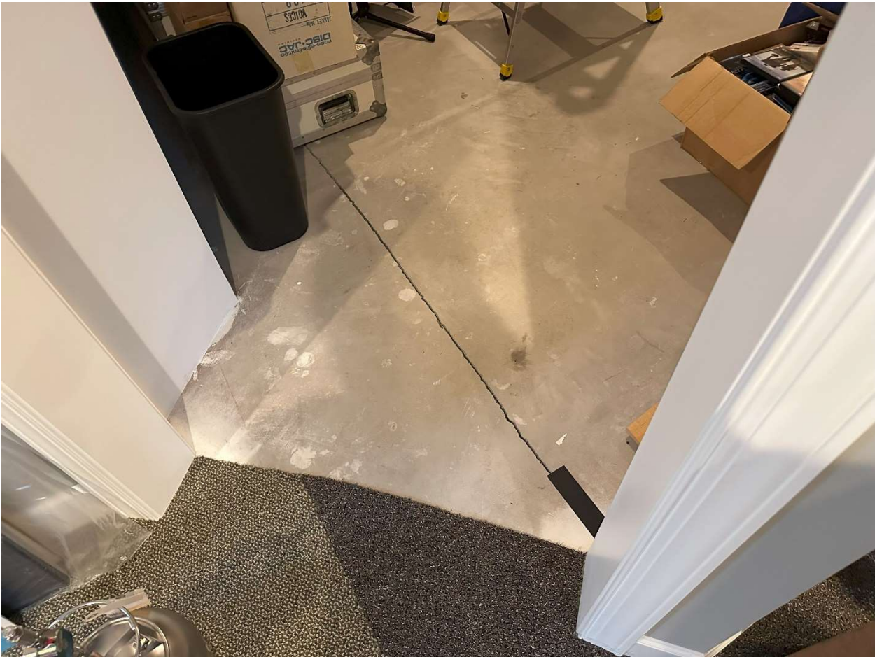
Photo 4 – Basement slab expansion joint (typ.)
