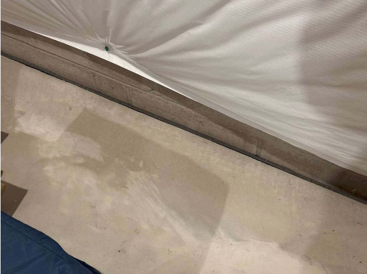
Photo 5 – Basement slab perimeter (typ.)
