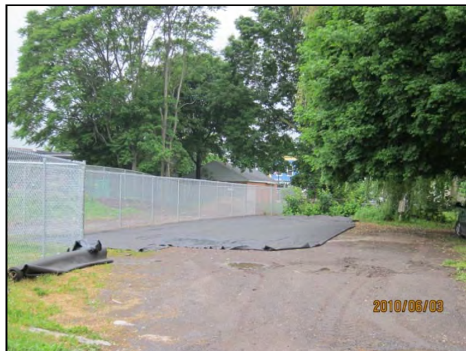
Photo #12 - June 03, 2010 Preparing surface cover area with geotextile fabric outside of the fence line; facing Southwest
