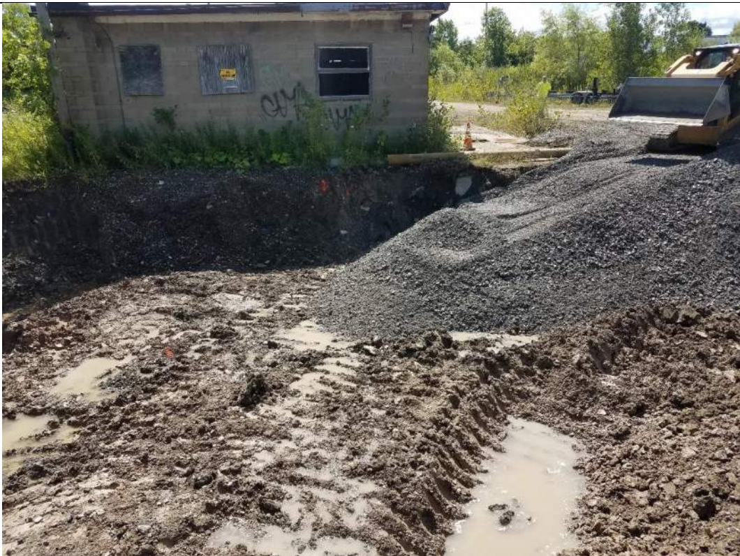
RAOC #1 being backfilled
