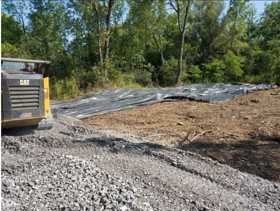
Demarcation fabric being placed in RAOC #3 central area
