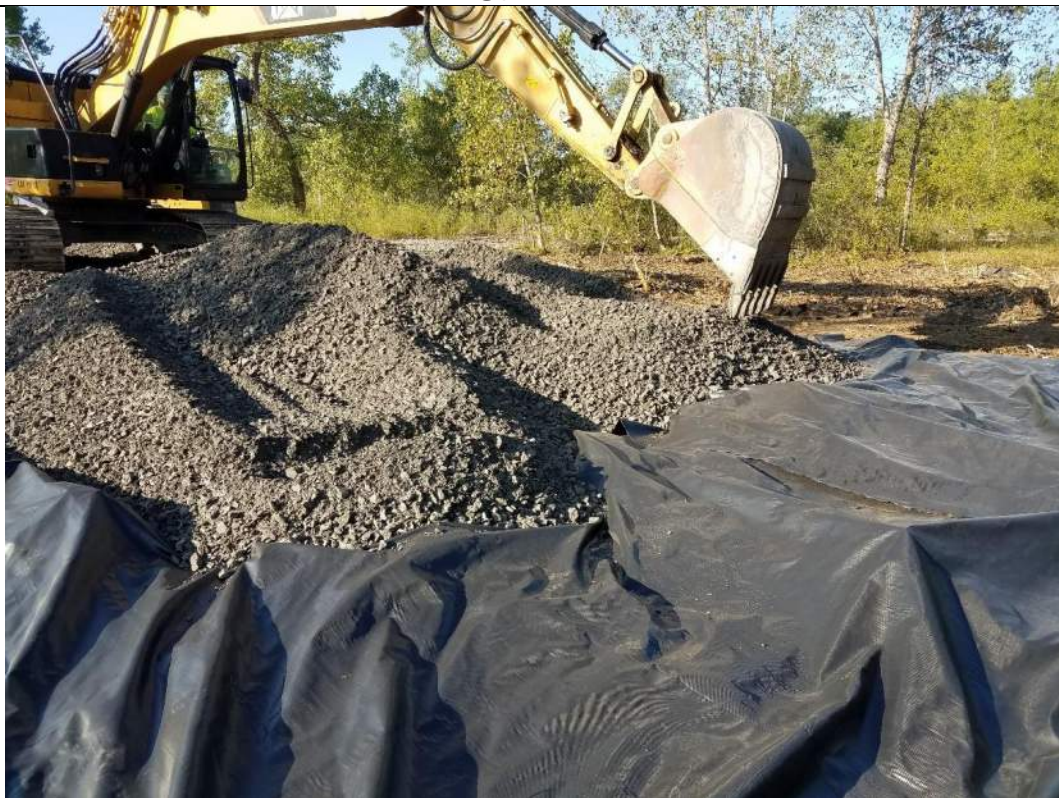
Stone being placed in RAOC #3 central area
