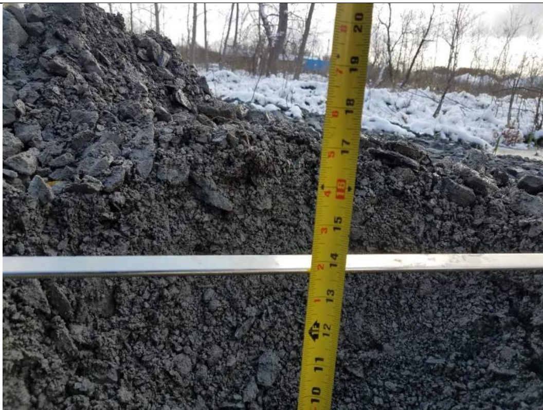
RAOC 3 El. 15 – Cover thickness at 13.75"
