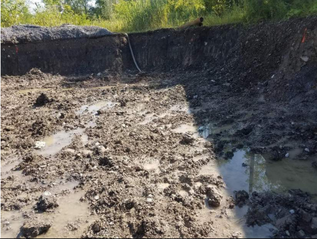
RAOC #1 excavation facing W; sidewall sample locations marked
