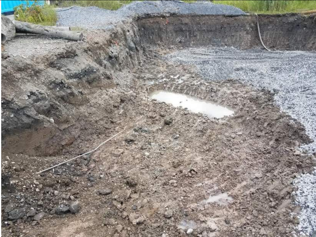
RAOC #1 being backfilled with stone
