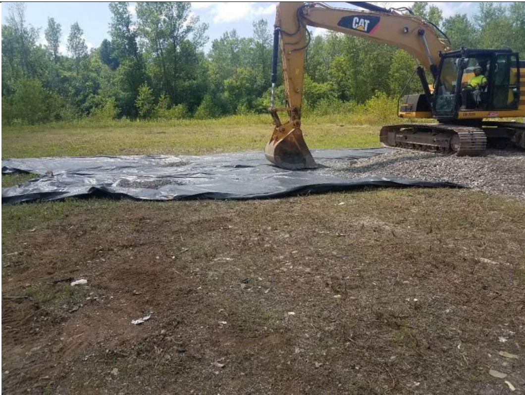
Stone being placed in RAOC #3 southern area
