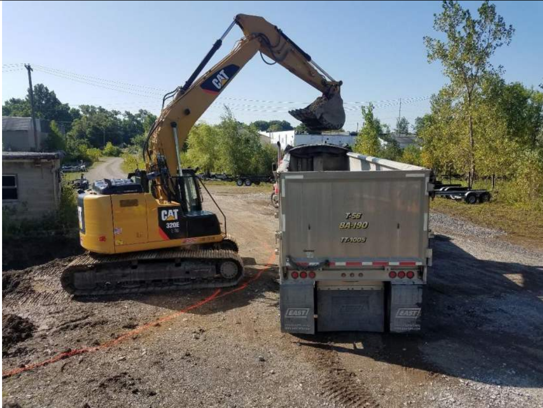
Excavated soil from RAOC #1 being direct-loaded
