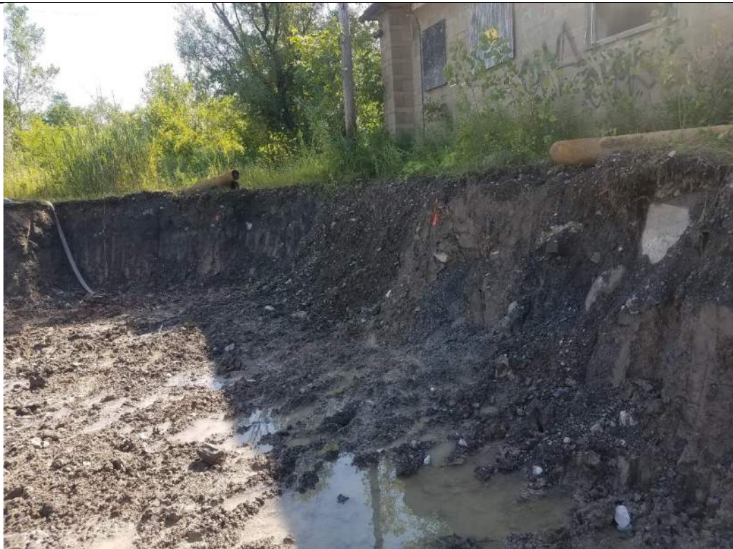
Southern sidewall of RAOC #1 along scale house; sidewall sample locations marked
