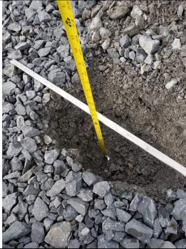
RAOC 3 El. 9 – Cover thickness measurement
