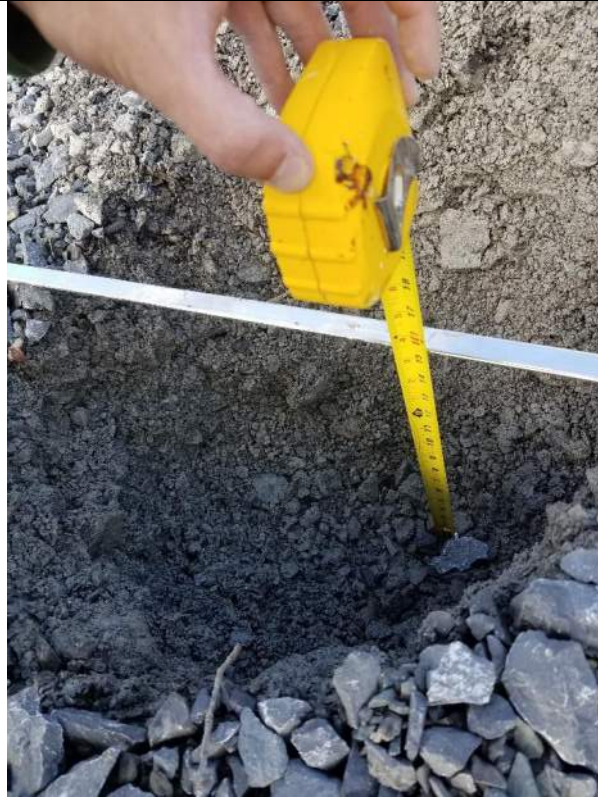
RAOC 3 El. 12 – Cover thickness measurement
