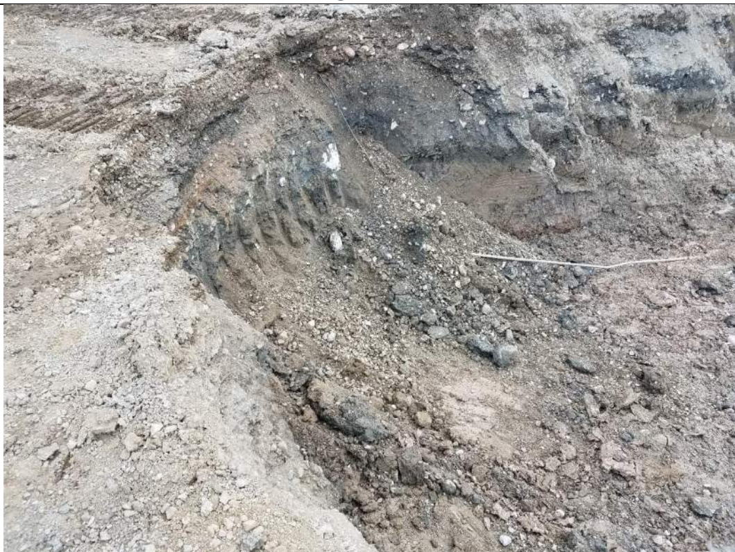
RAOC #1 northwest corner sidewall; strong petroleum odor
