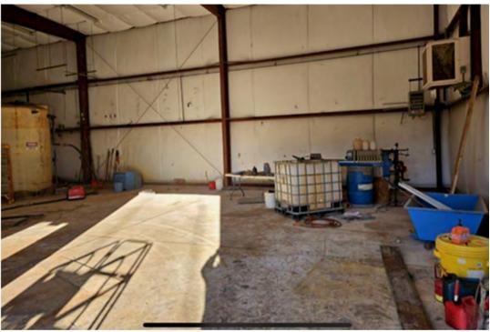
inside of former WTP with all process piping and equipment removed except for groundwater holding tank and filter press
