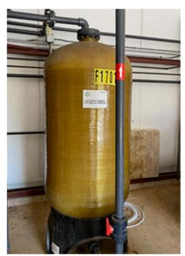
One of two carbon vessel which have been drained and carbon removed
