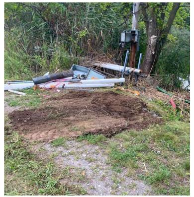
Extraction Well EW-4 prior to abandonment following grouting and removal of appurtenances and well casing.
