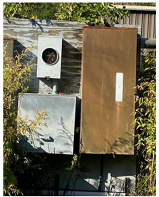
Remains of the old electrical panel with the main feed. Note that the electrical meter was removed by National Grid.
