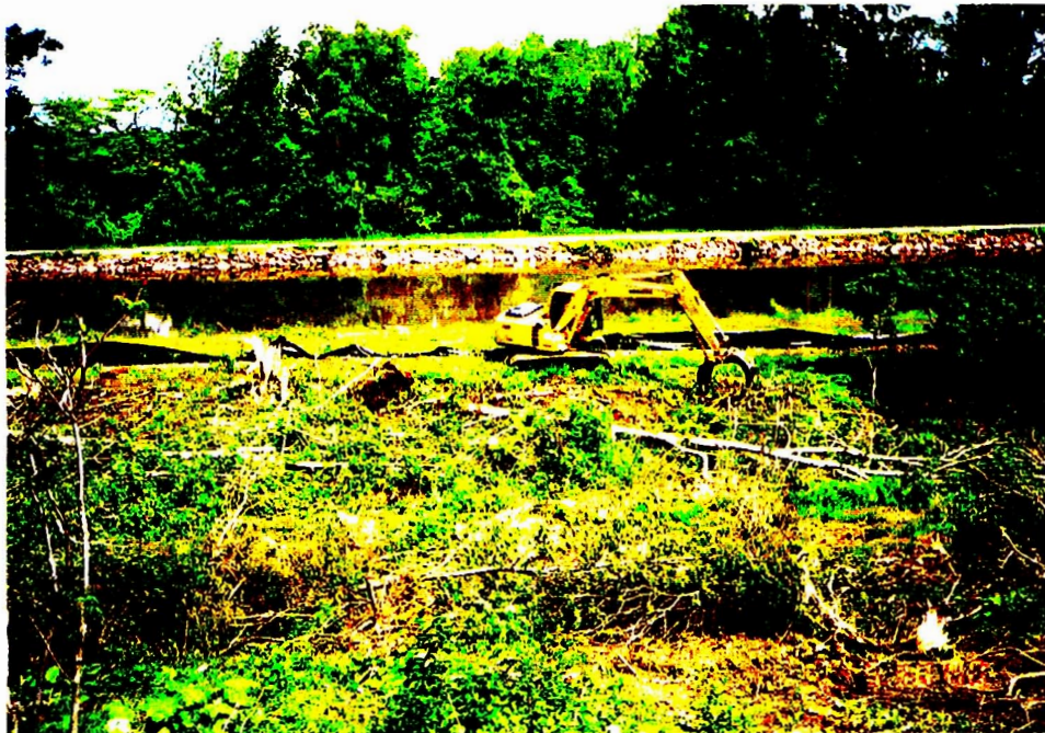
CLEARING AND GRUBBING OF TREES, SHRUBS AND BRUSH ALONG NORTH SIDE OF LANDFILL.
