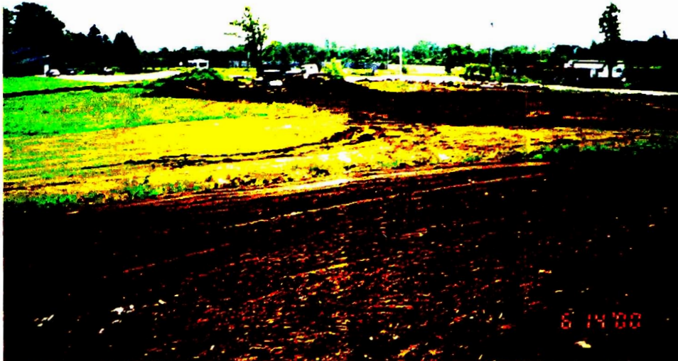
STRIPPING OF TOPSOIL FOR EXISTING SOIL RECOVERY
