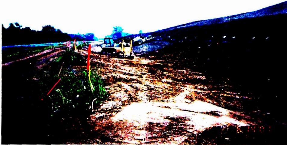
LOW PERMEABILITY CLAY PLACEMENT AND COMPACTION
