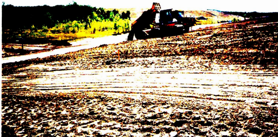
BARRIER PROTECTION MATERIAL PLACEMENT
