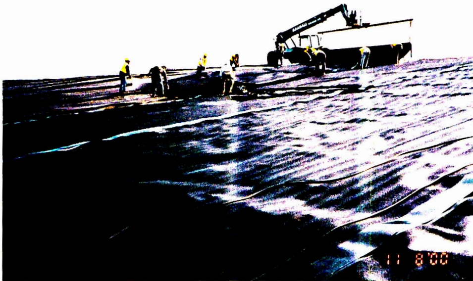
LLDPE GEOMEMBRANE DEPLOYMENT
