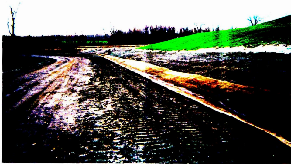
DRAINAGE CONTROL STRUCTURE-JUTE MESH WITHIN WEST END DRAINAGE SWALE
