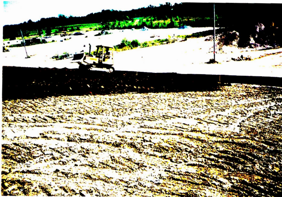
TRACKING IN TOPSOIL
