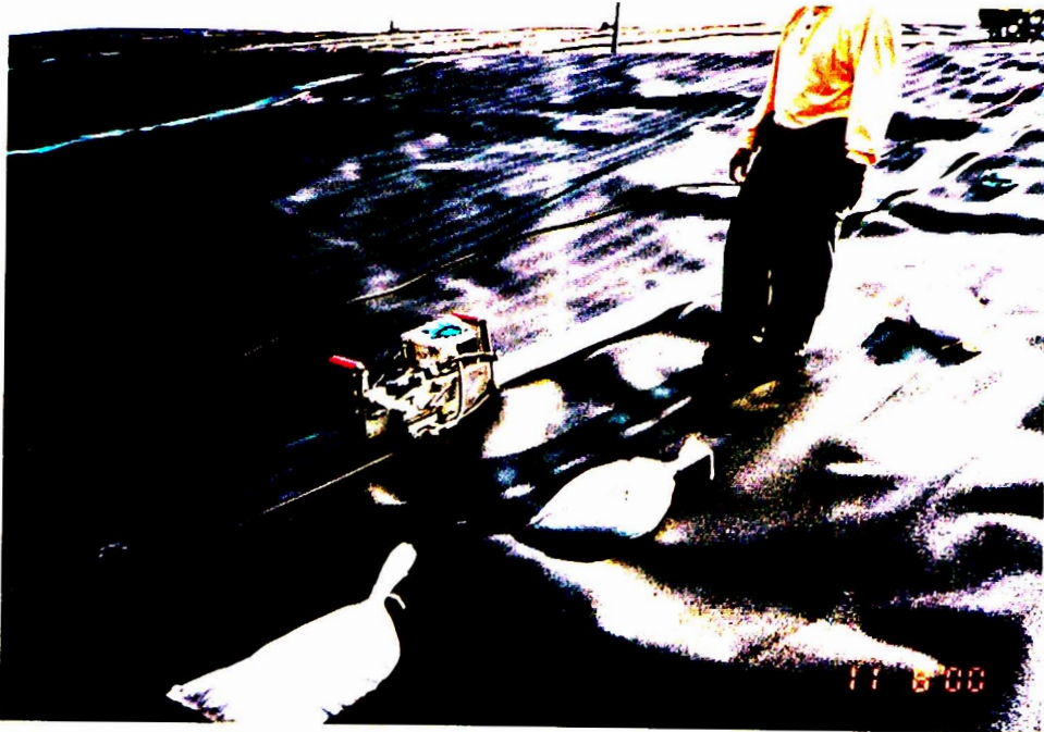
FUSION WELD OF LLDPE GEOMEMBRANE
