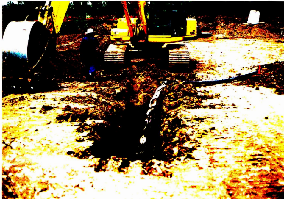
INITIAL EXCAVATION AND INSTALLATION OF SLURRY MIXTURE FOR SOIL-BENTONITE BARRIER WALL
