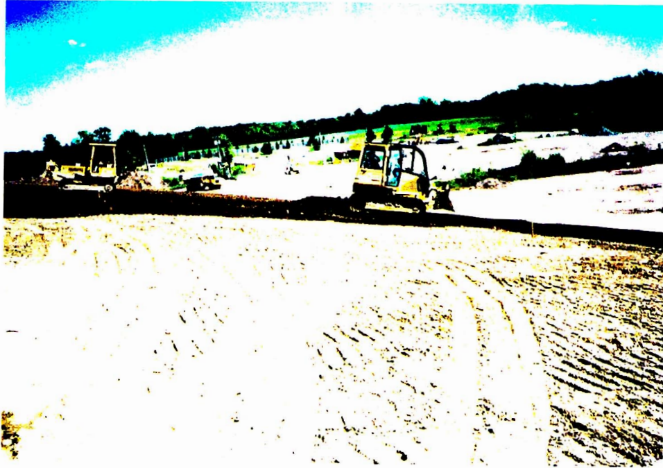
TOPSOIL PLACEMENT
