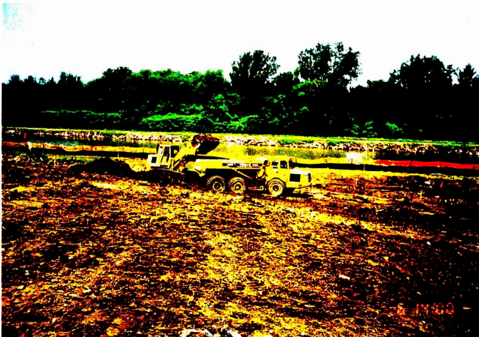
REMOVAL OF COVERSOIL FOR EXISTING SOIL RECOVERY
