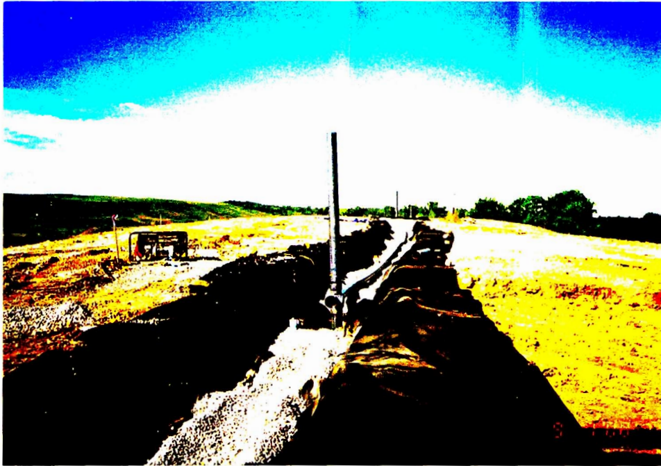
GAS VENT RISER AS PART OF GAS VENTING SYSTEM
