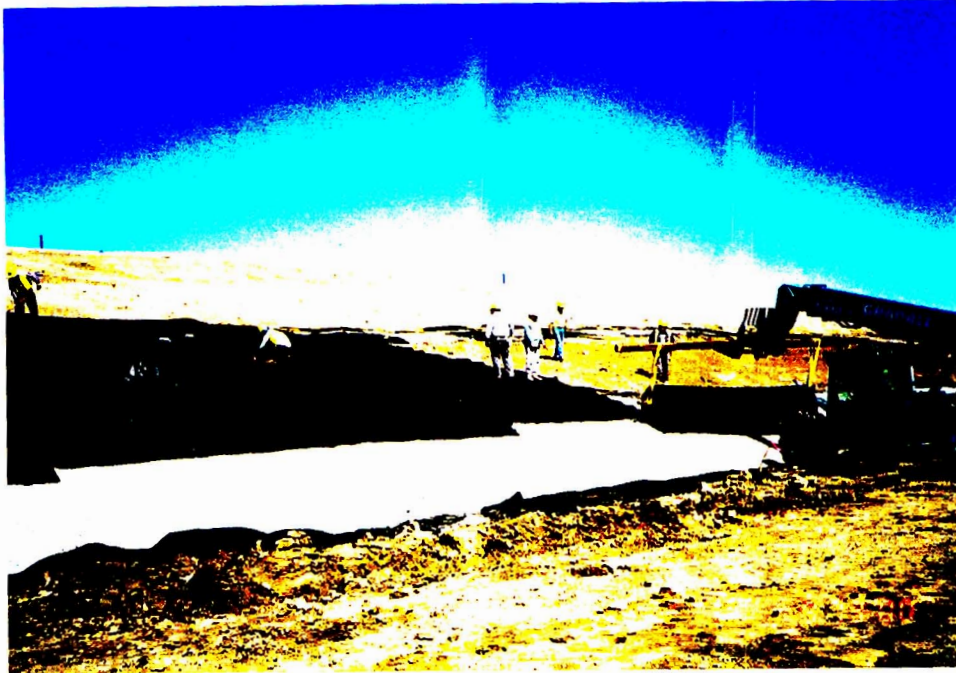
GAS VENTING/LEACHATE COLLECTION SYSTEM GEOCOMPOSITE DEPLOYMENT
