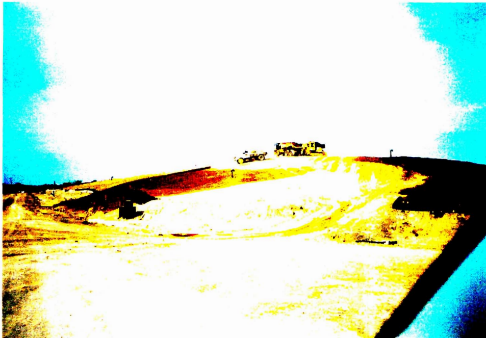
HYDRATING OF THE SUBGRADE PRIOR TO TOPSOIL PLACEMENT
