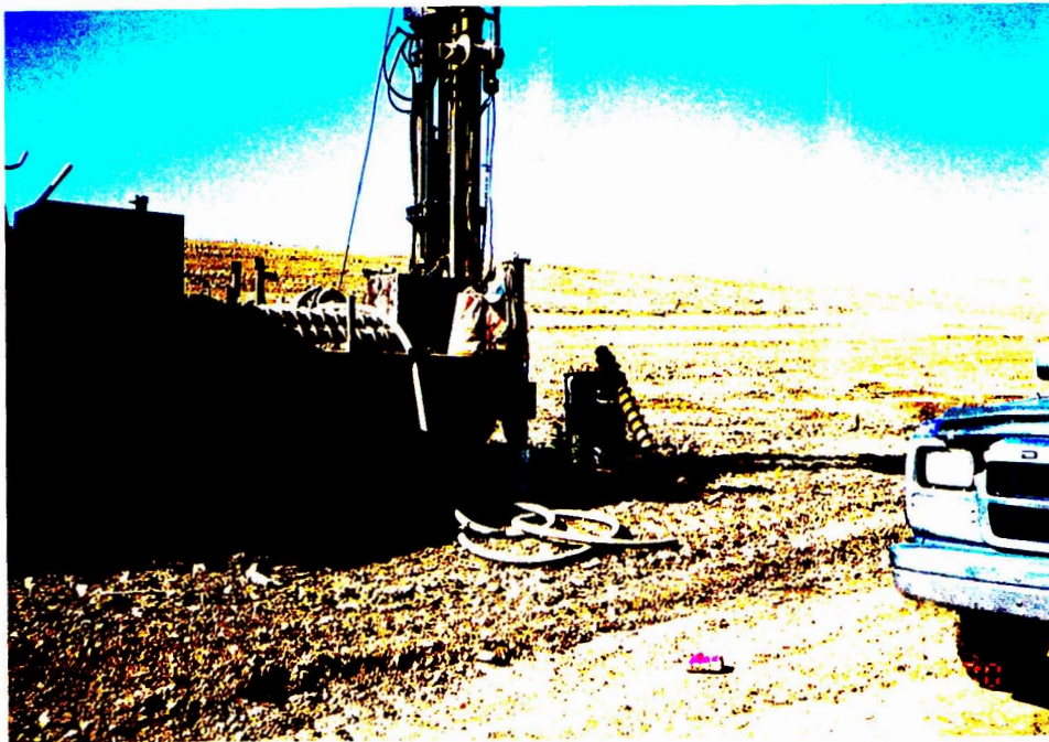
DECOMMISSIONING OF EXISTING MONITORING WELL PERFORMED BY SJB DRILLING SERVICES
