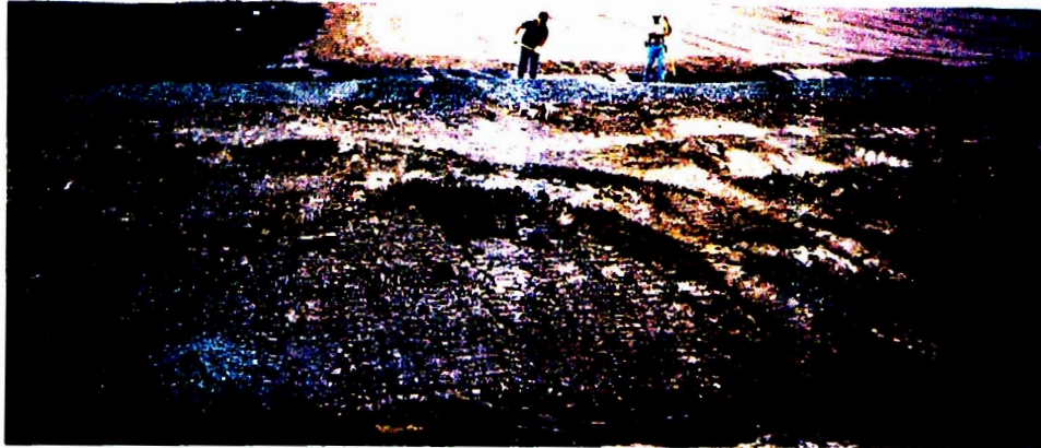
DRAINAGE STONE PLACEMENT FOR WEEP DRAIN CONSTRUCTION
