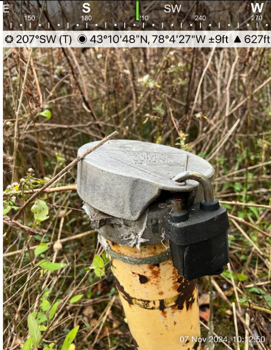
Photo 1: MW-15D broken casing cap and previously cut lock. Cap is unsecured, but able to close flush.
