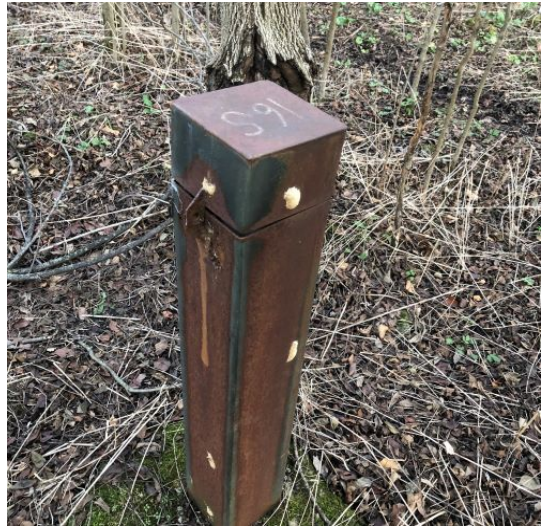
Photo 6: Looking northwest at monitoring well MW-16S
