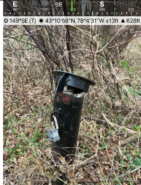
Photo 2: MW-19S unable to close cap due to riser and J-plug sitting too high.
