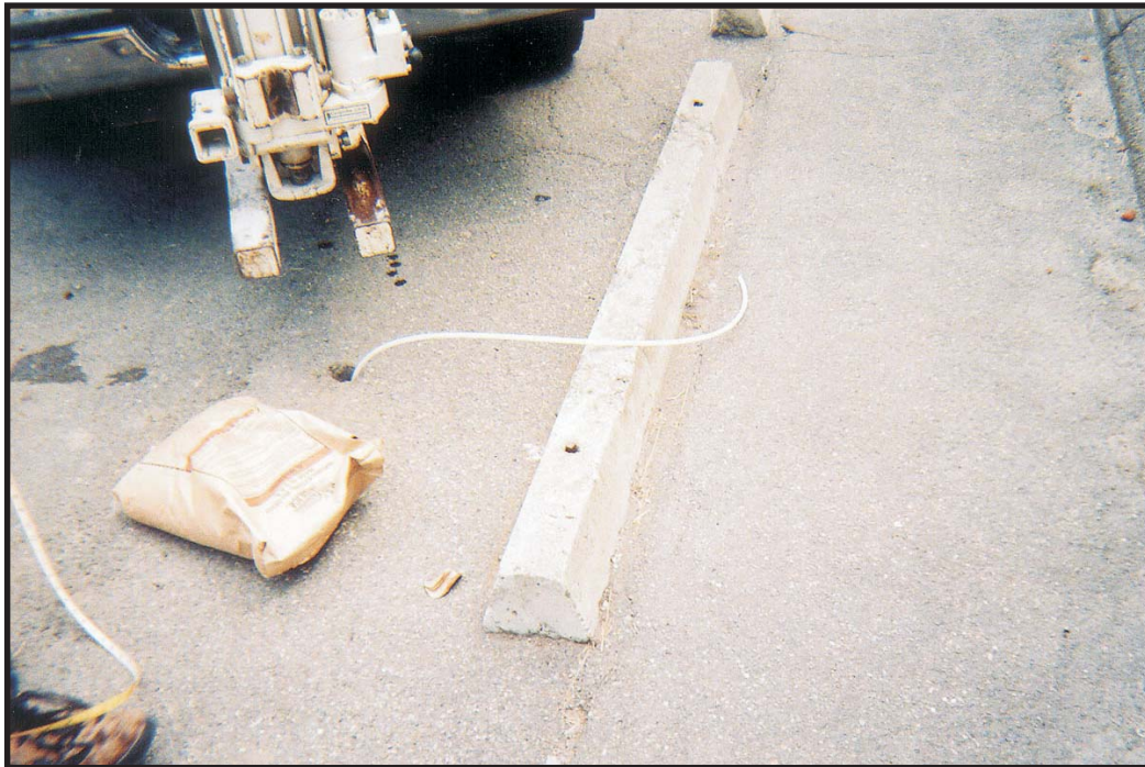
Photo 3: Photograph of installed soil gas implant prior to installation of bentonite seal and protective casing.
