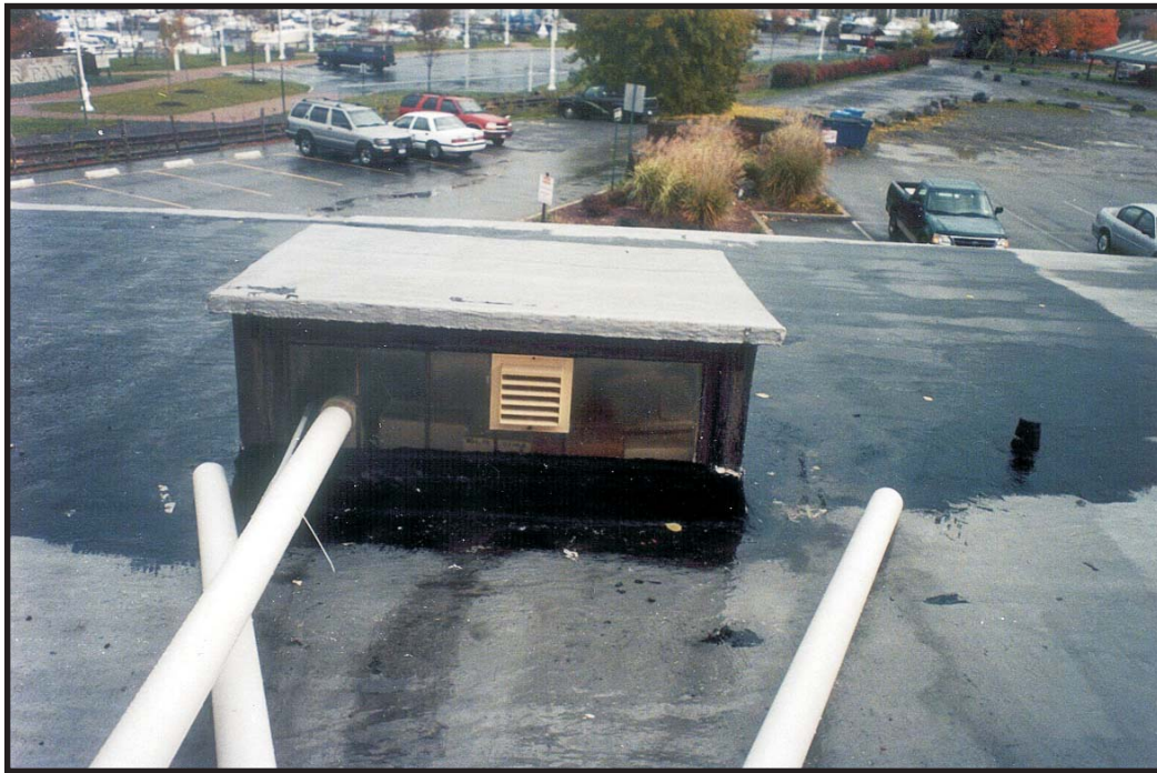
Suction pipe and electrical penetration of dormer.
