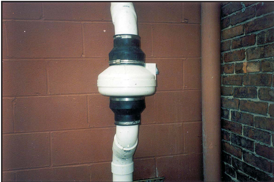
Photography of fan mounted on side of building.
