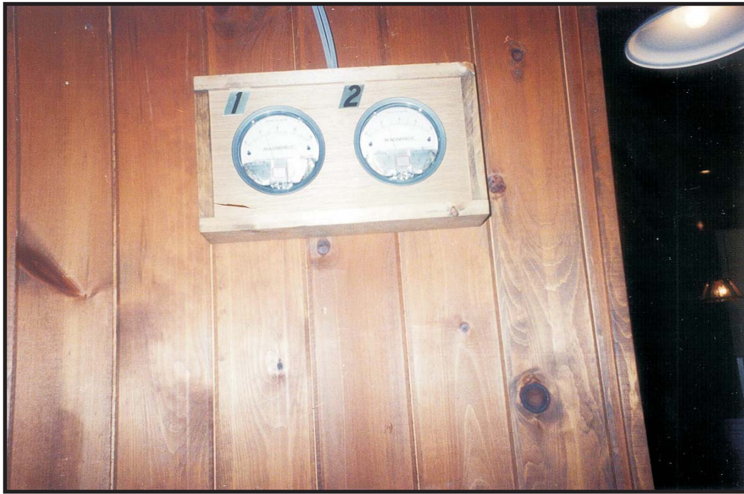
Photograph of Magnehelic gauges indicating suction at both points.
