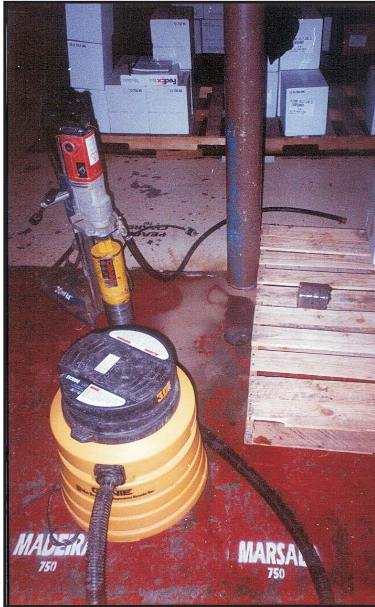
Photograph of coring slab at suction point #1.
