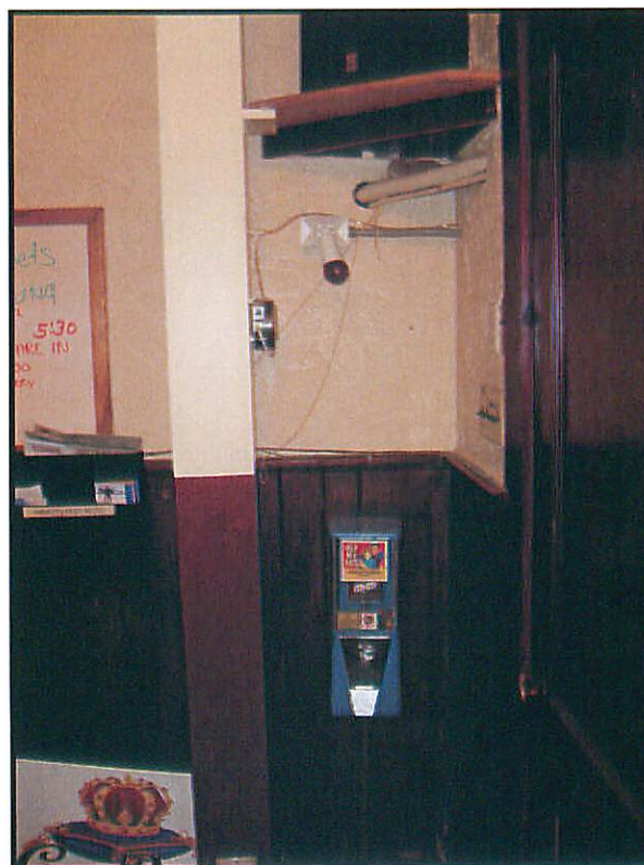
Photo 4: VFW suction point #3, magnahelic, and indicator light.
