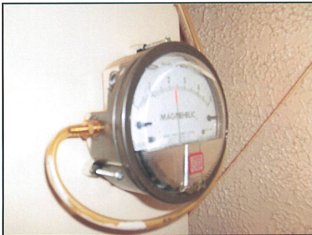
Photo 3: VFW suction point #3 magnahelic.
