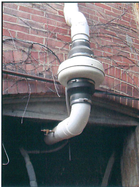
Photo 5: VFW SSD system fan.
