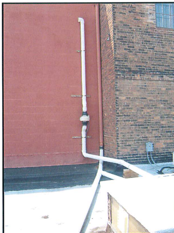
Photo 10: Seneca Market SSD system fan and vent stack.
