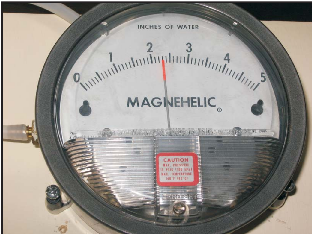
Photo 6: VFW suction point #1 magnehelic reading after installation of new connection hose.
