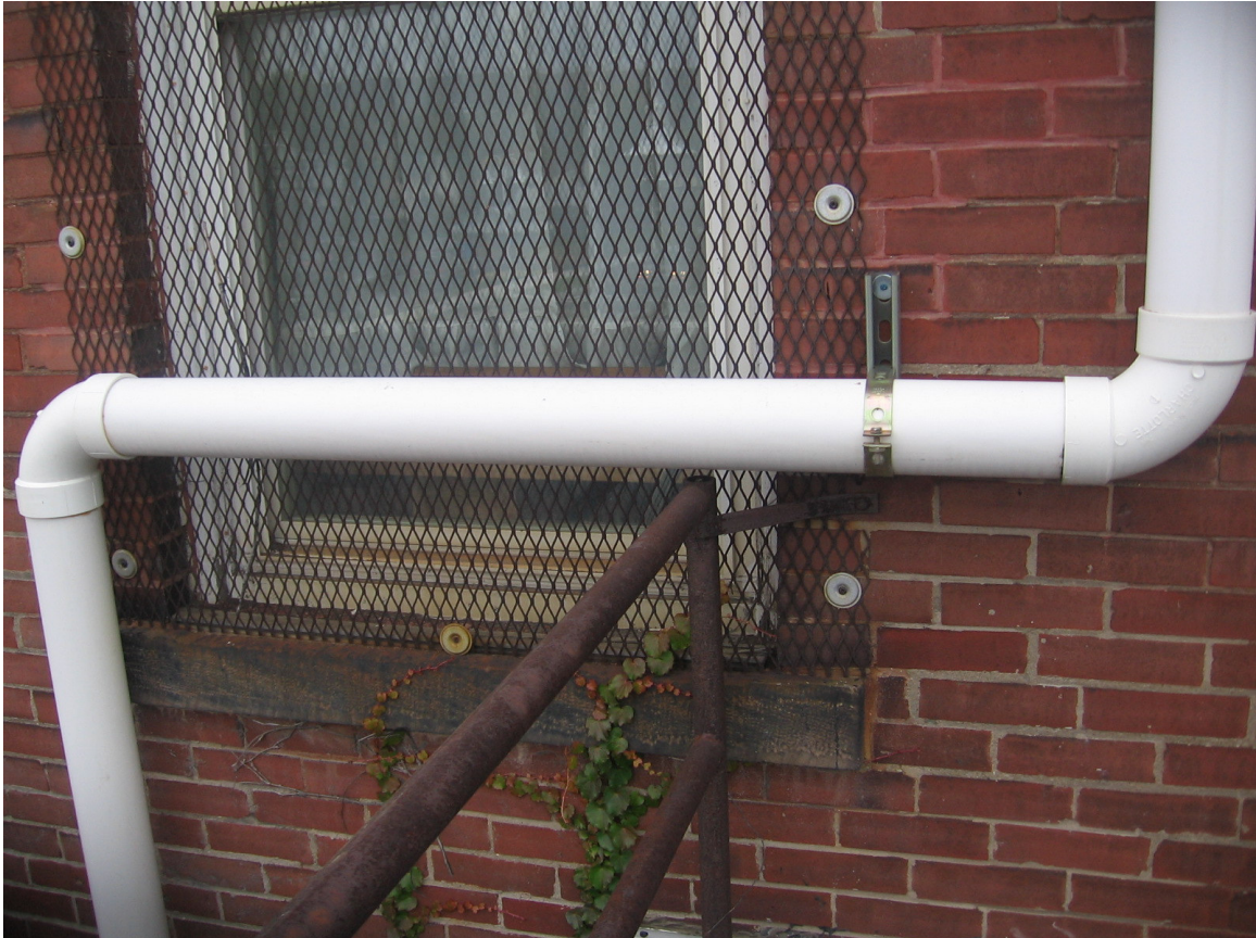
7. Close up of vent pipe and fasteners.
