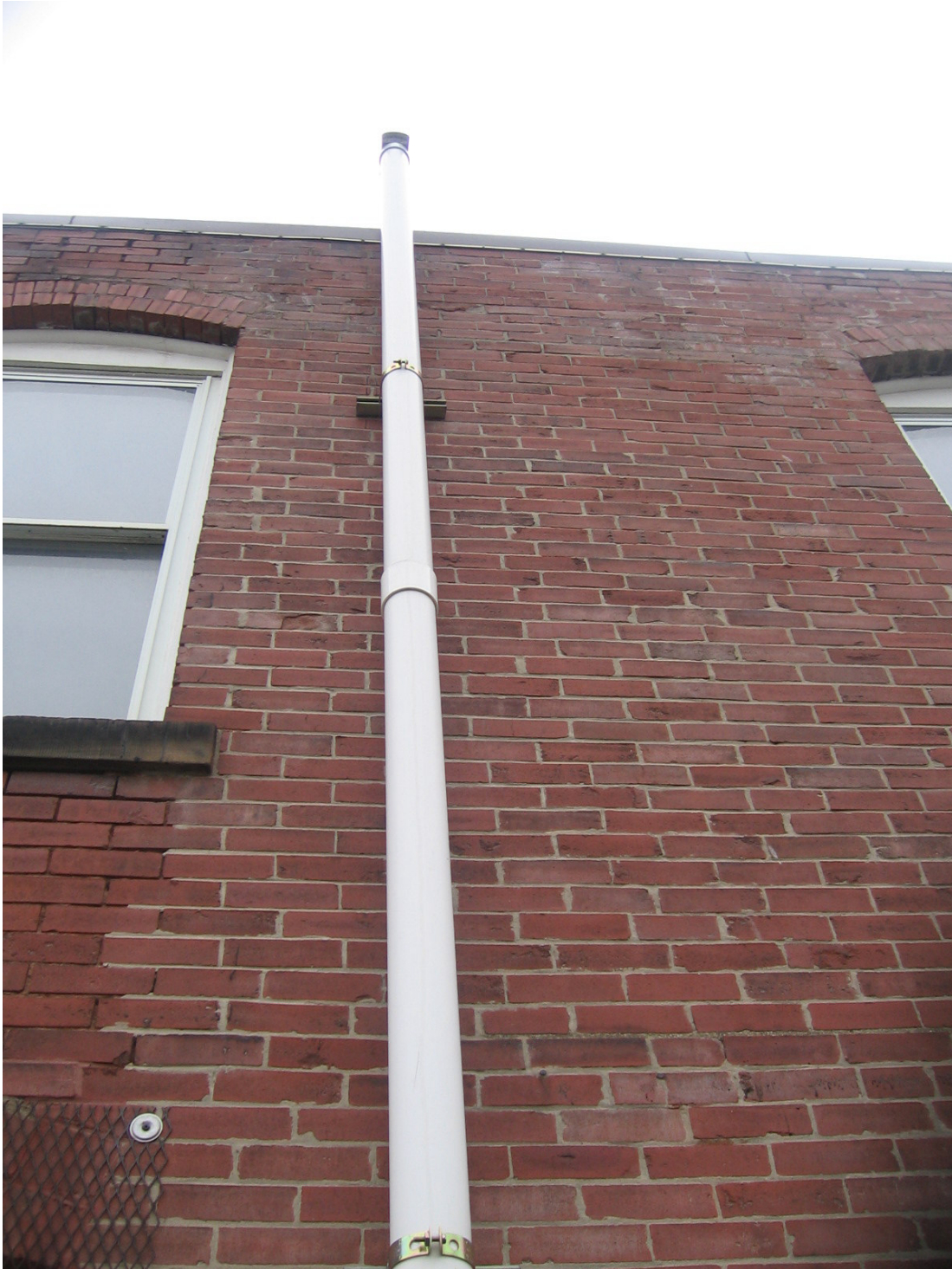
8. Close up of top of vent pipe, and fasteners.
