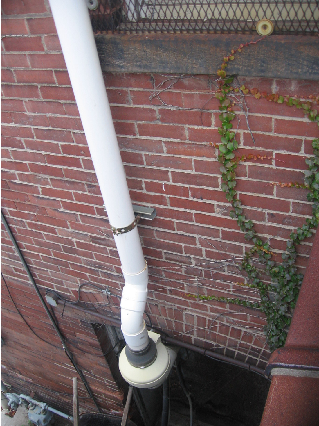
6. Close up of suction fan, vent pipe and fasteners.
