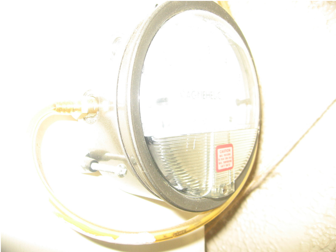
4. Photograph of suction point #3 magnehelic gauge.
