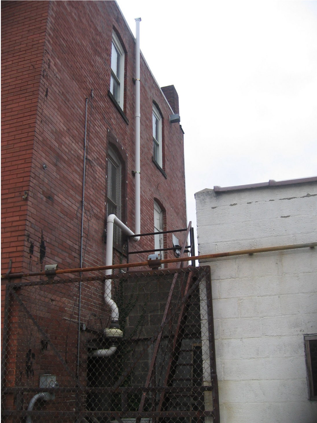
5. Photograph of suction fan and vent pipe. All fasteners re holding vent pipe securely to the wall..
