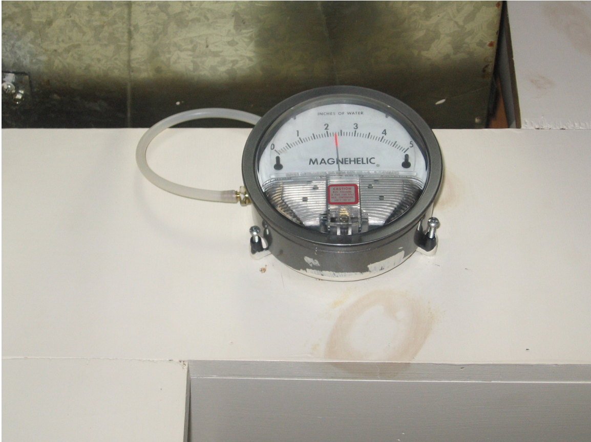
2. Photograph of suction point #1 magnehelic gauge.
