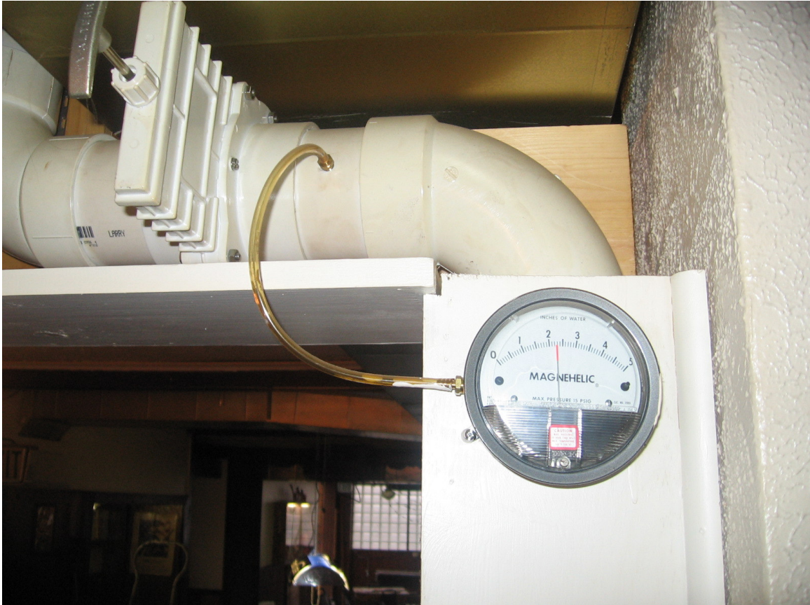
3. Photograph of suction point #2 magnehelic gauge.
