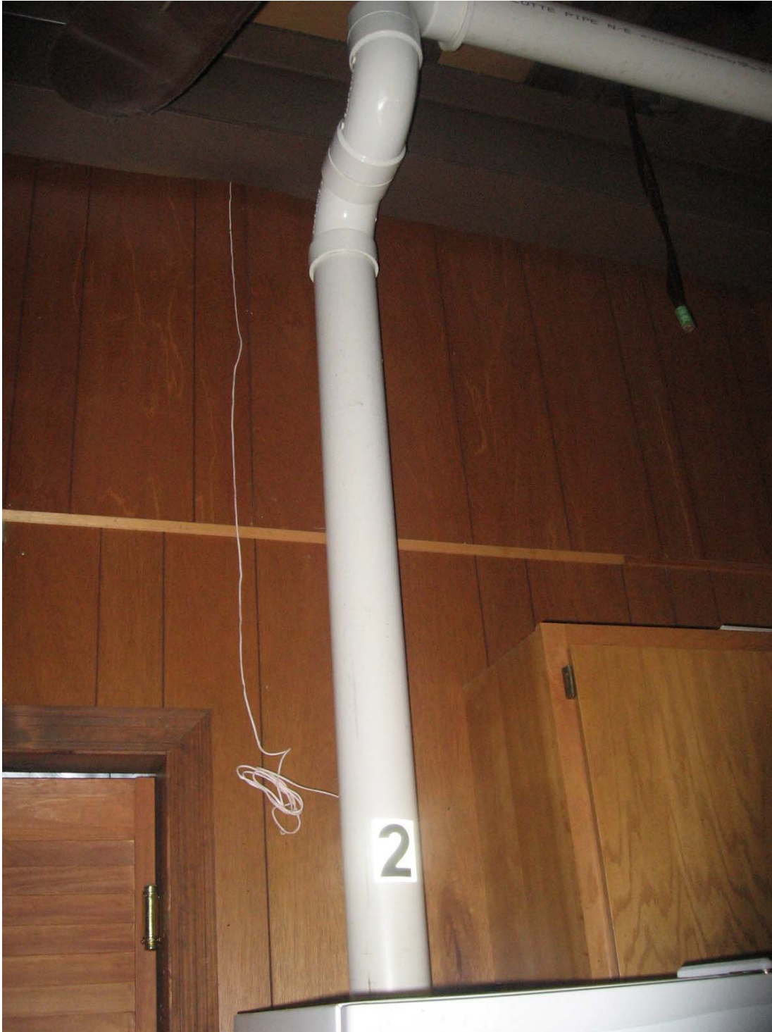
4. Photograph of suction point #2. All PVC welds are in good shape.
