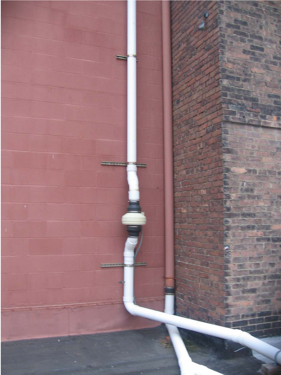
5. Photograph of suction fan and vent pipe. All fasteners are holding vent pipe securely to the wall.
