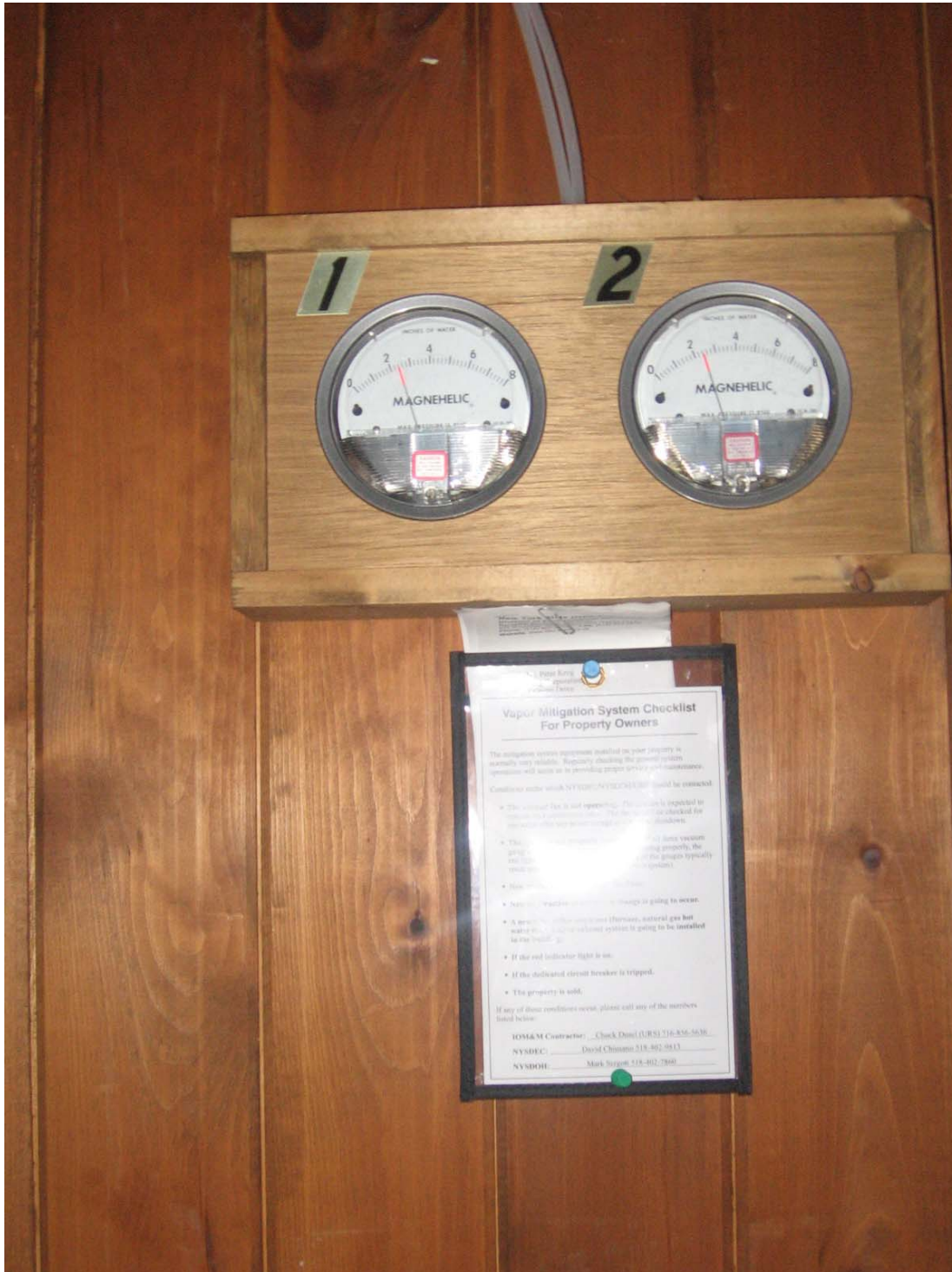
2. Photograph of magnehelic gauges and mitigation system labels
