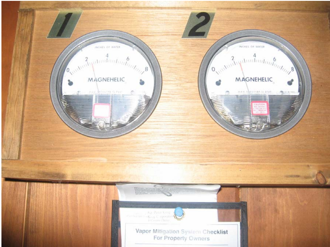
1. Close up of magnehelic gauges.
