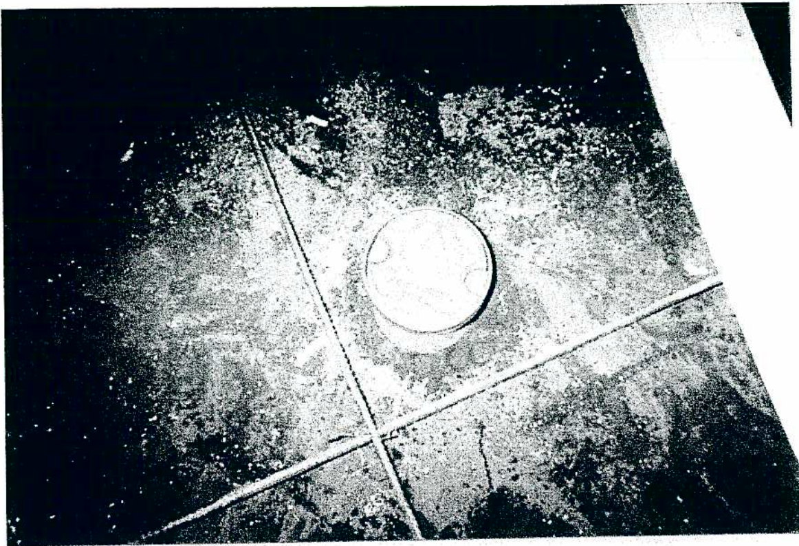
Photo 11: View of completion for newly installed sump well.
