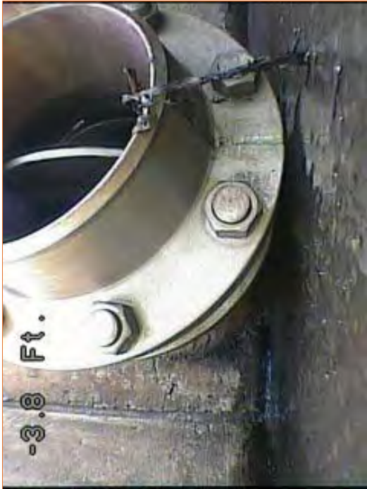
Photo 84. Outfall 010 (010-001 to 010-000): Outfall 010-000 gate valve from canal side chamber
