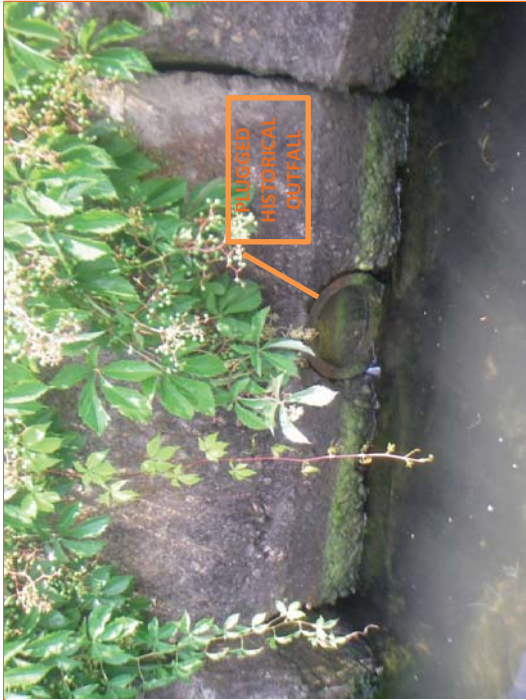
Photo 44. Abandoned 6" diameter historical outfall located between Outfalls 005 and 010. Plugged at discharge point. Seems to correspond to historical pipe No. 8.
