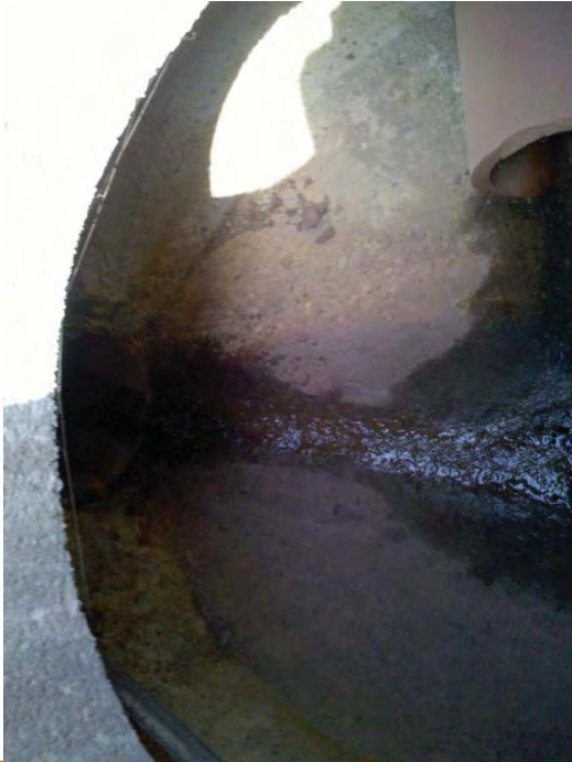
Photo 93. Outfall 001: 001-001 Manhole topside (north up). North and east pipes.
