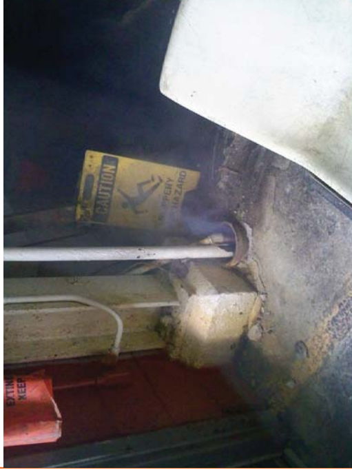
Photo 4. Outfall 001: Smoke observed at new vertical pipe between 001-001 and 001-001C
