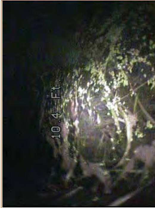
Photo 72. Outfall 005 (005-001A to 005-001): Roots and weeds at 10ft upstream of 005-001
