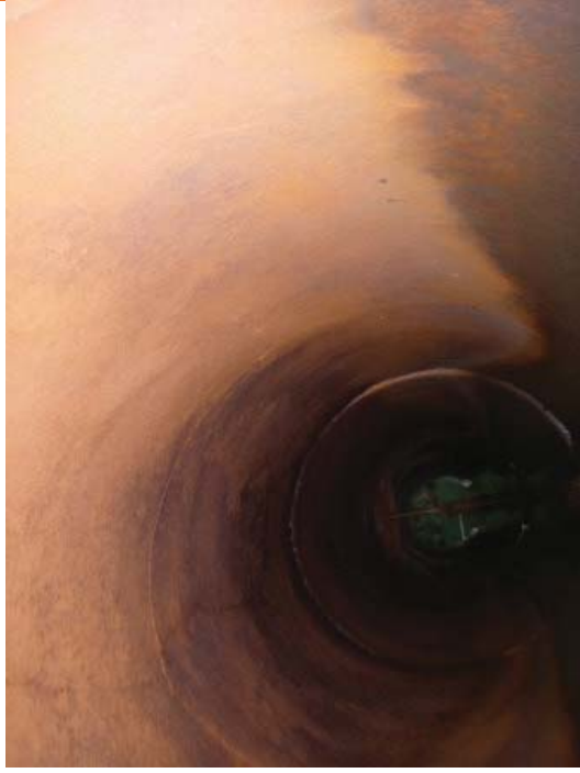
Photo 102. Outfall 004: 004-001 Pipe connections (south pipe)
