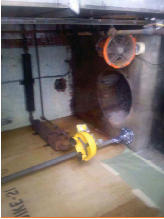
Photo 140. Former Hotwell 4A in S-6 shed outside south wall of Building 4; concrete paved with inlet piping
