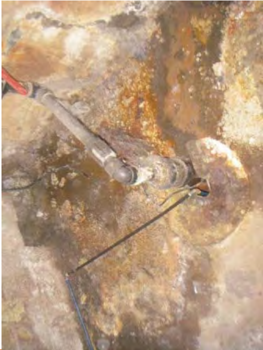
Photo 117. Building 1: 007-003 Floor drain area
