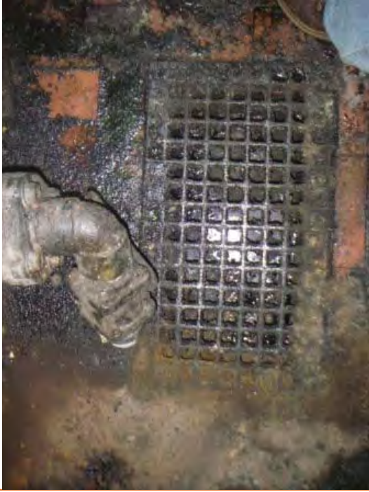
Photo 121. Building 2A: 007-008 floor drain
