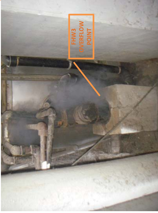
Photo 14. Outfall 005: Smoke observed at 005-001B near former Hotwell 3 overflow point
