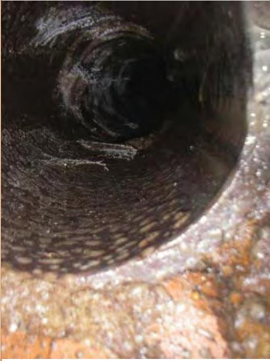
Photo 112. Sanitary sewer: 004-008 Pipe connections (west pipe)
