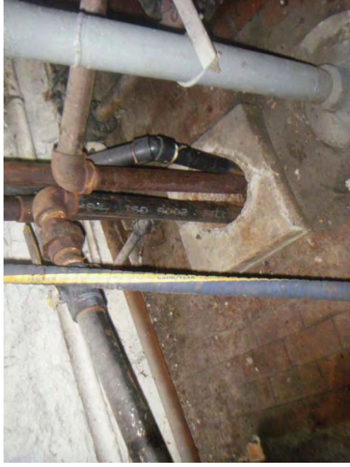
Photo 126. Building 4 floor drain near northeast wall
