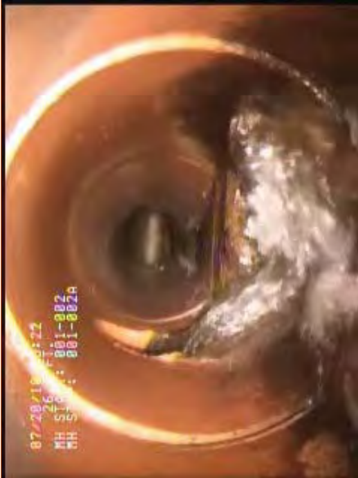
Photo 47. Outfall 001 (001-001B to 001-001): Noncontact cooling water discharged from active factory tap in Building 4 (001-001D to 001-001C)
