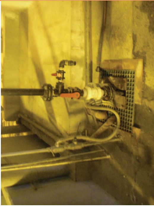
Photo 122. Building 3 floor drain near northwest wall
