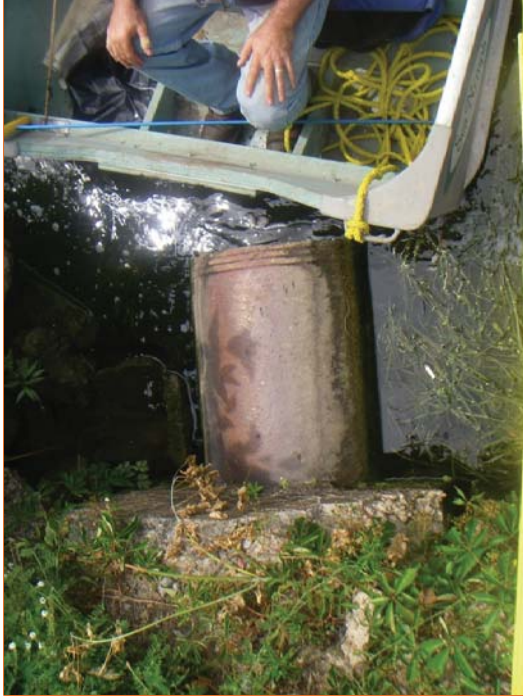
Photo 27. Outfall 005: Discharge point 005-000
