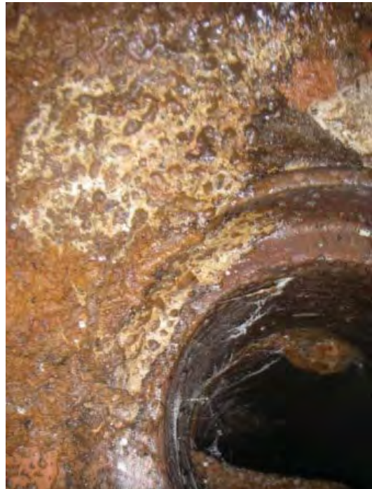
Photo 110. Building 2-A sanitary sewer: 004-008 Pipe connections (east)
