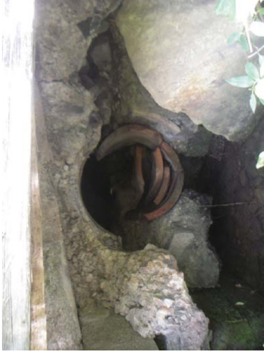
Photo 30. Outfall 006: 15" Diameter abandoned discharge point 006-000 which seems to correspond to historical pipe No. 15
