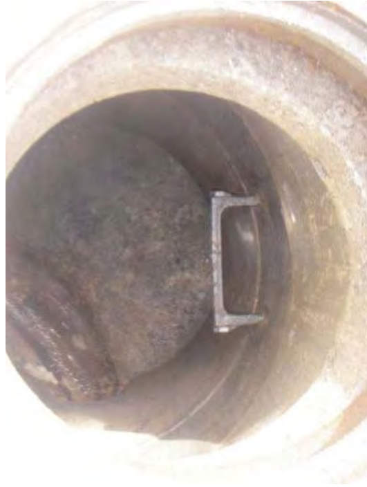
Photo 114. Outfall 007: 007-001 Manhole topside (north up)
