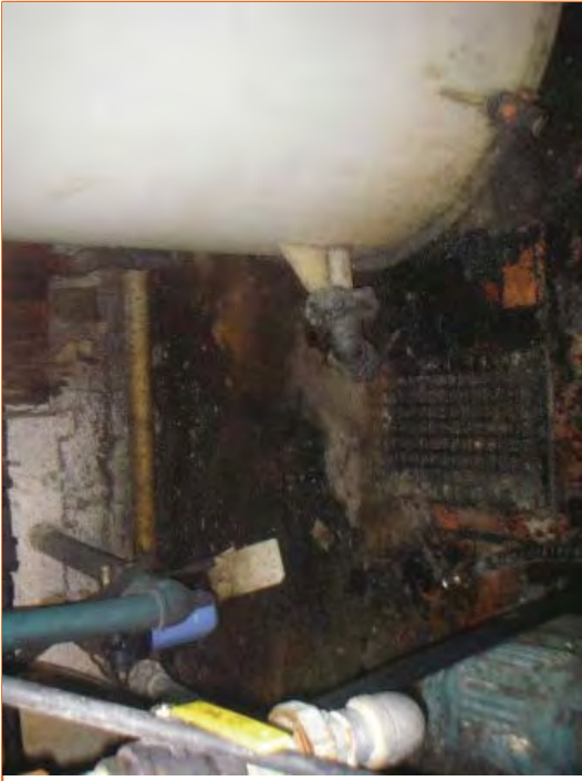
Photo 120. Building 2A : 007-008 Floor drain
