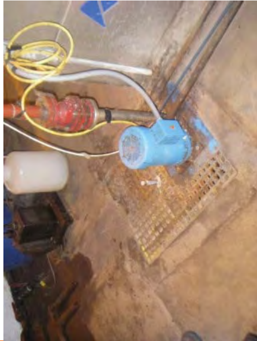
Photo 105. Building 1: 004-002 Floor drain
