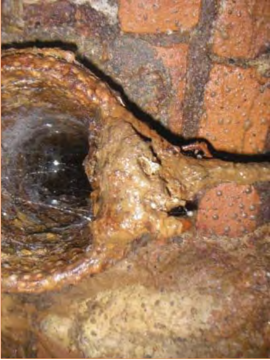
Photo 111. Building 2-A sanitary sewer: 004-008 Pipe connections (south pipe)
