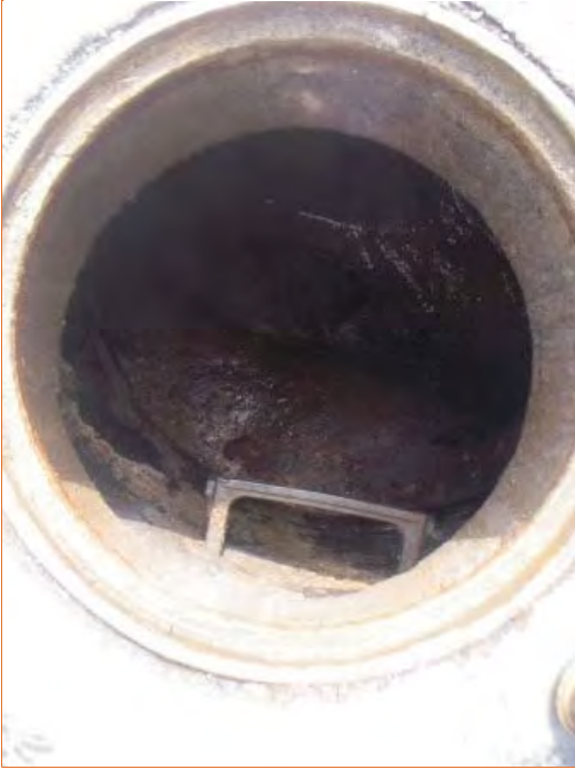
Photo 99. Outfall 004: 004-001 Manhole topside (north up)
