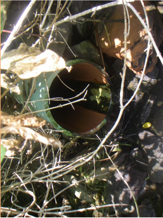
Photo 39. Outfall 013: Discharge point 013-000
