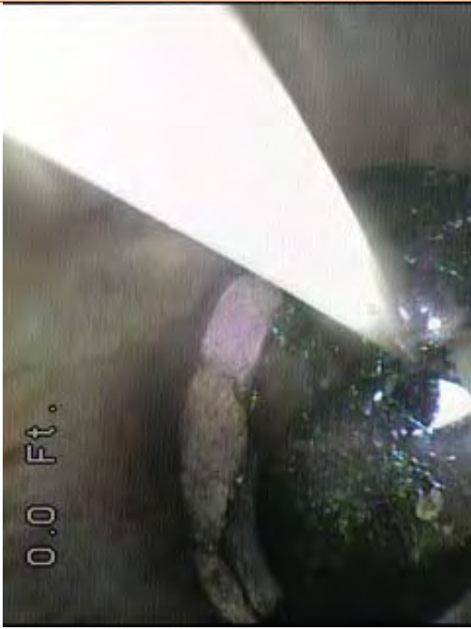
Photo 72. Outfall 005 (005-001A to 005-001): Roots and weeds at 10ft upstream of 005-001
