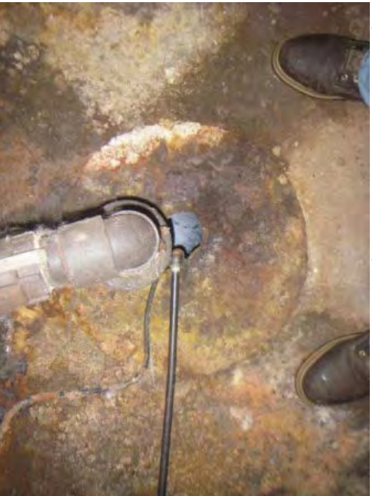
Photo 118. Building 1 : 007-003 floor drain topside. Note: 007-004 floor drain had a 8" x 14" grate with a 2" black PVC and a 1/4" diameter pipe
