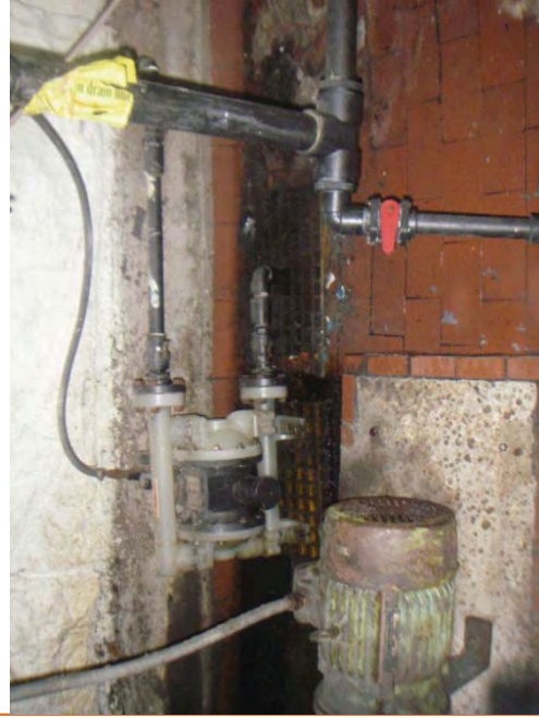
Photo 125. Building 4 floor drain near east wall
