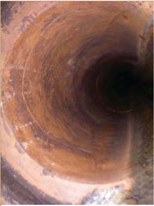
Photo 104. Outfall 004: 004-001 Pipe connections (east pipe)
