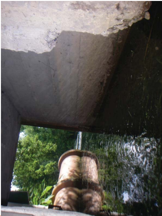
Photo 45. South view of culvert wall west of Outfall 008
