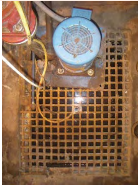
Photo 106. Outfall 004: 004-002 floor drain topside (north up)
