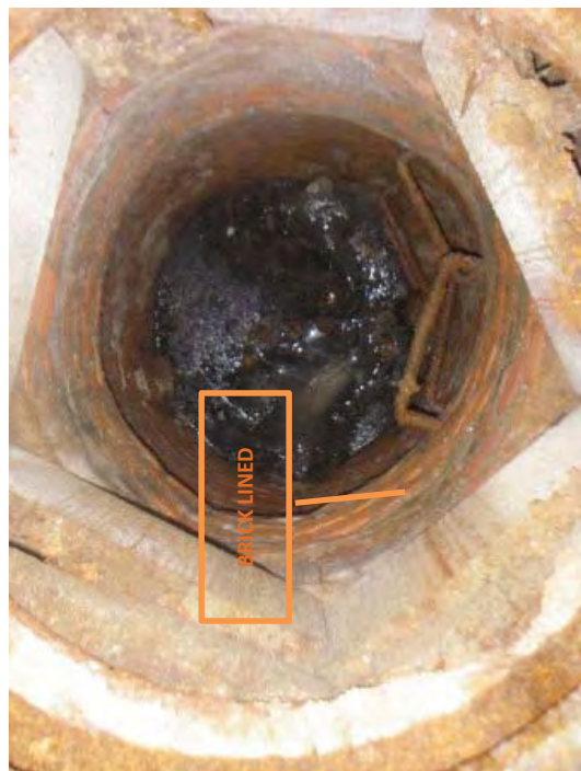
Photo 109. Building 2-A Sanitary sewer: 004-008 Manhole topside (north up)
