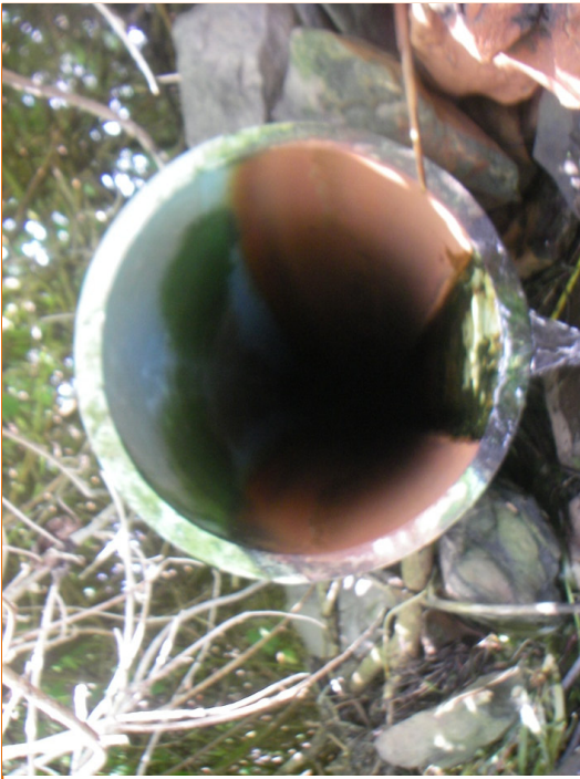
Photo 40. Outfall 013: Interior of 12" diameter discharge point 013-000
