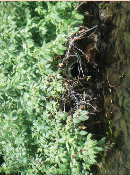
Photo 38. Outfall 013: Discharge point 013-000
