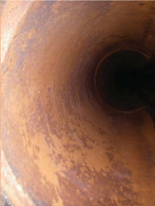
Photo 115. Outfall 007: 007-001 Pipe connections (west pipe)
