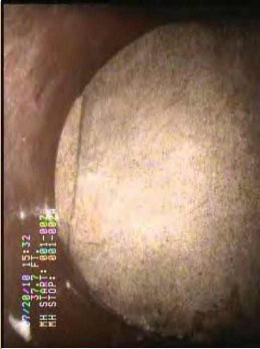
Photo 48. Outfall 001 (001-001B to 001-001): Cement plugged lateral south of 001-001B which seems to correspond to Outfall 002
