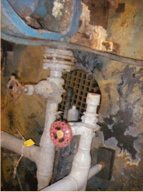
Photo 123. Building 3 floor drain near northeast wall
