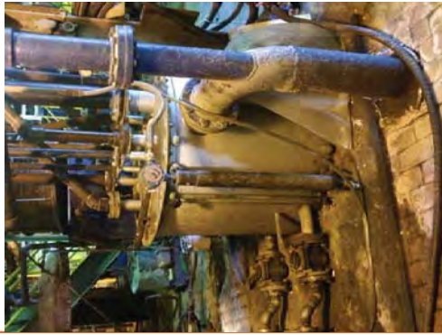
Photo 137. Former Hotwell 2A; concrete paved with AST and inlet piping
