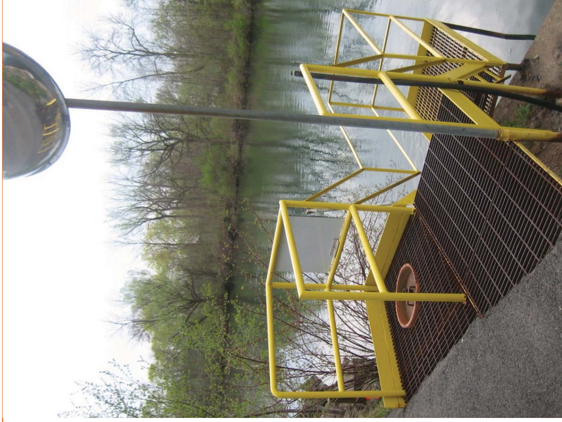
Photo 10. Outfall 005: Location for smoke blower at 005-000A vertical pipe
