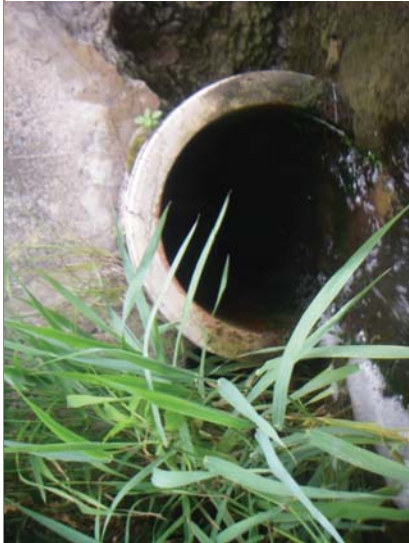
Photo 19. Outfall 001: 12" Diameter discharge point 001-000
