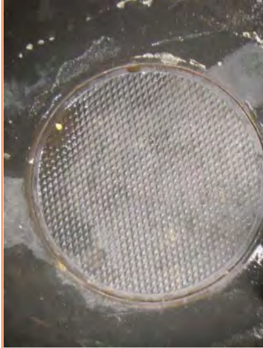
Photo 108. Building 2-A sanitary sewer: 004-008 Manhole cover
