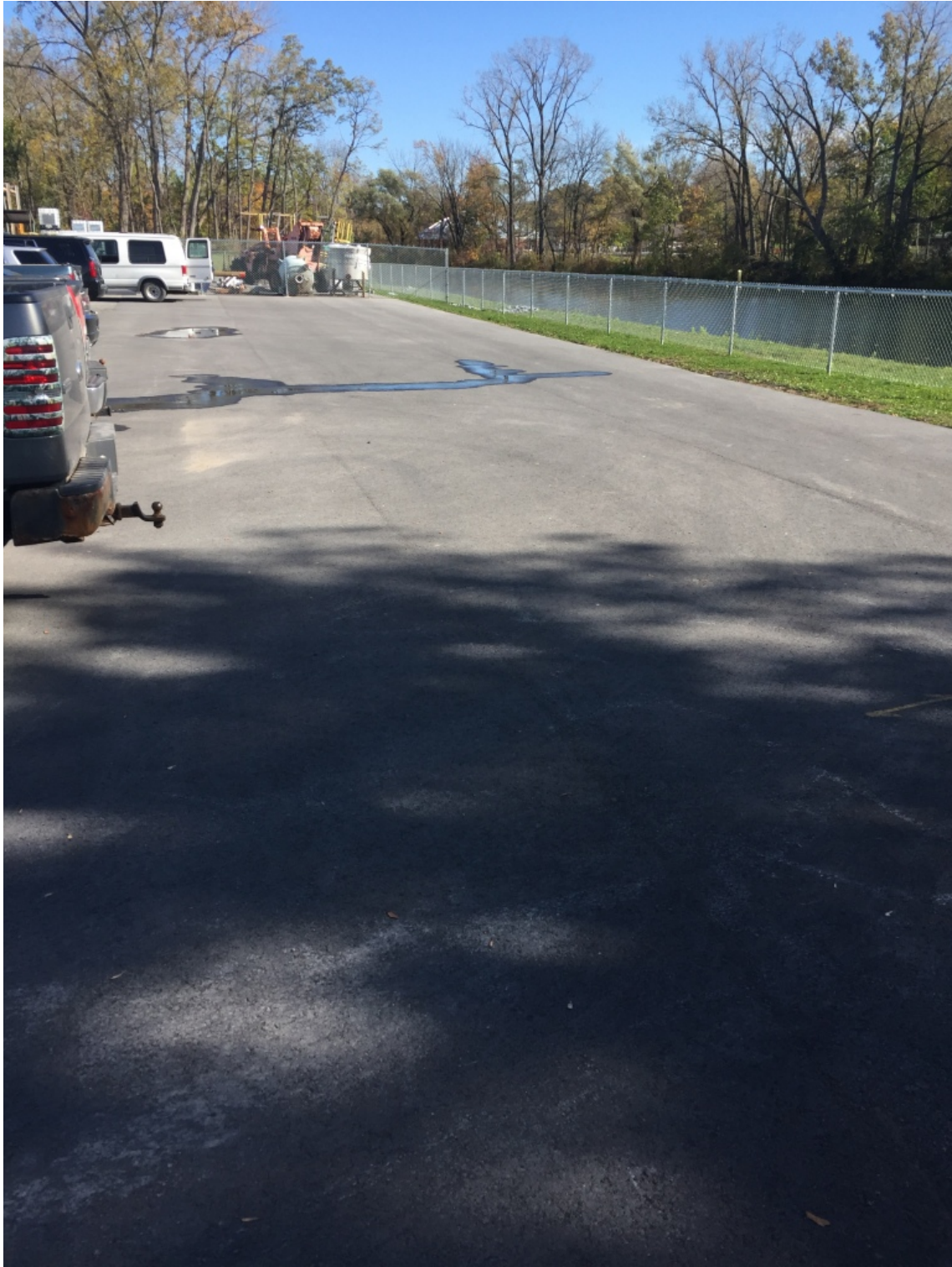
Asphalt Cover Area
