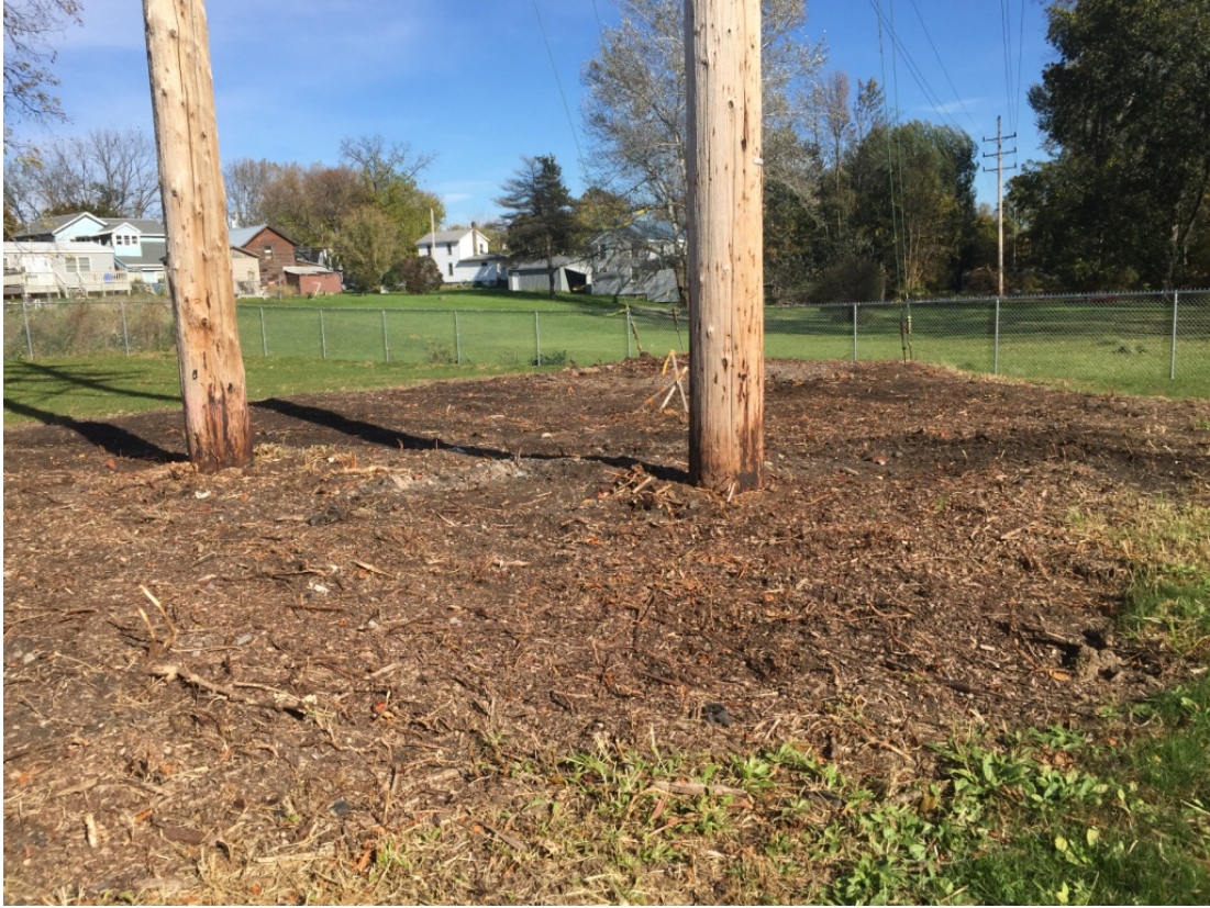
Tree Clearing around Power Poles
