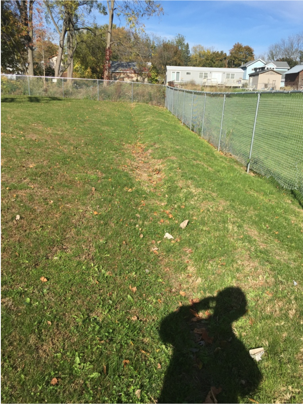
Drainage Swale Located on East Side of Cover Area
