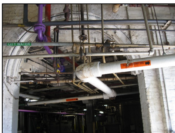
Photo 5. Example doorway between buildings, showing the difficulty of airsealing
