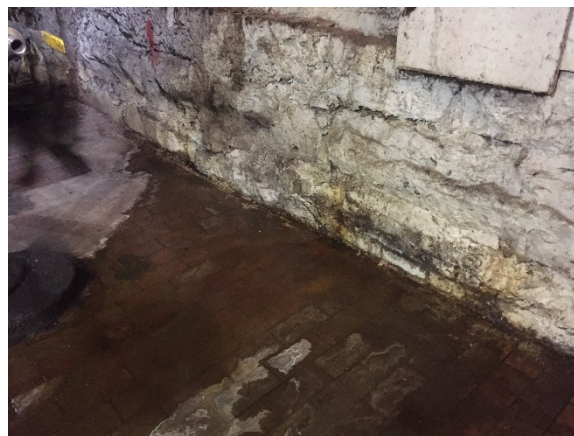
Photo 7. Water seeping from the northern wall of Building 4 near SV-12 during spring of 2017.
