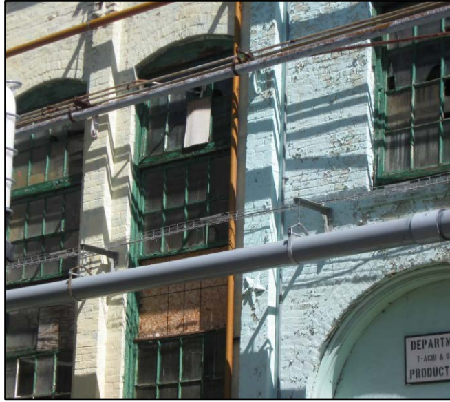
Photo 4. Detail Windows on West Facade of Building 4, Showing Mix of Conditions
