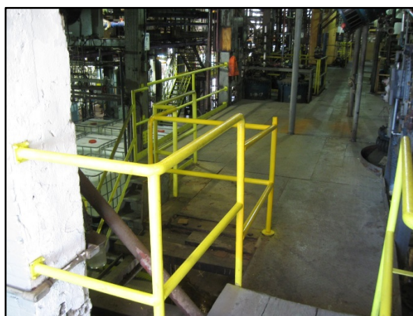
Photo 6. Doorway on west facade of Building 4, showing presence of handrail that would make installation of a door and sealing difficult.
