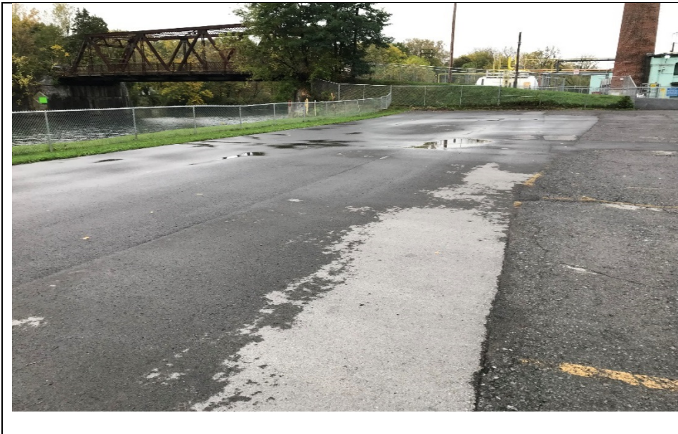
Southern end of Gorham Street area asphalt cap (looking west).
