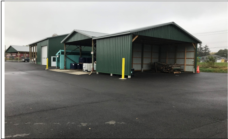
North side of asphalt cap (looking west).
