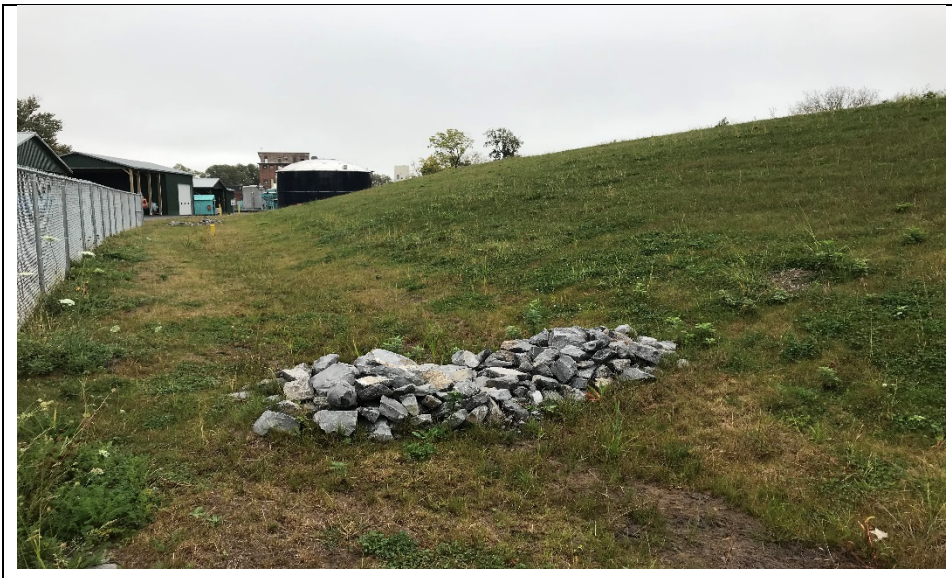
Northern side of SWMU-1 drainage swale and rock check dam (looking east).
