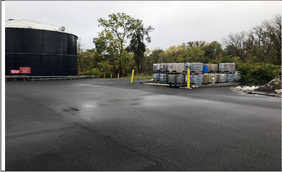
Eastern end of asphalt cap (looking east).
