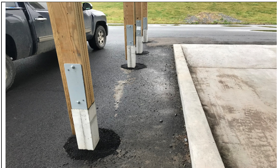
Sealed asphalt cap penetrations for new storage buildings.
