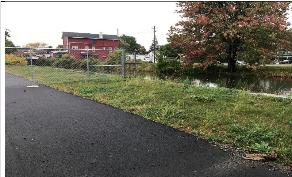
Western end of asphalt cap (looking northwest).
