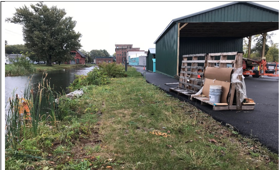
North side of asphalt cap (looking east).
