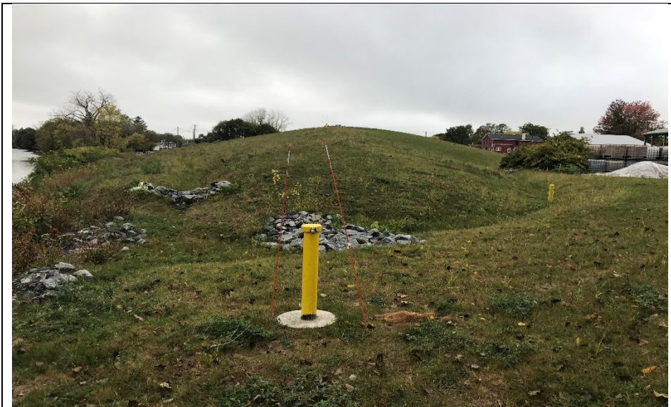
Eastern end of South Side of SWMU-1 (looking west).
