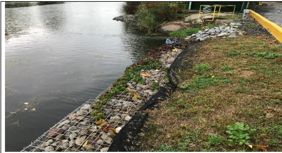
Western end of Gabion Wall (looking west).
