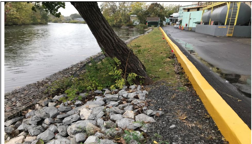
Eastern end of Gabion Wall (looking west).
