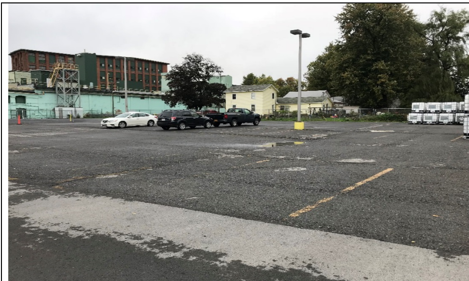
Gorham Street area asphalt cap (looking north).
