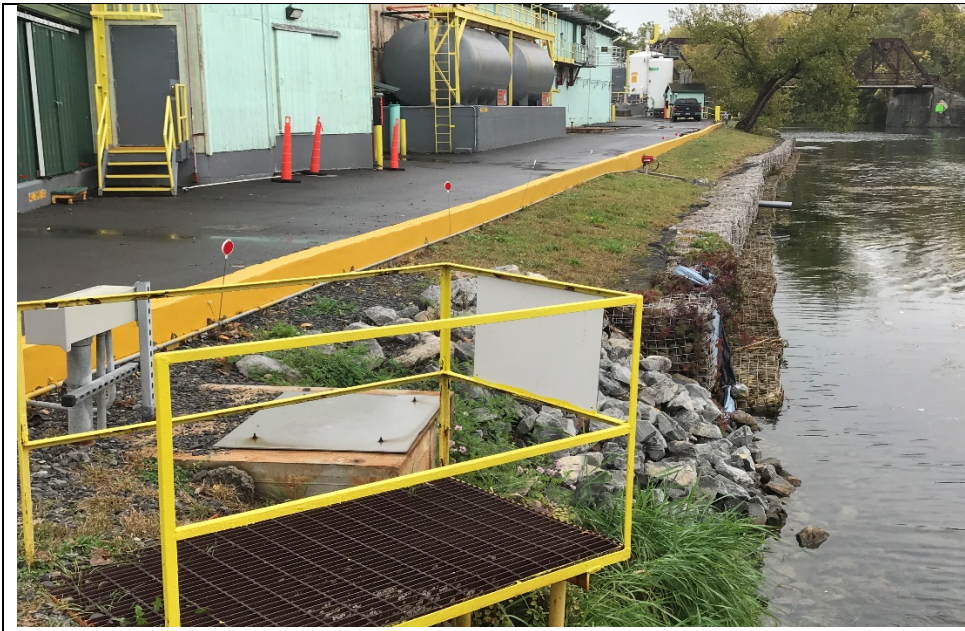
Western end of Gabion Wall (looking east).
