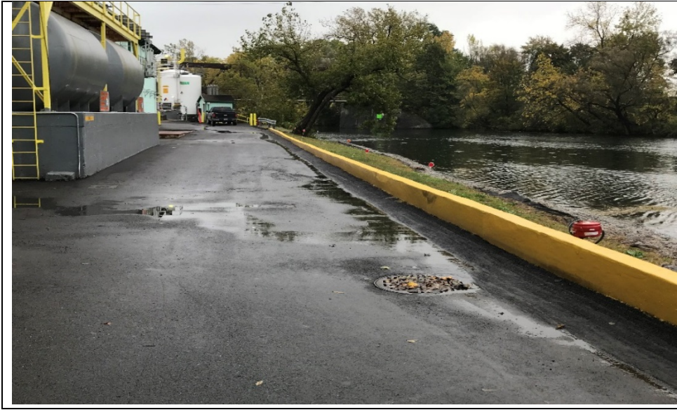
Western end of Gabion Wall Access Road (looking east).
