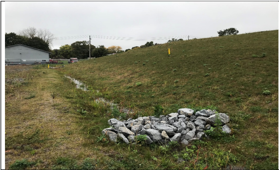
Western end of south side of SWMU-1 (looking west).
