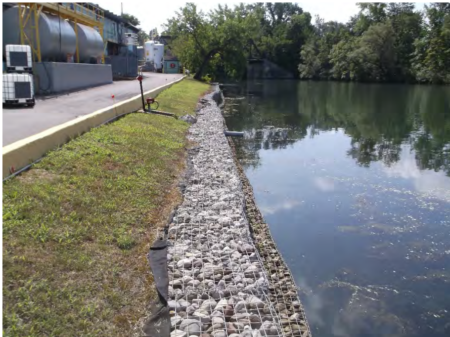
Photograph 12: View of gabion alignment (looking east).
