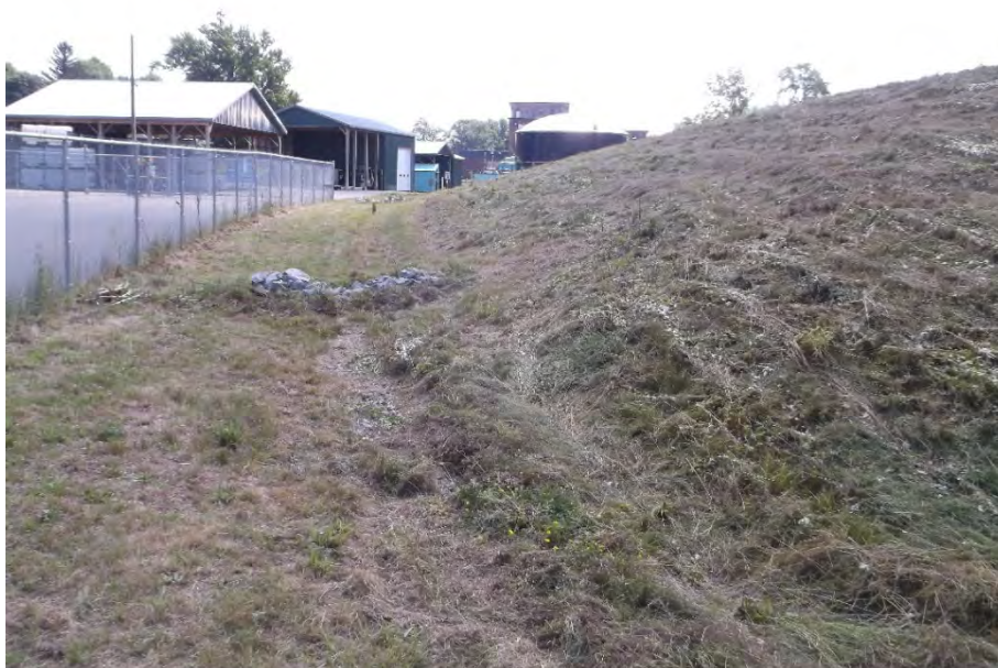
Photograph 22: Portion of SWMU-1 cover system immediately following cutting (looking east) with swale system and check dams visible.
