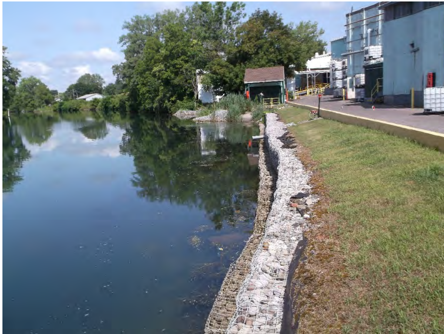
Photograph 13: View of gabion alignment (looking west).
