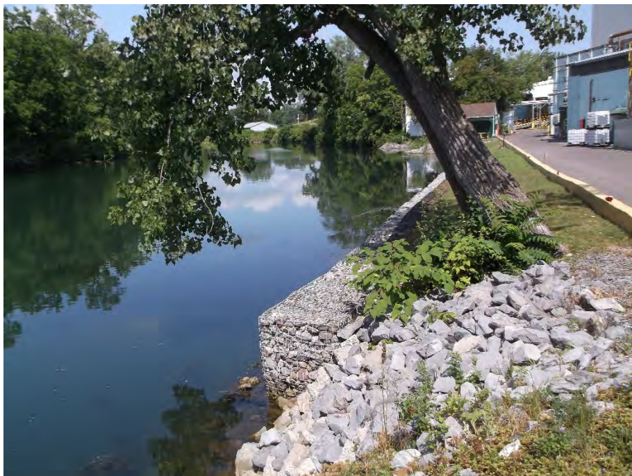
Photograph 14: View of gabion alignment (looking west) – rip-rap at termination for stormwater management.
