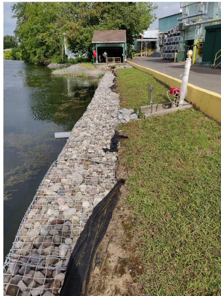
Photograph 15: View of gabion alignment, including stormwater control outfall (looking west).
