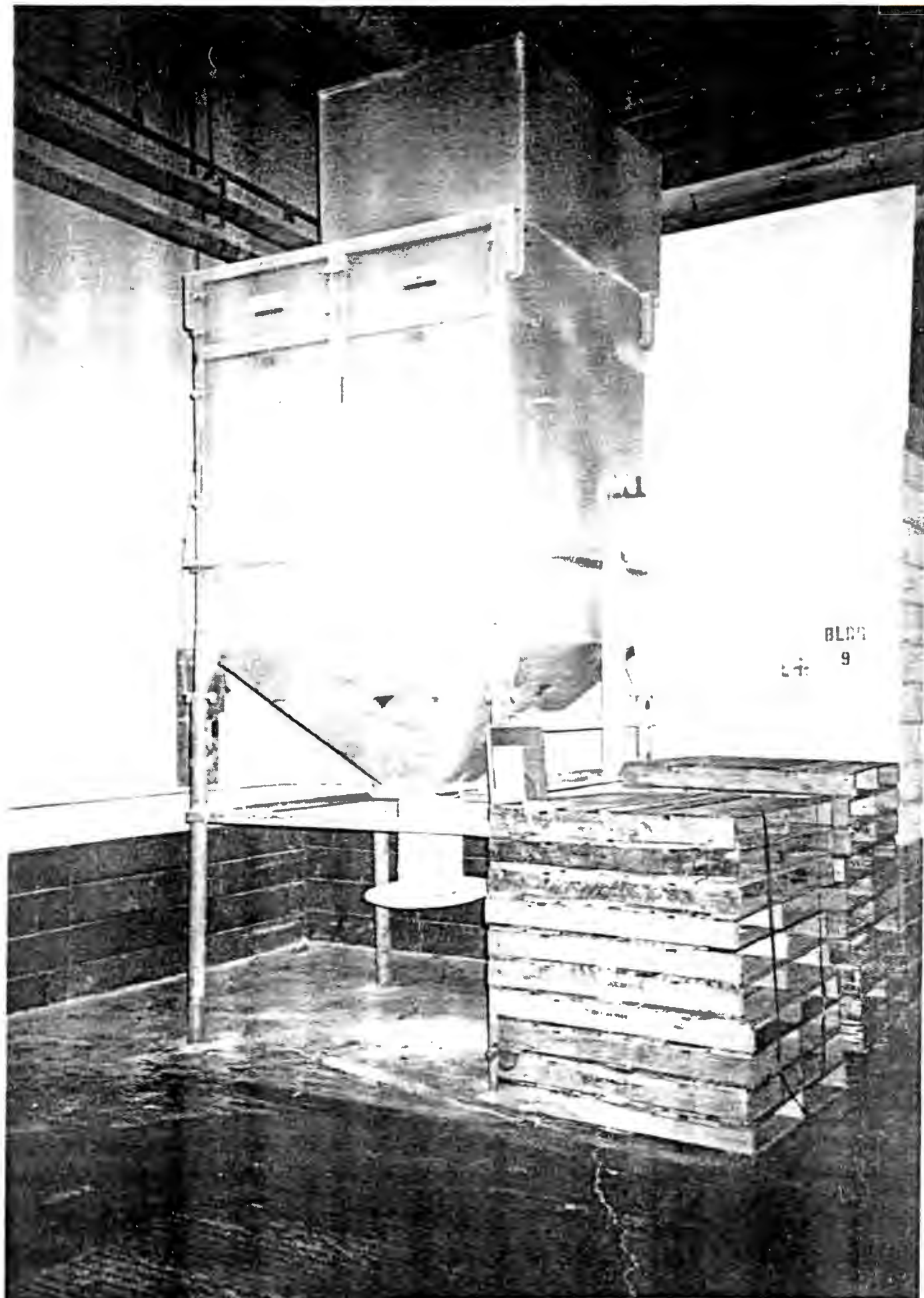
Figure 4 Glass Buffing Dust Collector Building No. 9
