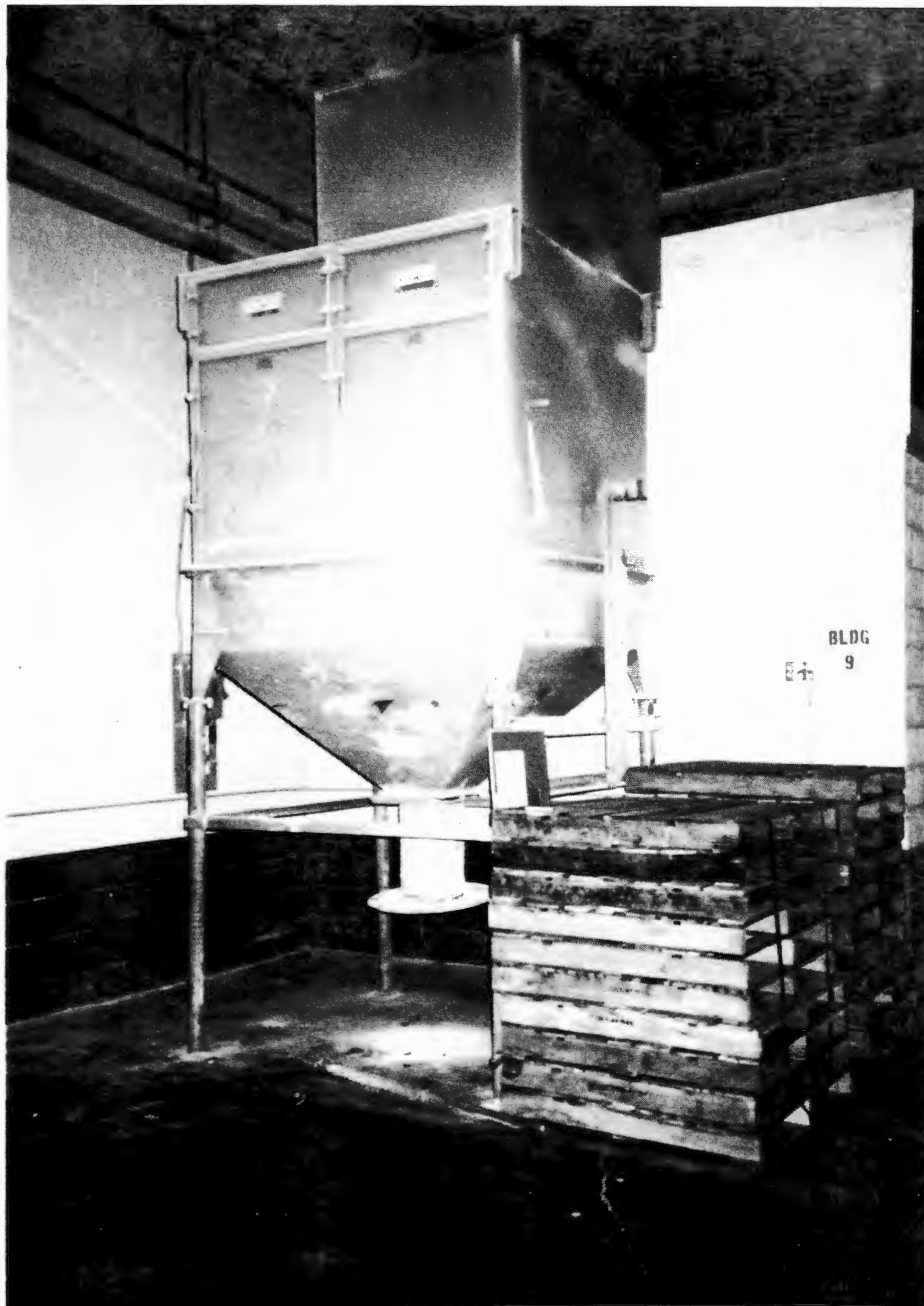
Figure 4 Glass Buffing Dust Collector Building No. 9
