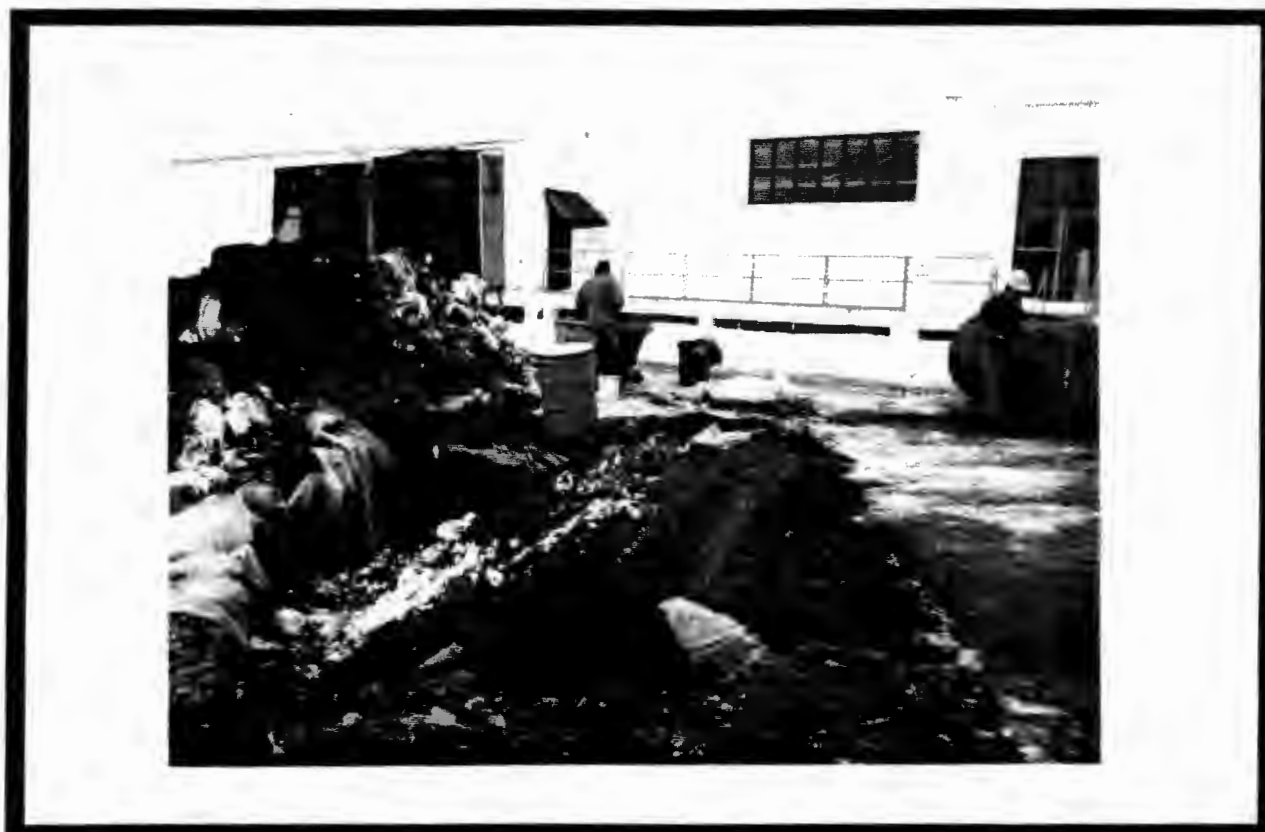
Photo #8: BACKFILLING UST EXCAVATION WITH IMPORTED CLEAN FILL. (LOOKING WEST)
