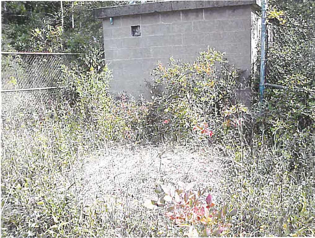
1. Flowhouse and Manhole MH12
