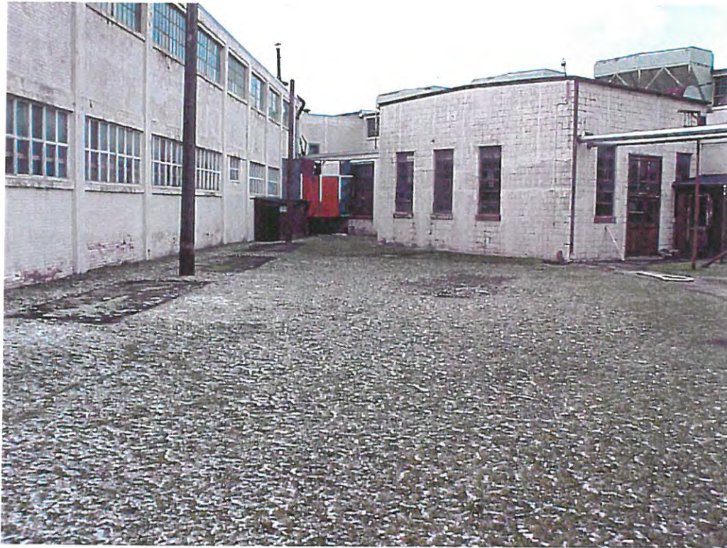
21. Concrete pads where former transformers existed along Building 2.
