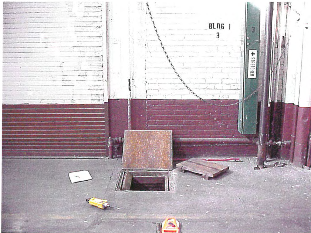
3. Pit and tunnel located in the west end of Building 1.
