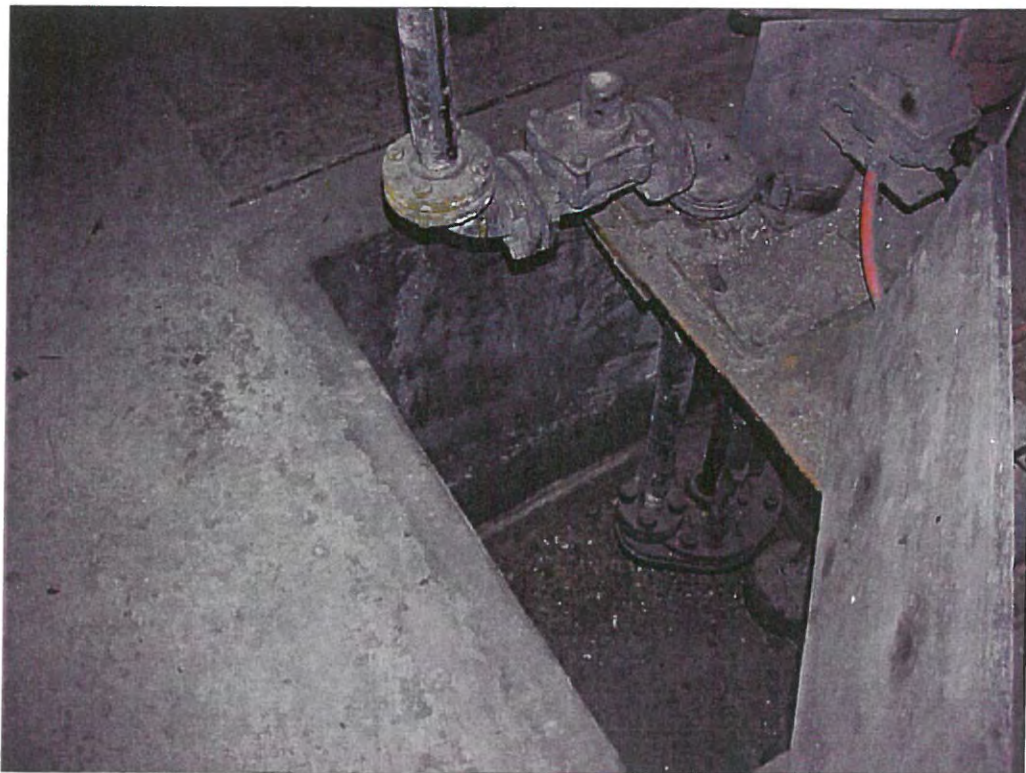
2. Empty pit with sump pump associated with the former industrial WWTP (no sludge in bottom).
