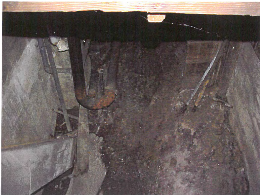
4. Looking into the pit/tunnel with earthen bottom, used for steam pipes, etc.
