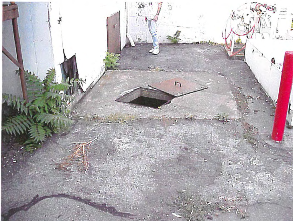
10. Pit located in truck dock area near Building 9B.
