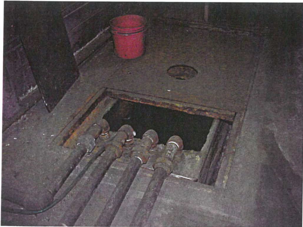
8. Blowdown pit next to Boiler Room in Building 11.
