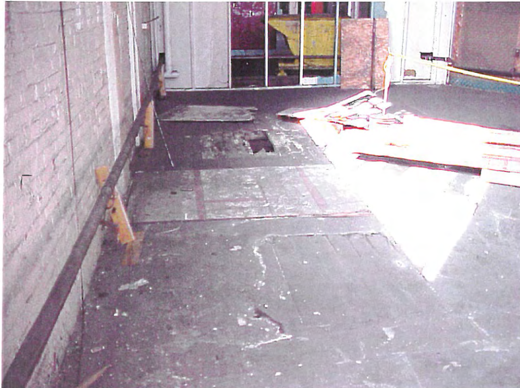
6. Covered pit in Building 3 containing sludge (unknown former use).
