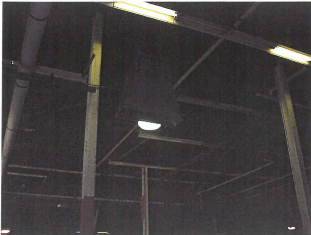
4. Former vent through roof from vapor degreaser.
