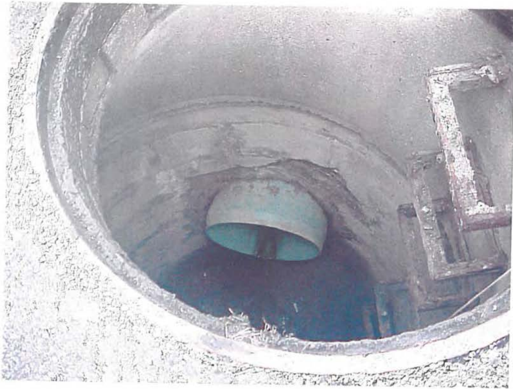
21. Example of a storm sewer where tie-in is cemented in well.
