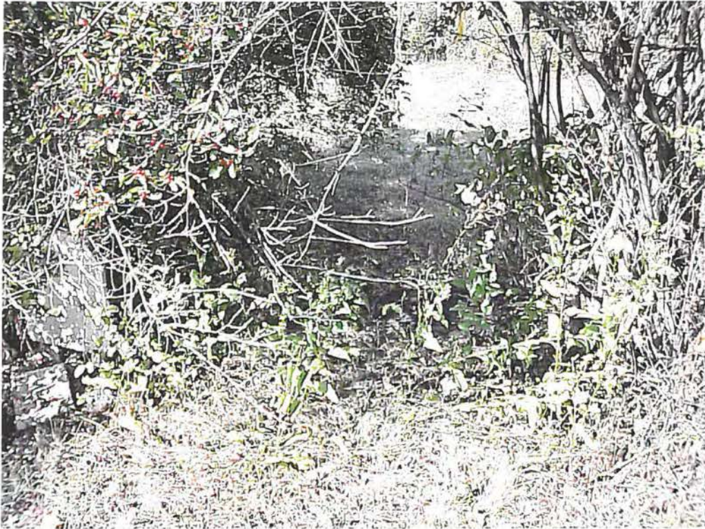
15. Manhole MH9 under bushes
