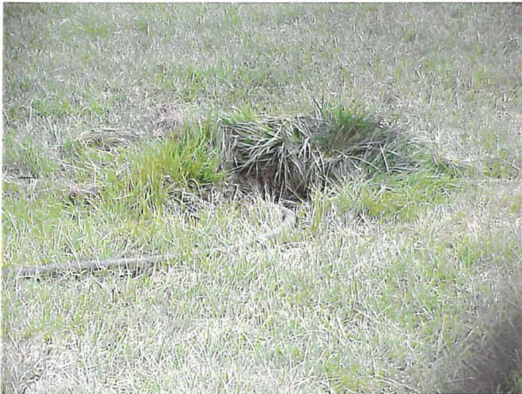
6. Catch basin near sanitary sewer lift station.
