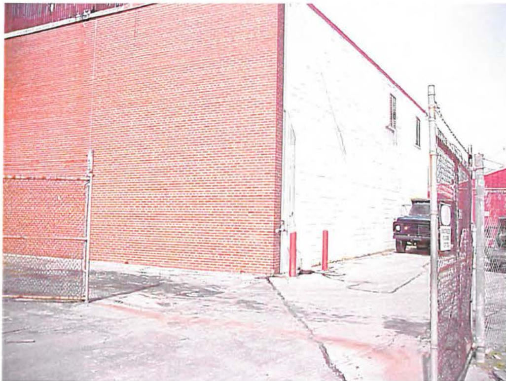
2. View of the TCE standpipe next to a re-routed PVC roof drain.
