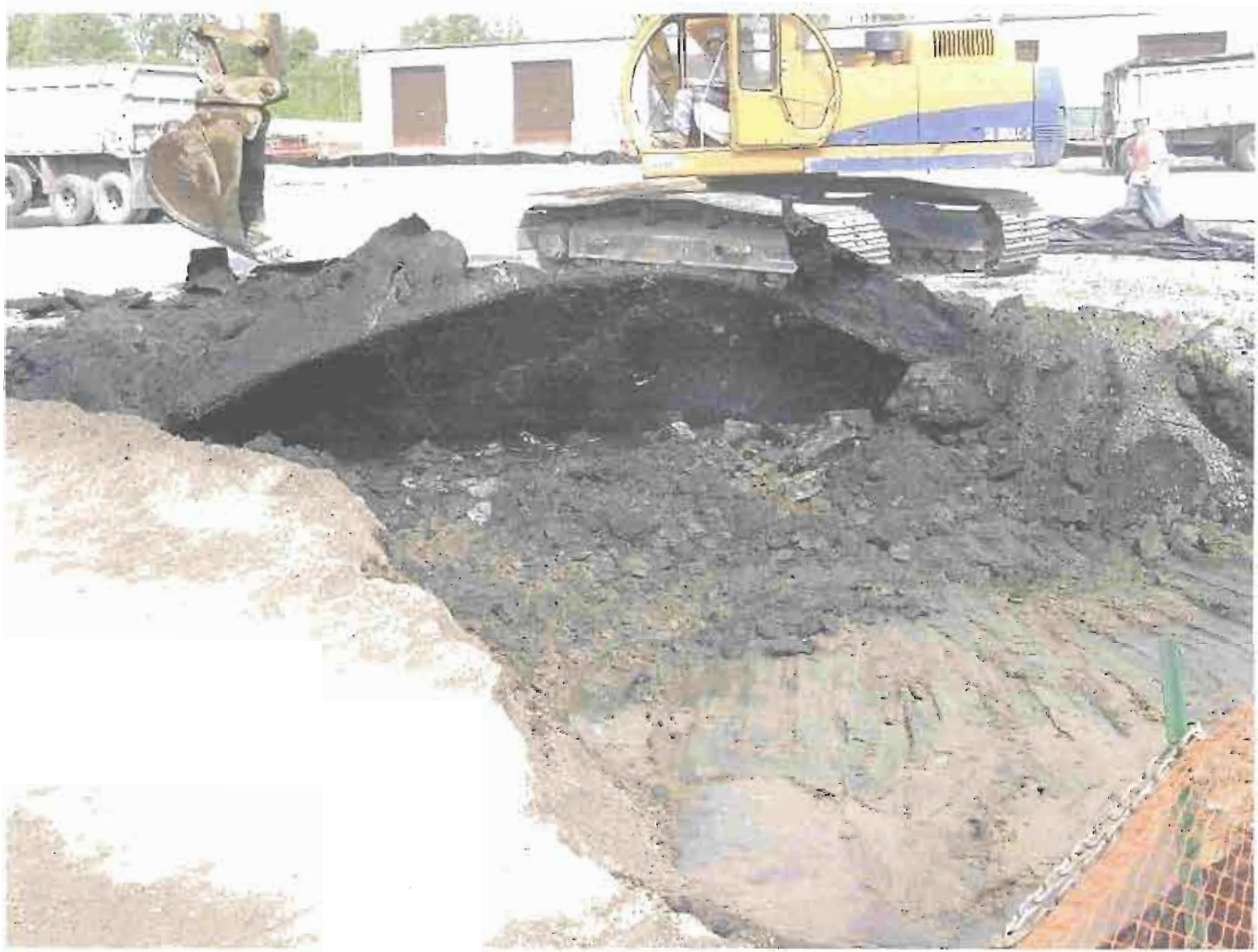
2004 REMEDIATION PROJECT PHOTO NUMBER 9
