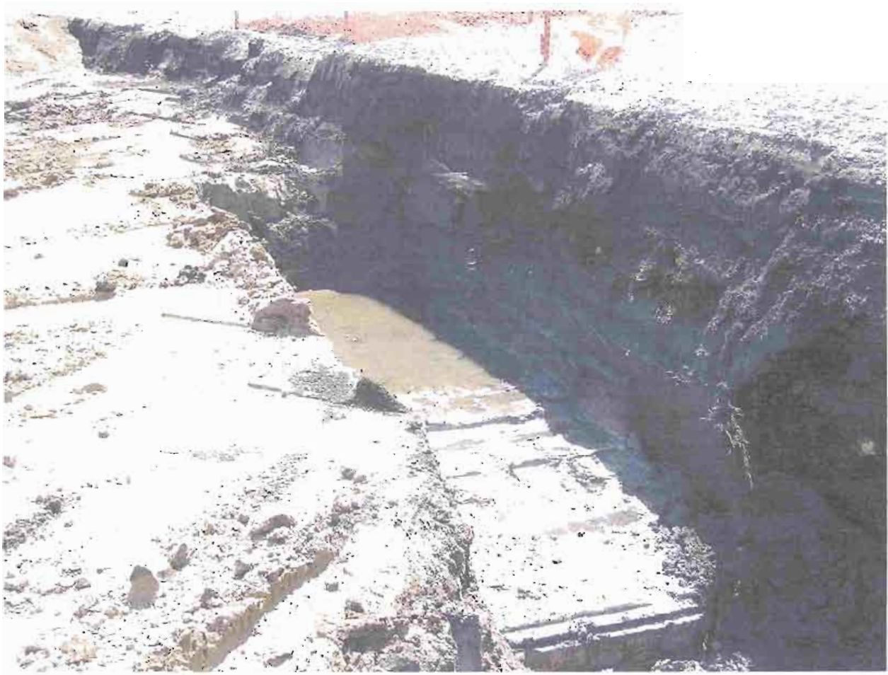
2004 REMEDIATION PROJECT PHOTO NUMBER 18
