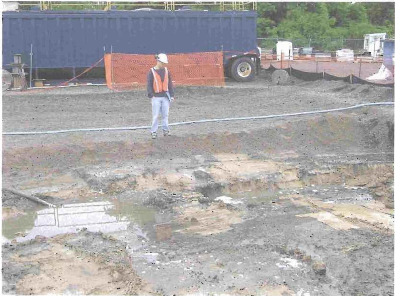
2004 REMEDIATION PROJECT PHOTO NUMBER 3
