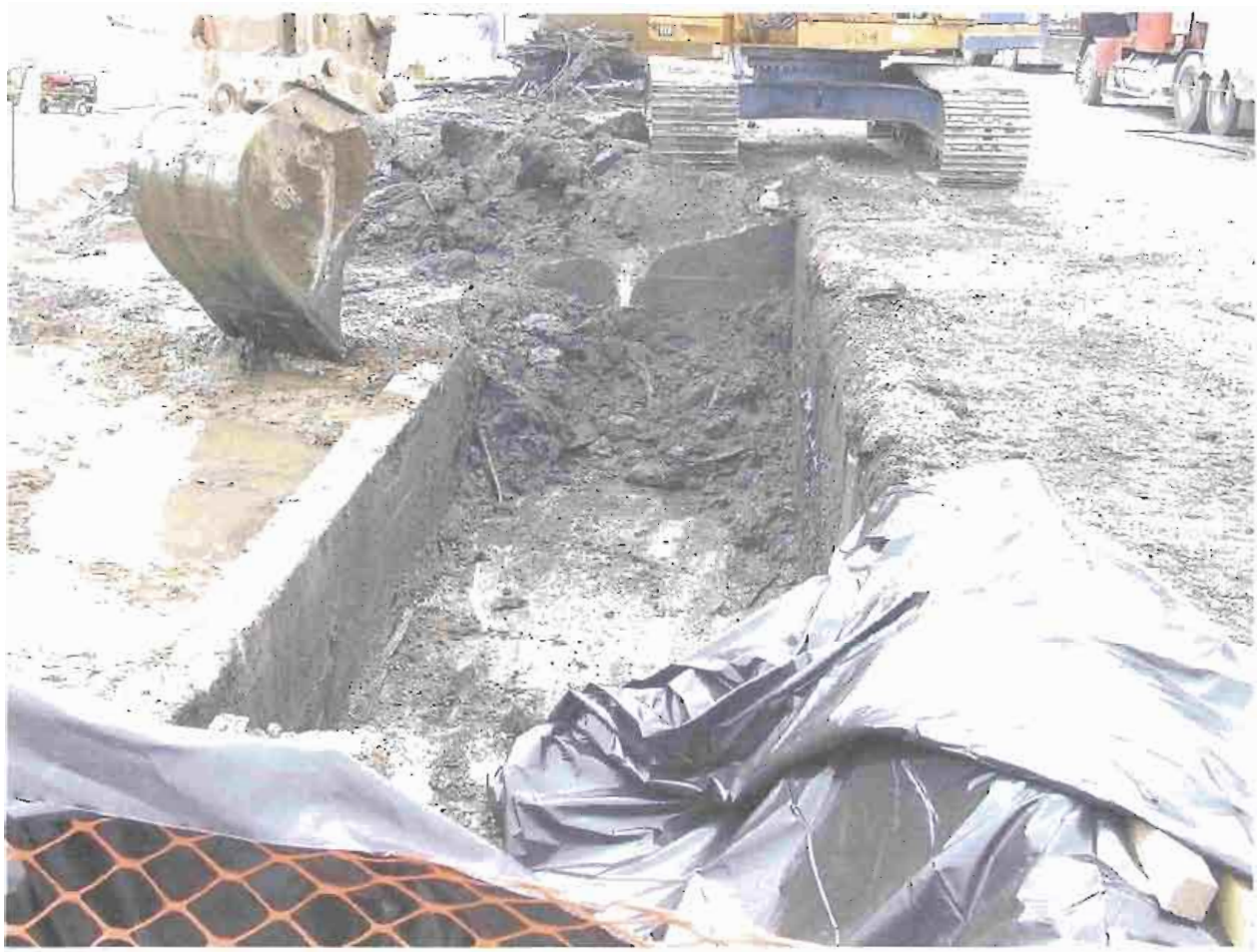
2004 REMEDIATION PROJECT PHOTO NUMBER 14
