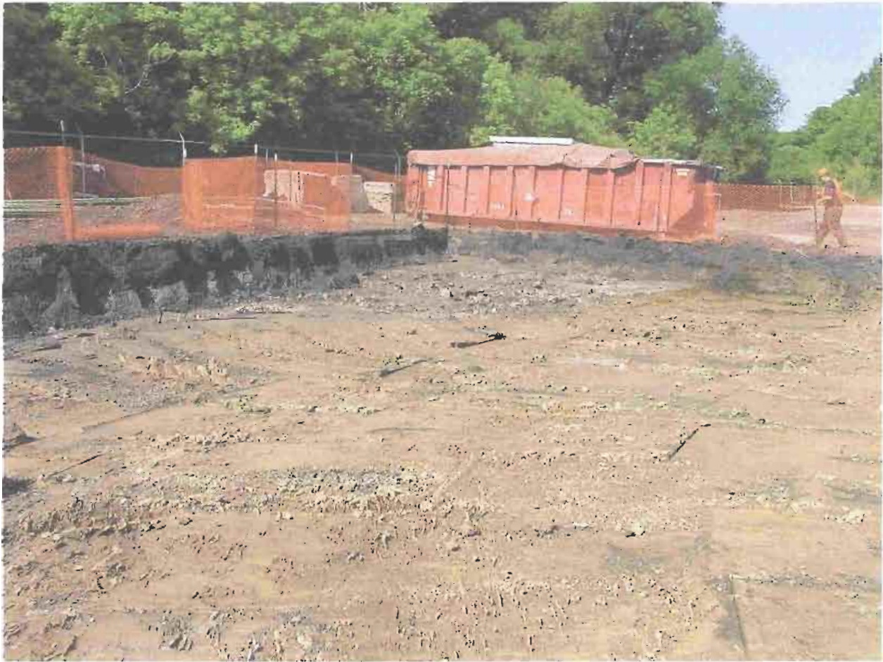
2004 REMEDIATION PROJECT PHOTO NUMBER 20
