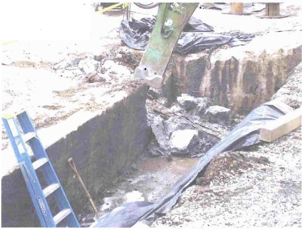
2004 REMEDIATION PROJECT PHOTO NUMBER 17
