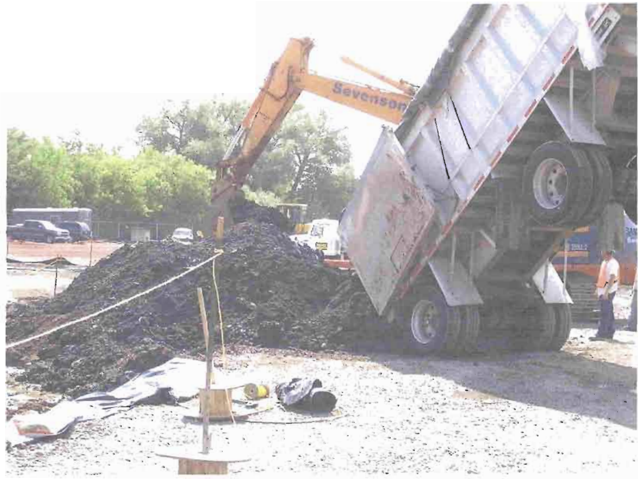
2004 REMEDIATION PROJECT PHOTO NUMBER 21
