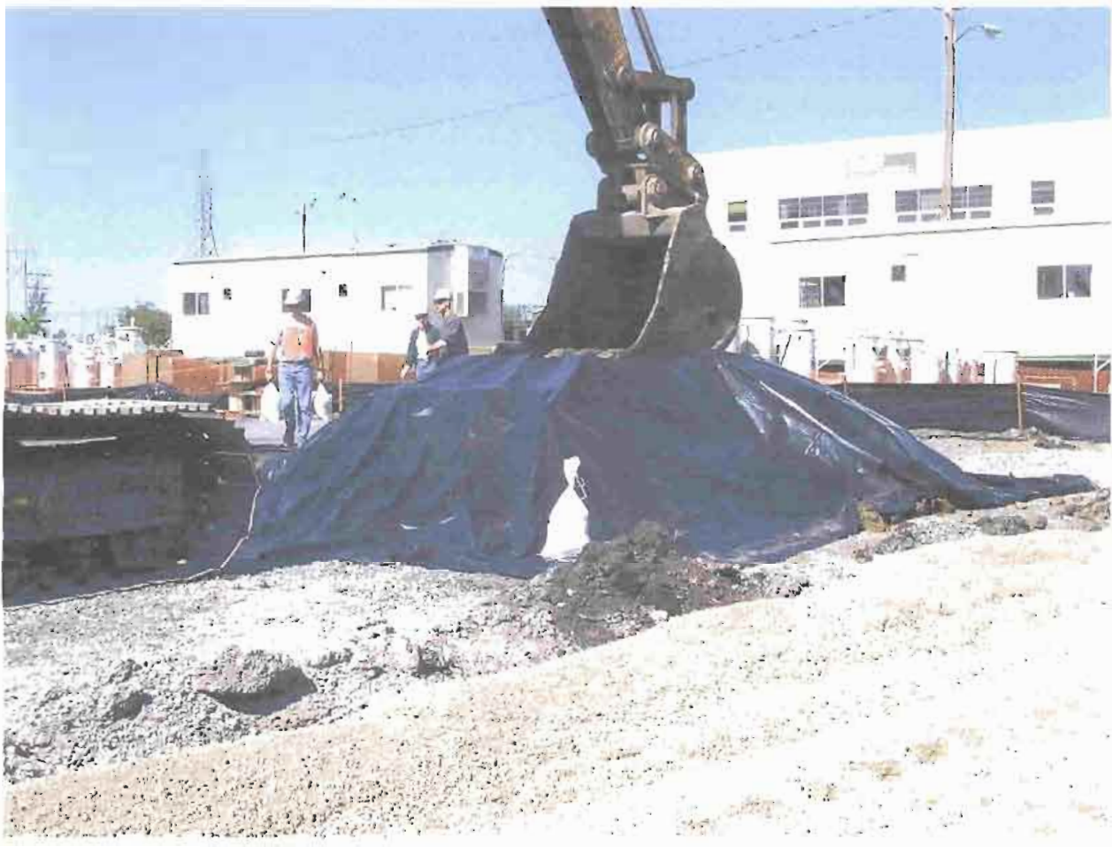
2004 REMEDIATION PROJECT PHOTO NUMBER 6
