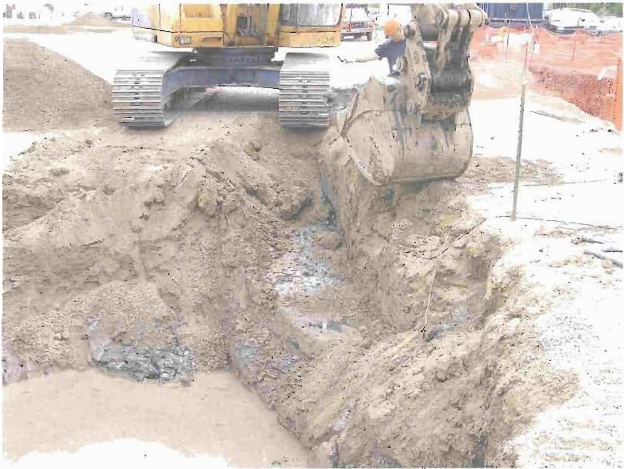
2004 REMEDIATION PROJECT PHOTO NUMBER 25
