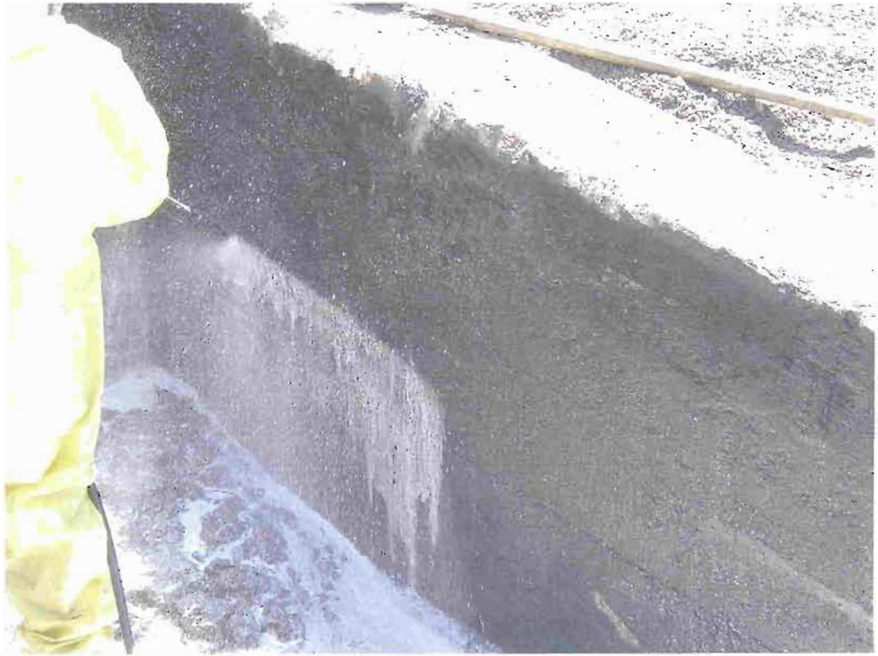
2004 REMEDIATION PROJECT PHOTO NUMBER 16
