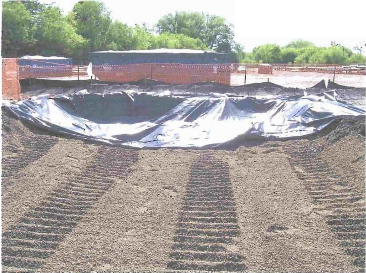
2004 REMEDIATION PROJECT PHOTO NUMBER 5
