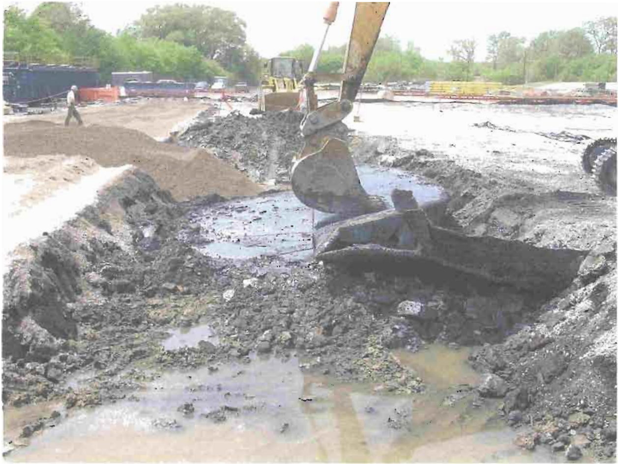
2004 REMEDIATION PROJECT PHOTO NUMBER 10
