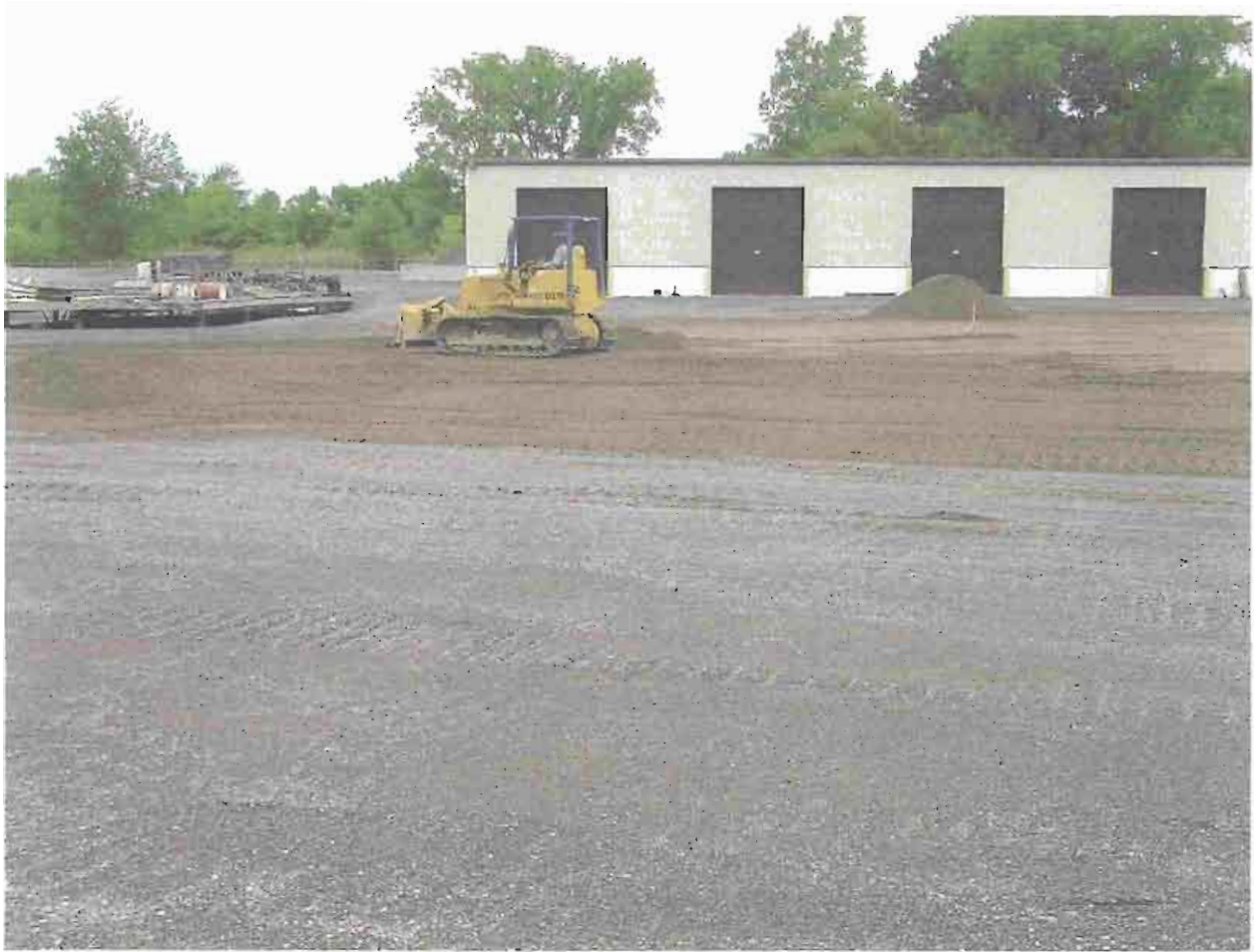
2004 REMEDIATION PROJECT PHOTO NUMBER 26
