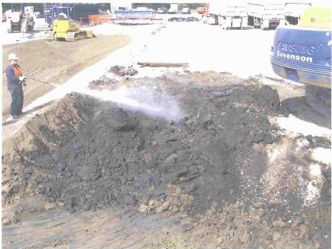
2004 REMEDIATION PROJECT PHOTO NUMBER 7
