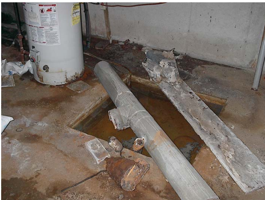
Basement sump surface water sample location (SW-2). (9/9/05)
