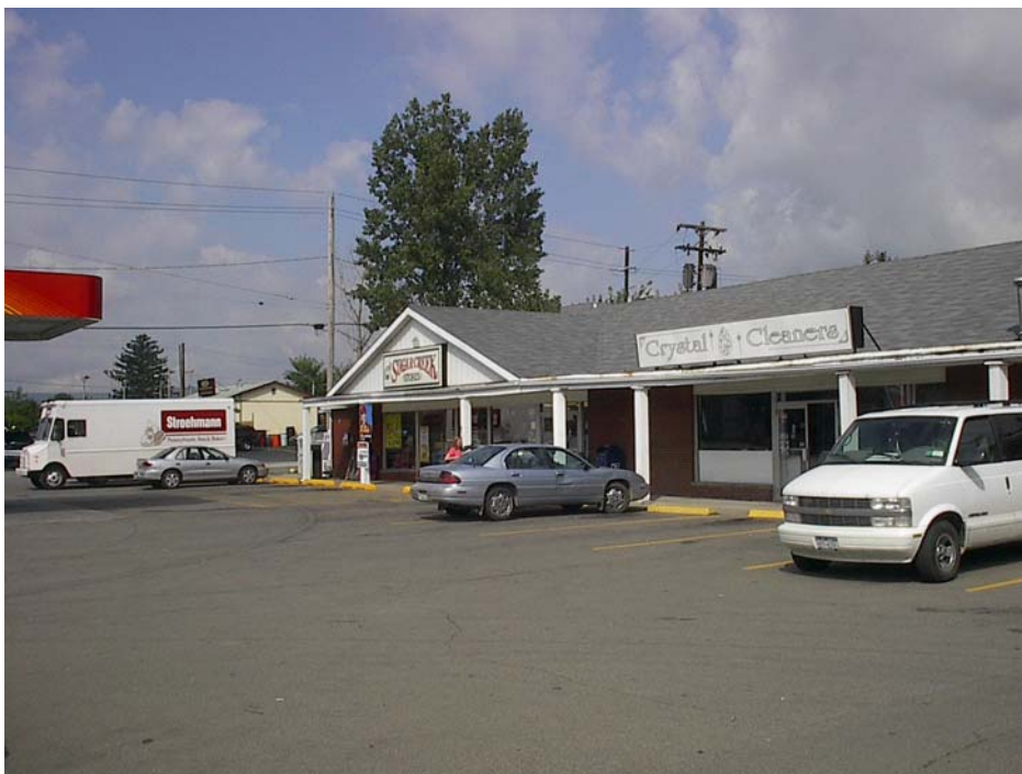
South side of the Site building. (9/9/05)
