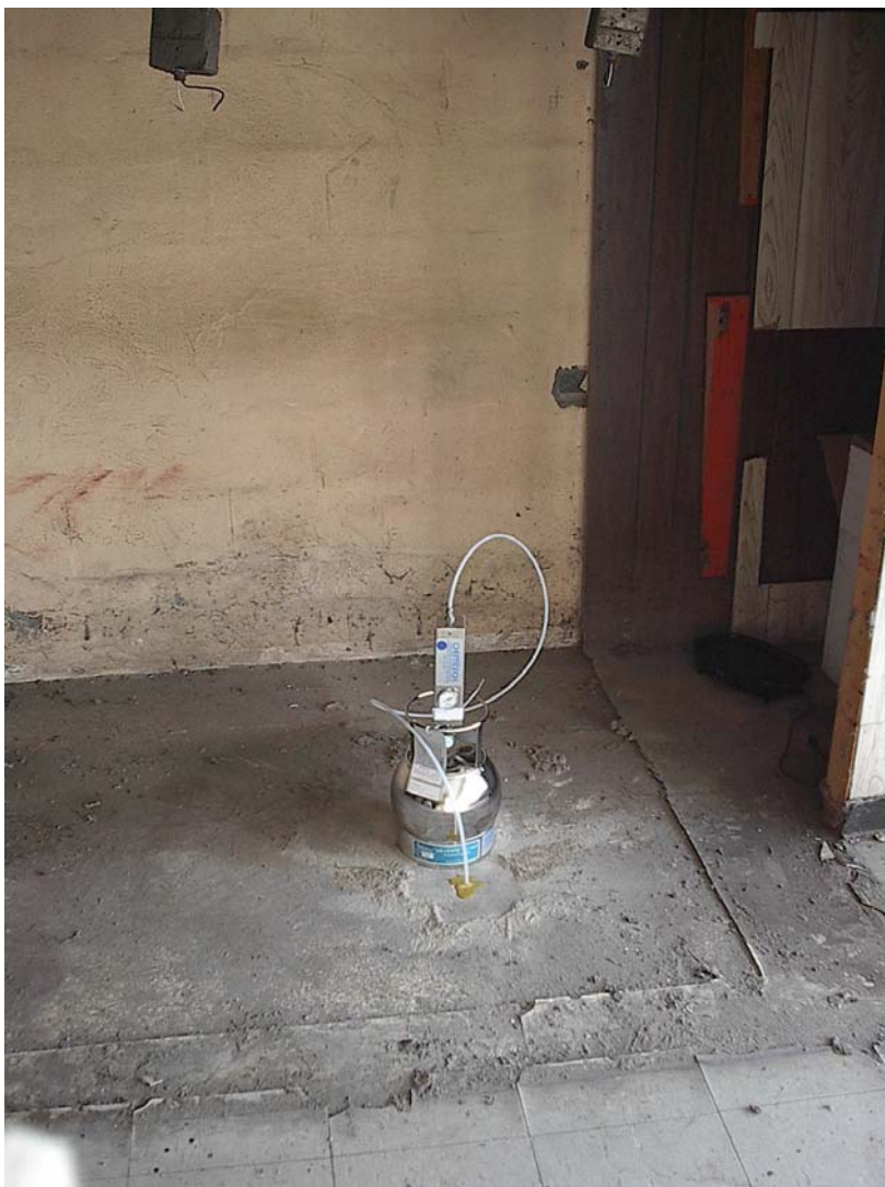
Sub-slab sample in south east corner of Site building (vacant space). (1/26/06)
