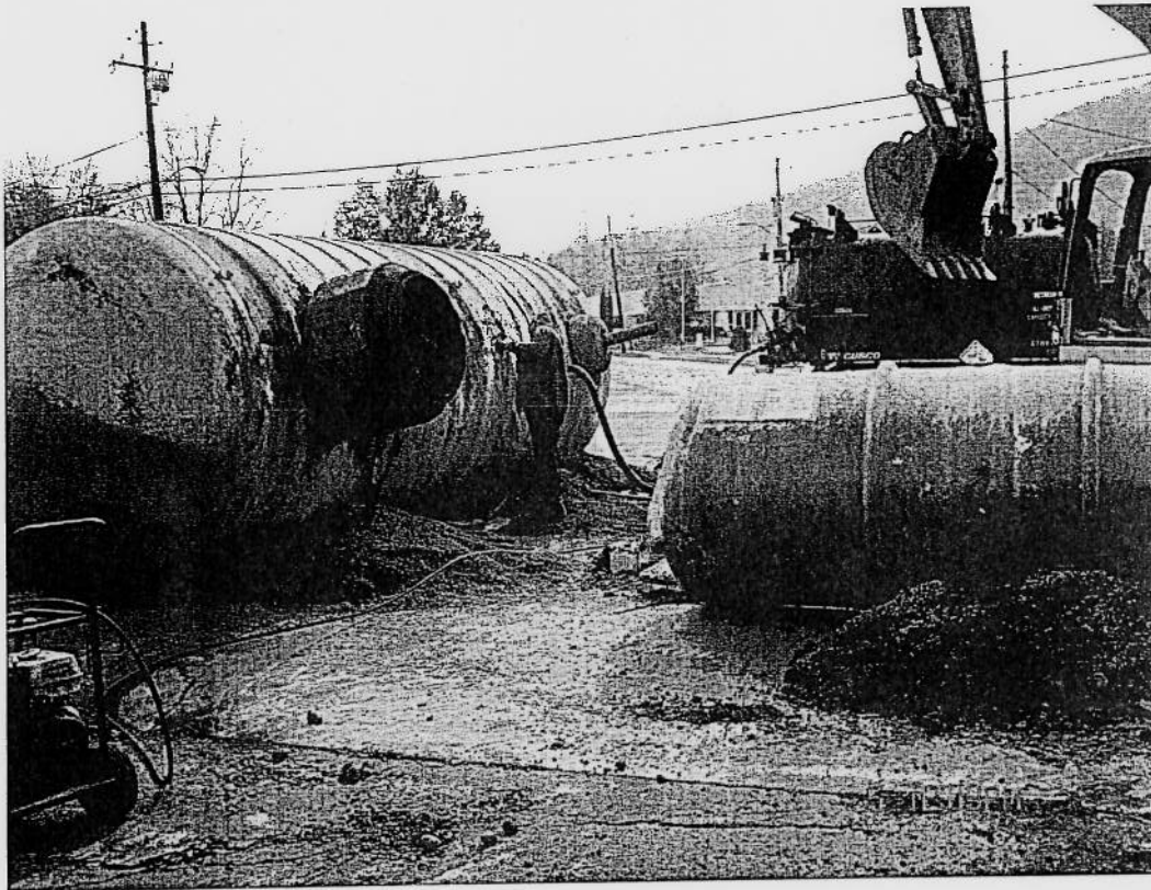
Photo 5: View South-Southeast showing removed G-1 (8,000-gal super unleaded gasoline) and K-1 (1,000-gal kerosene) tanks staged for disposal.
