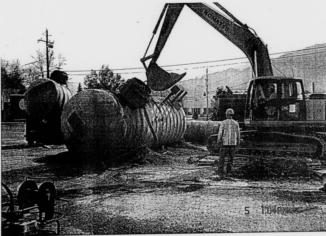
Photo 4: View Southeast of G-1, G2, and K-1 removed from tank pits.
