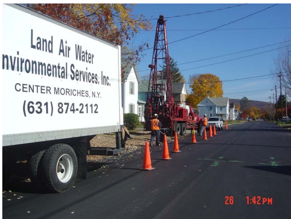
Monitoring well installation
