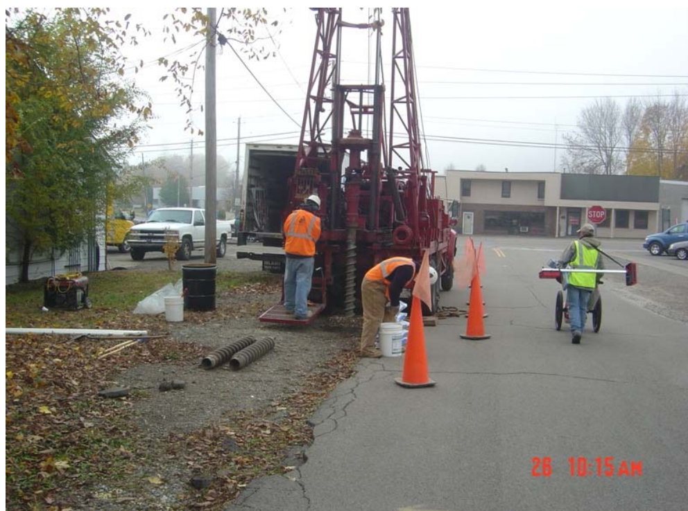
Monitoring well installation (Hollowstamp Augur), GPR Survey
