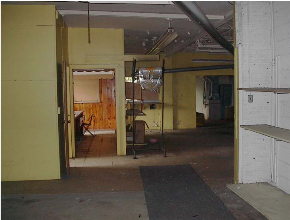
Looking west into customer area and center room of Site Building.
