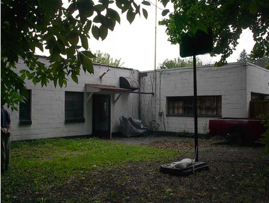
Southwest side of Site building – main door to work space.
