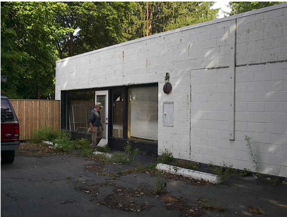
Southeast side of Site building – former laundry drop off location.
