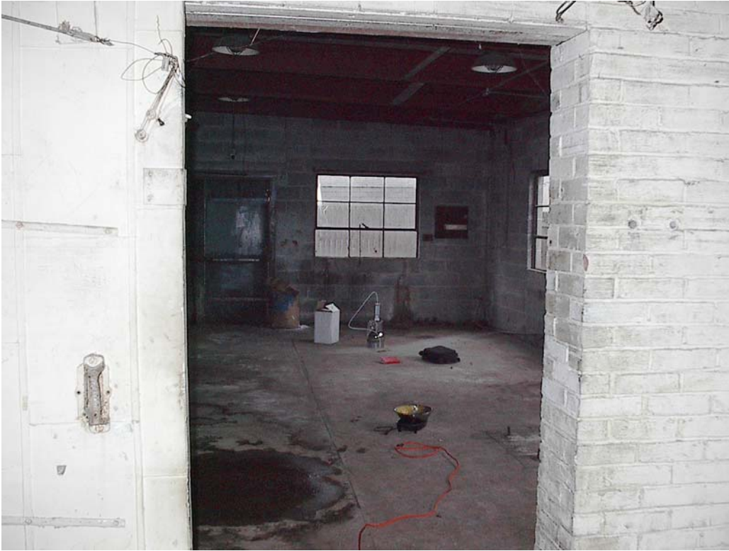
Former dry-cleaning room in northeast corner of Site building (picture facing west). (with Summa can and sub-slab sample)
