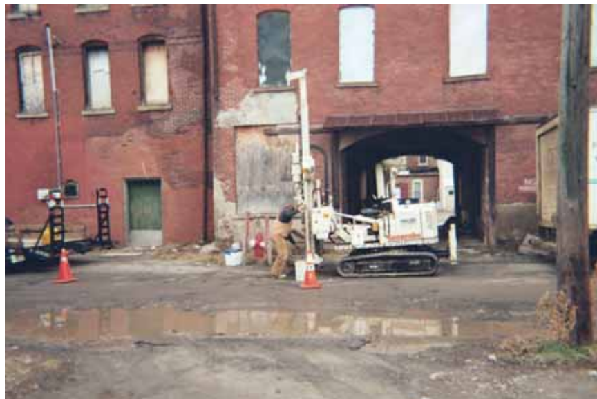
Date: 1/13/06 Subject: Direct-Push activities at the Band Box Cleaners Photographer: Jim Mays Site boring BB-BH-02
