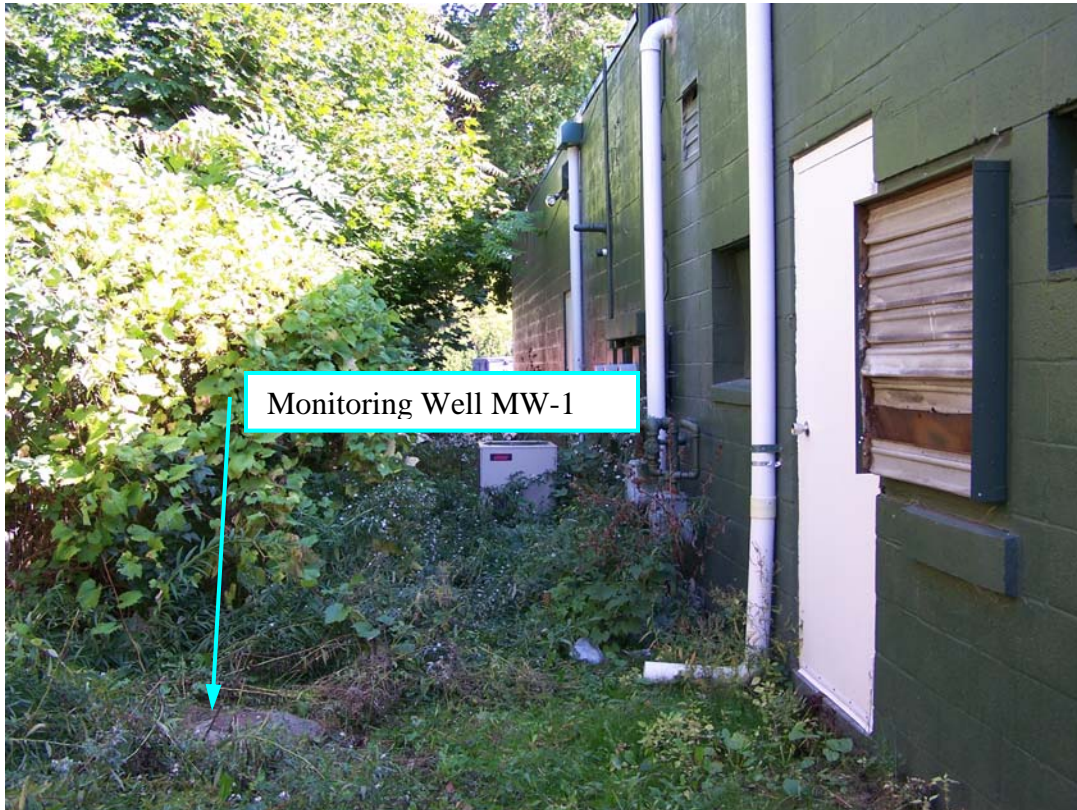
Looking east along rear of Site building. First door is the rear door of the former dry cleaners.
