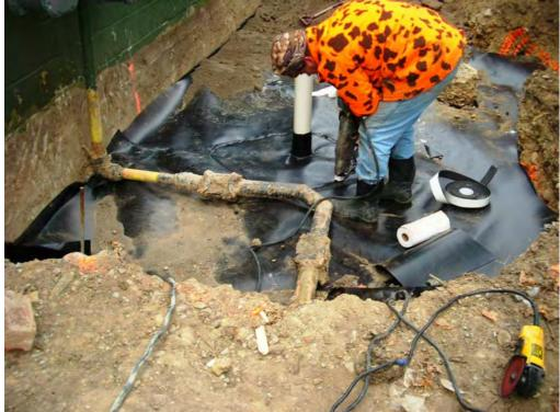
Welding seam around vapor well
