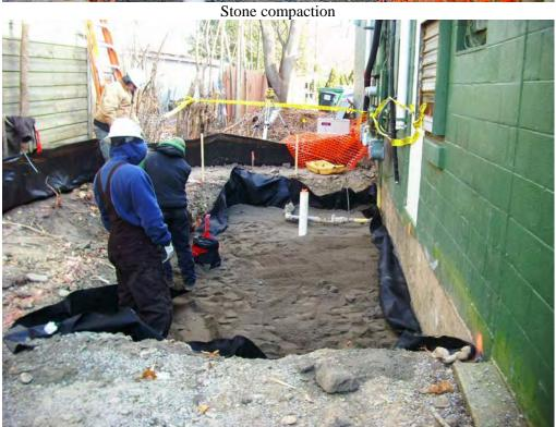
Sand installation (sand layer placed on geotextile)
