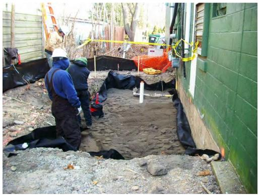
Sand installation (sand layer placed on geotextile)
