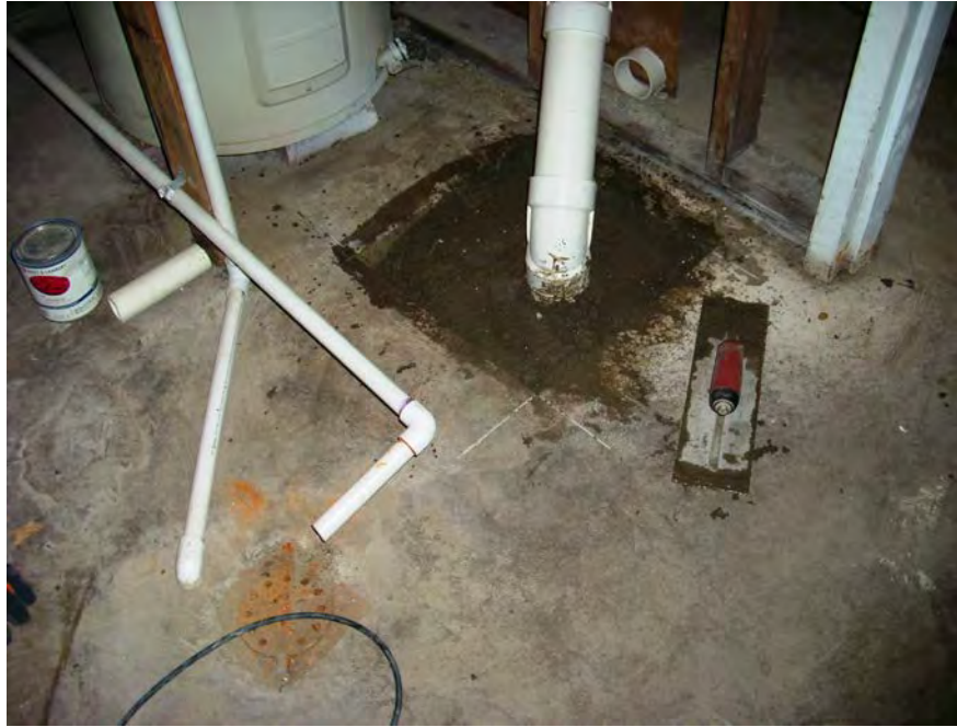
SVE Riser with Grout Seal
