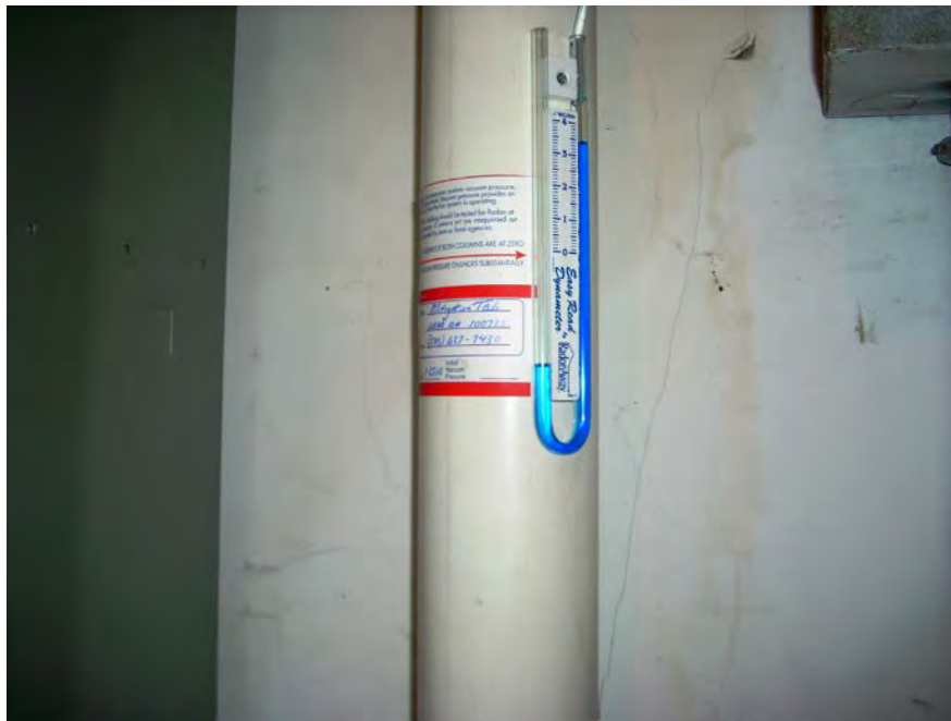
Installed Manometer
