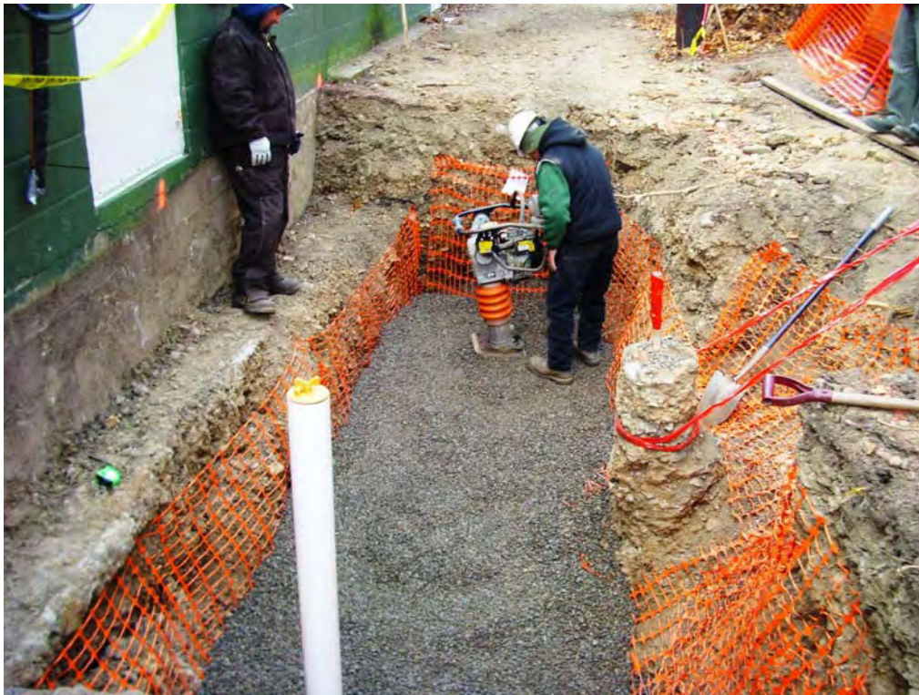
Stone compaction
