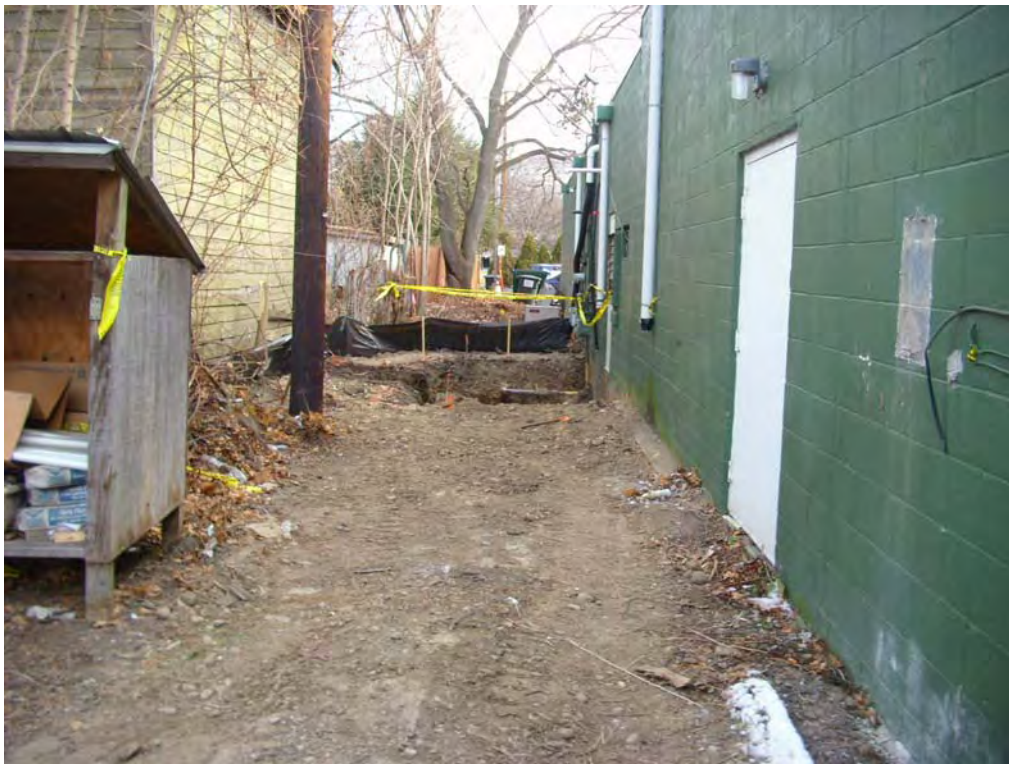
Work area (west to east)
