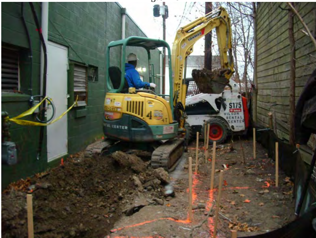
Excavating East to West
