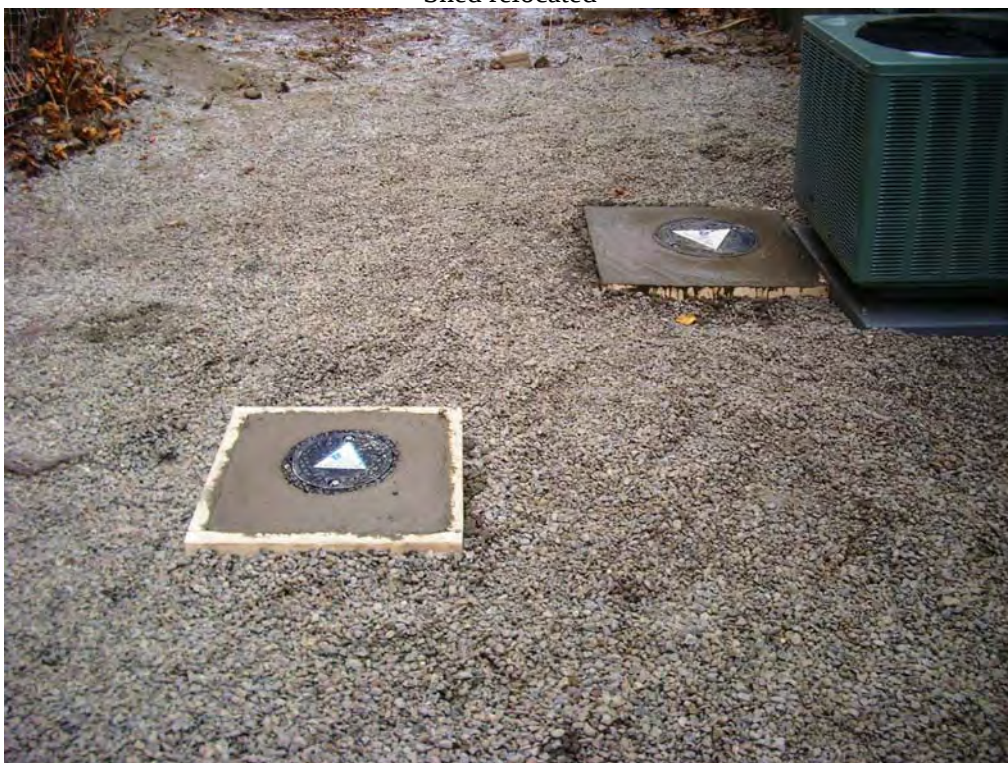
Road boxes (forms still present)
