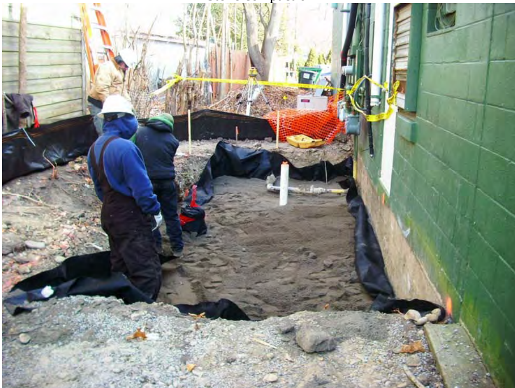
Sand installation (sand layer placed on geotextile)
