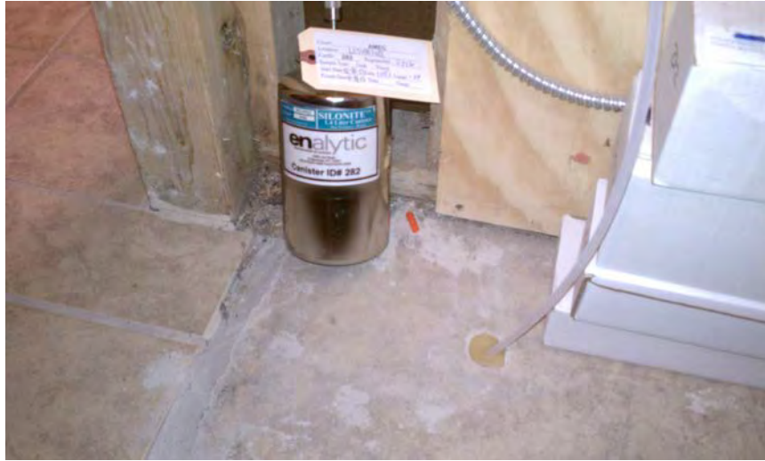
Sub-Slab Soil Vapor Sample Location at Structure 3
