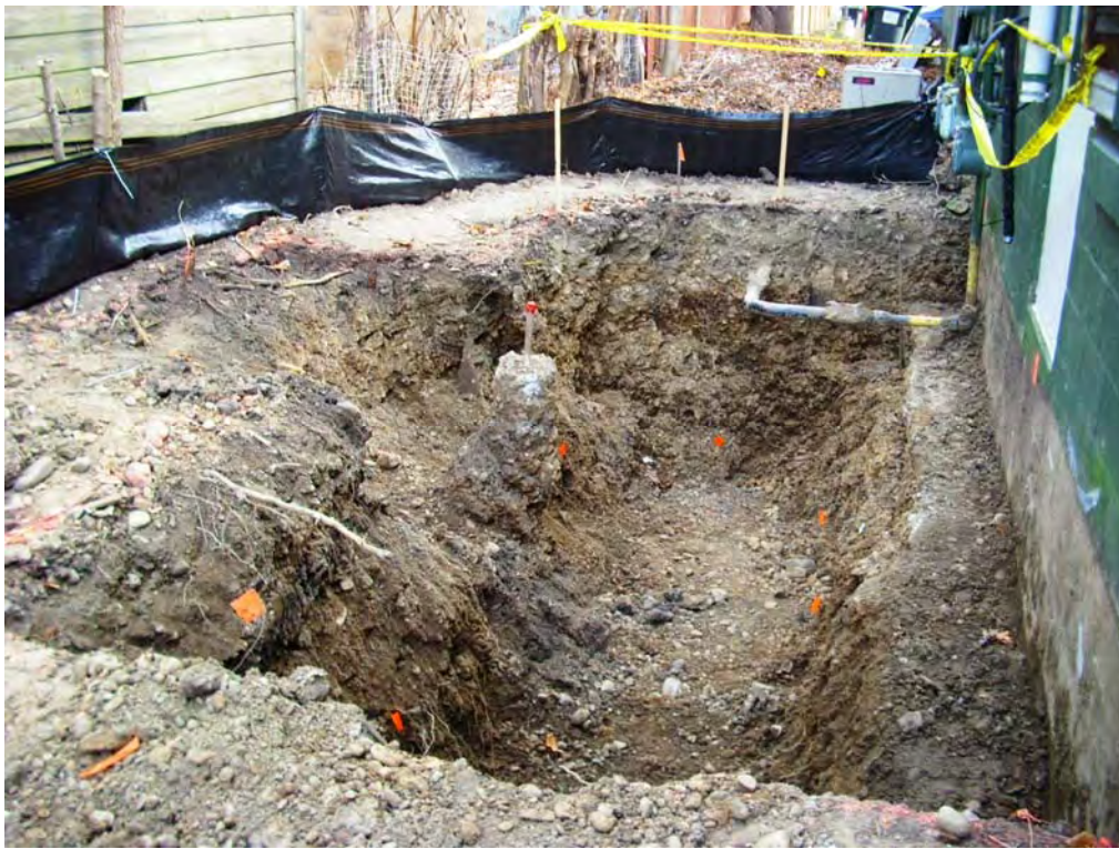
View towards East end of excavation
