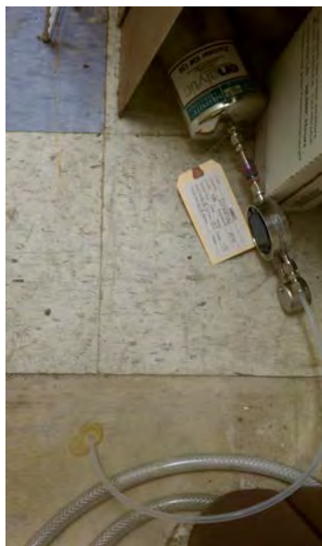
Sub-Slab Soil Vapor Sample Location at Structure 5.
