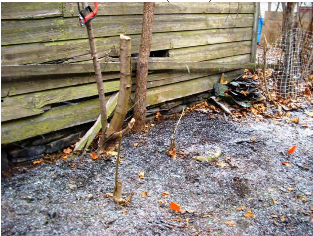
Barn foundation (SE corner)
