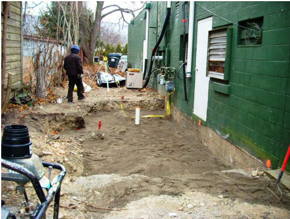
Top sand layer placed on liner
