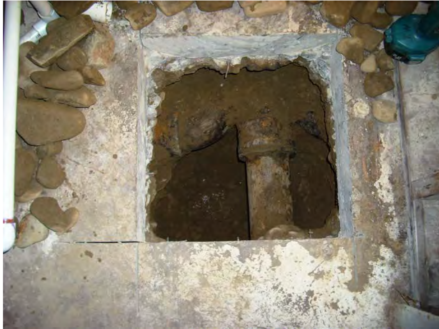
SVE Floor Cut Opening
