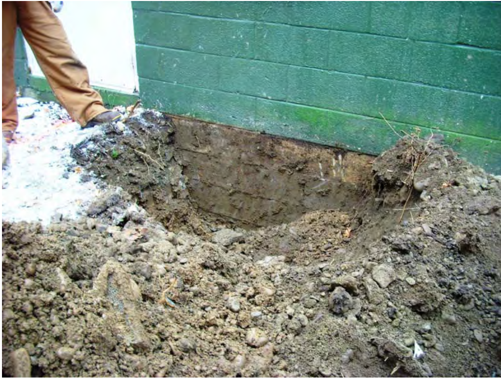
Hand digging for gas line
