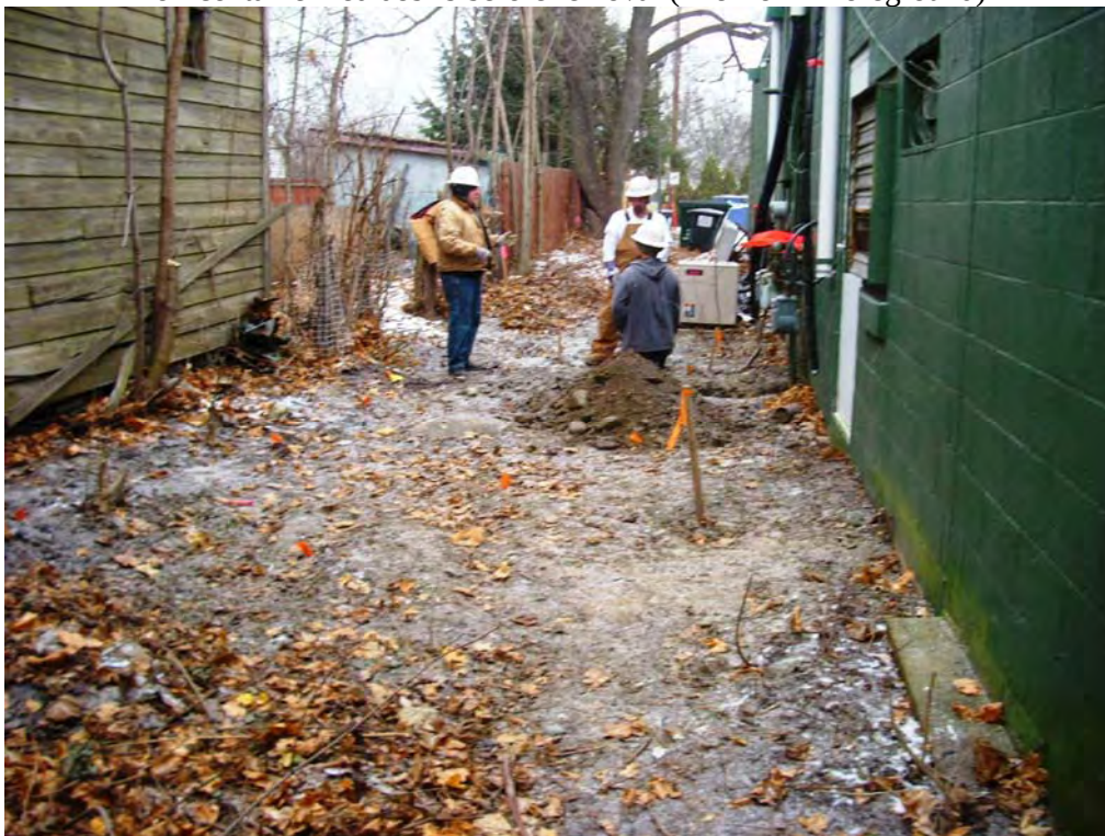
Hand digging for gas line (view towards east)
