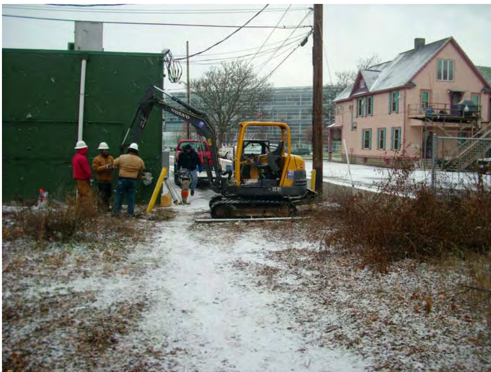
Bucking post removal (at NW corner of Site structure)
