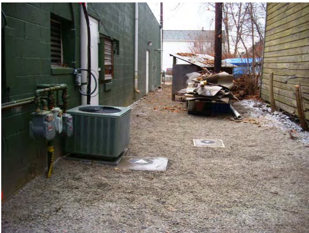
Final grade stone (before trash removal)
