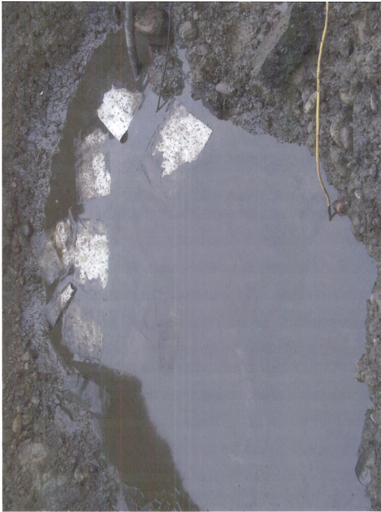
#4: Sorbent pads on residual spill
