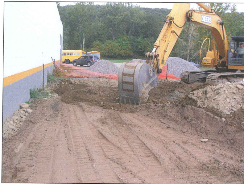
Picture 6 – UST excavation backfill.
