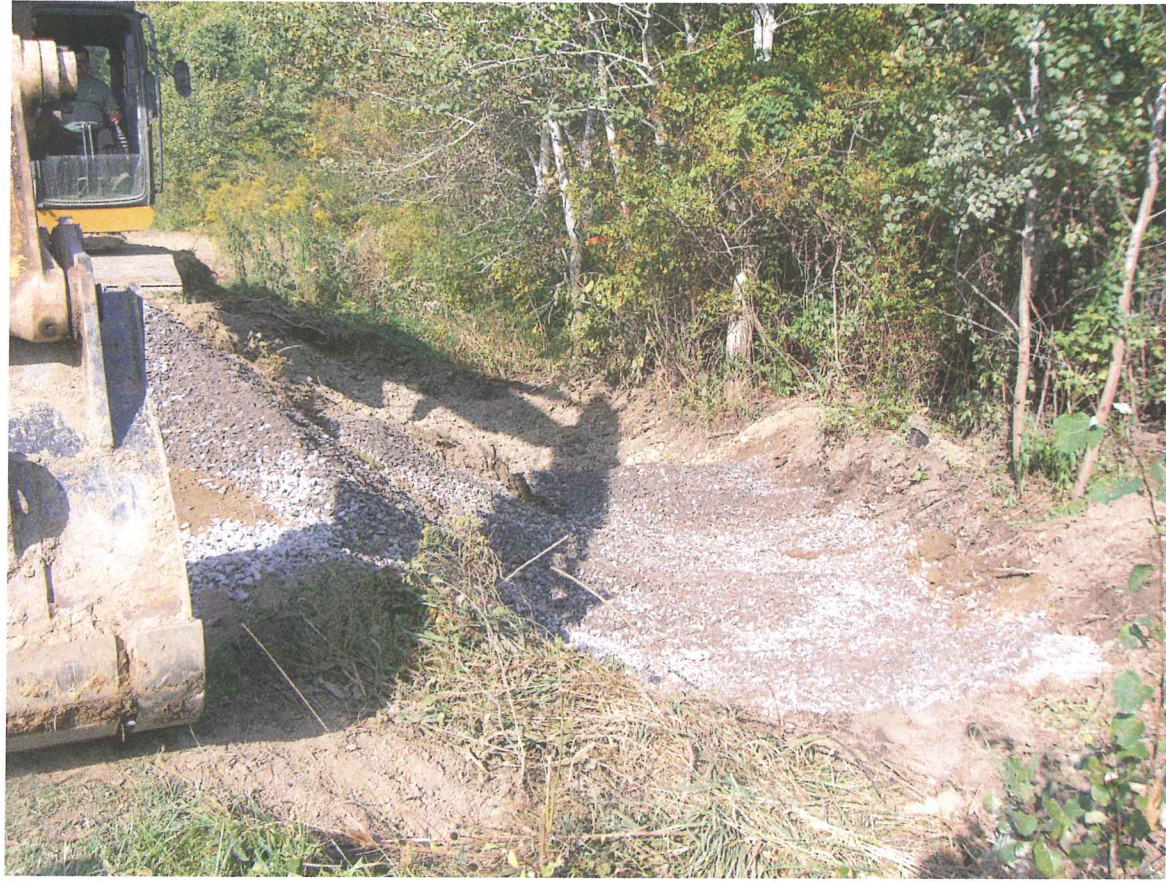
Picture 3 – Drainage ditch excavation backfill with imported fill.
