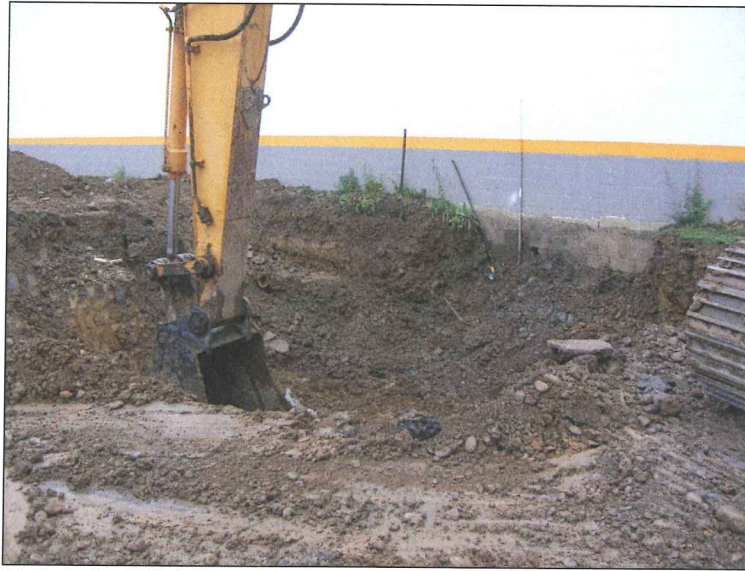
Picture 2 – UST excavation in progress
