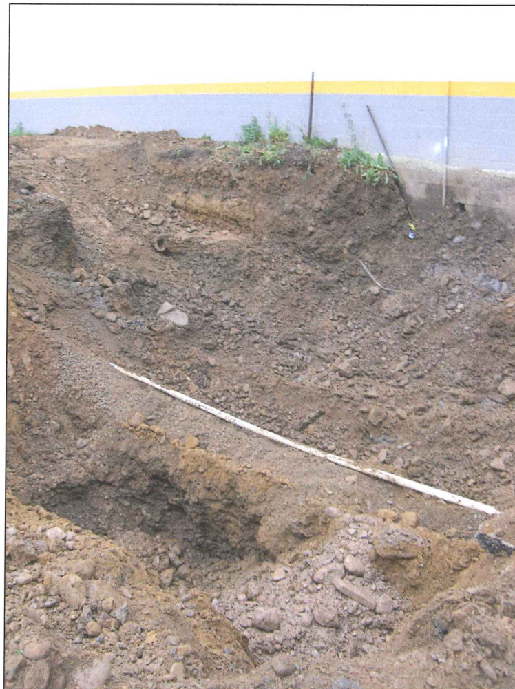
Picture 4 – UST excavation with sewer force main supported by mounded soil.
