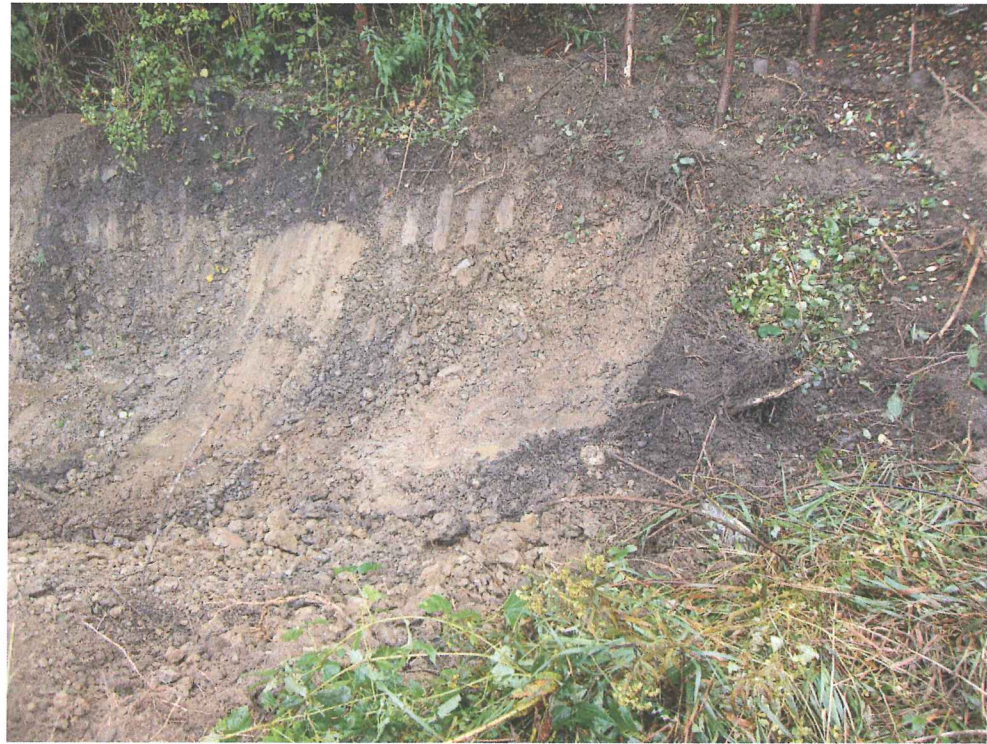
Picture 1 – Drainage ditch excavation
