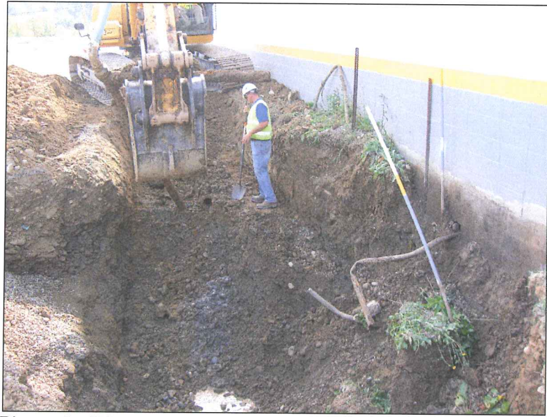
Picture 5 – UST excavation, removing section of separator effluent line
