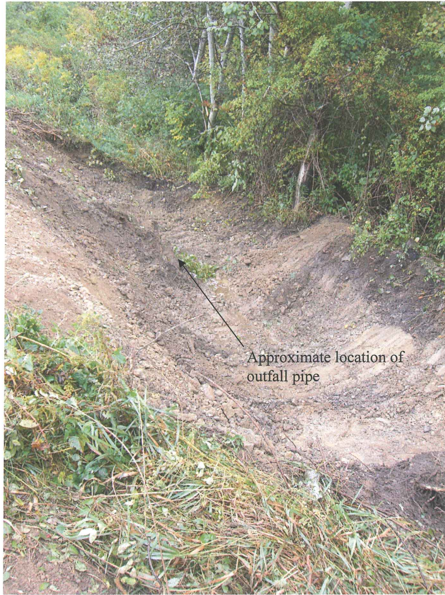
Picture 2 – Completed drainage ditch excavation
