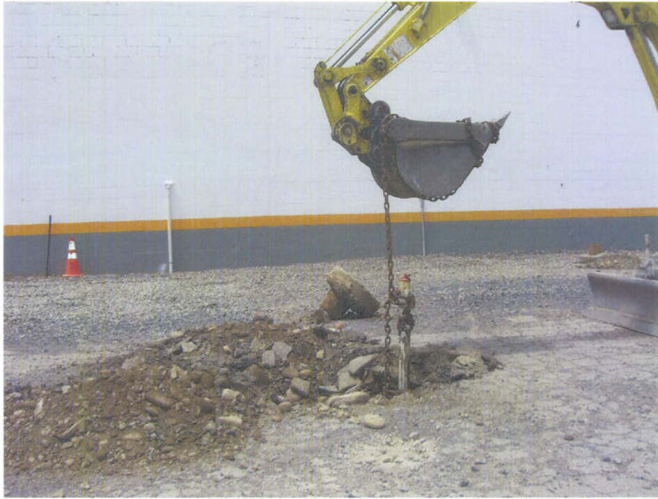
Picture 3 – Pulling MW-2 off of the bottom of the well boring.
