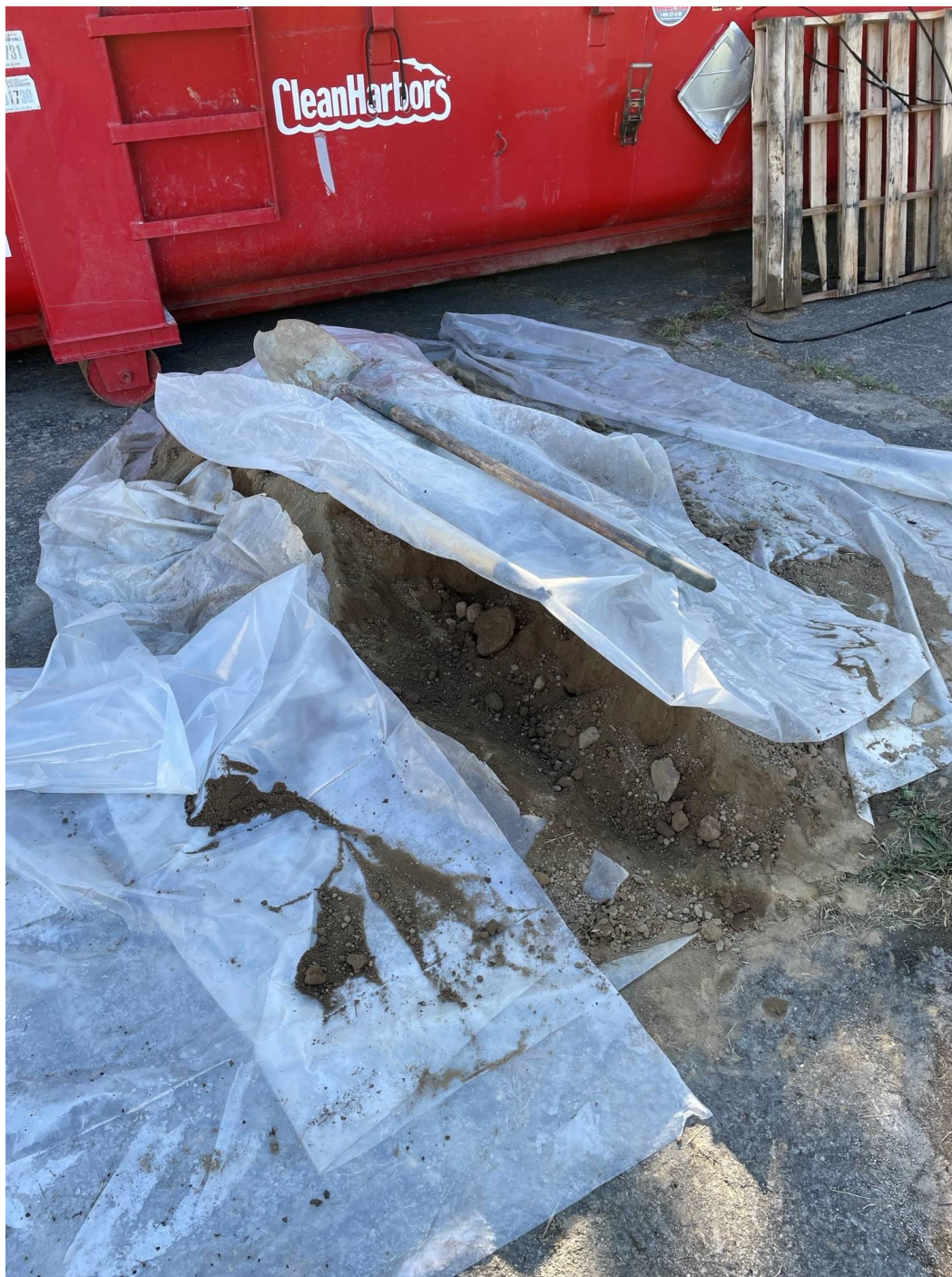
Clean topsoil from clearing borings to 5 feet
