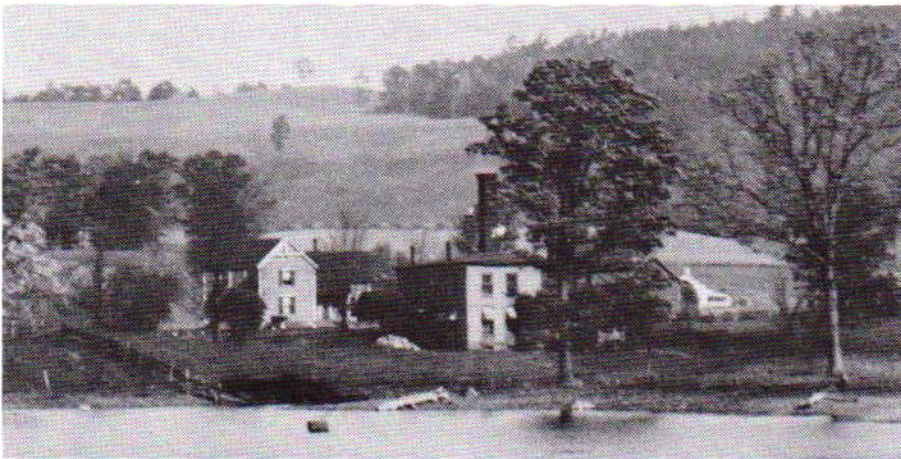
The Bath Water Works, located at the site of the former Cook's Pond.
