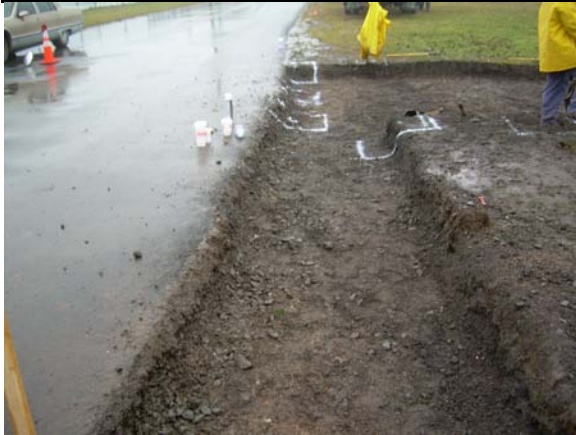
Picture 1: Sidewalk excavation and bollard layout
